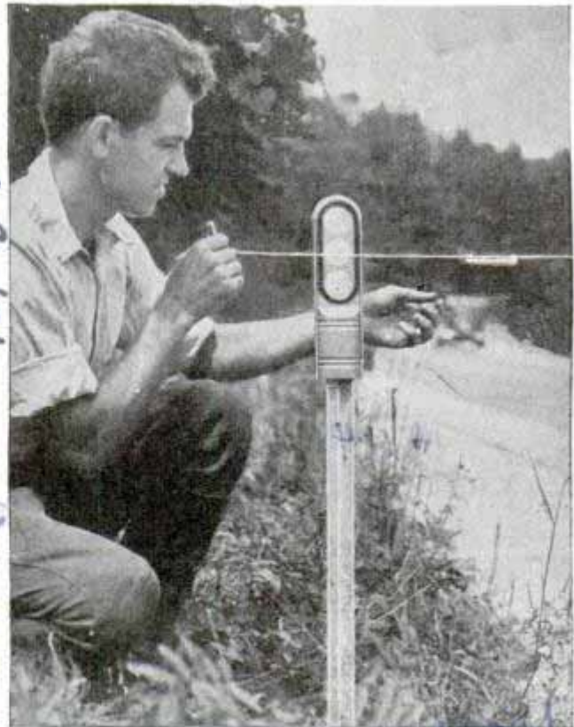
An engineer of the U. S. Bureau of Public Roads adjusts a "cat eye" on roadside post in Maryland.
