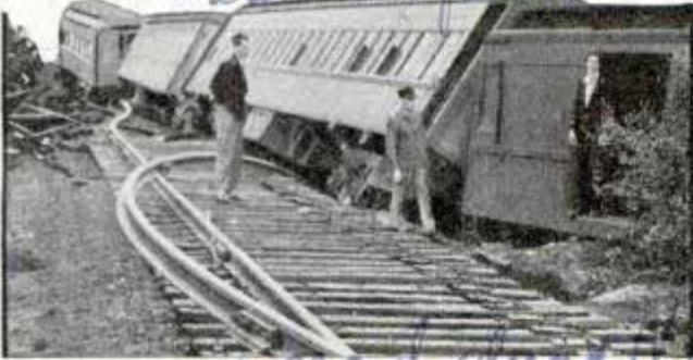
Train derailed by recent hurricane. Note rail twisted from its ties
