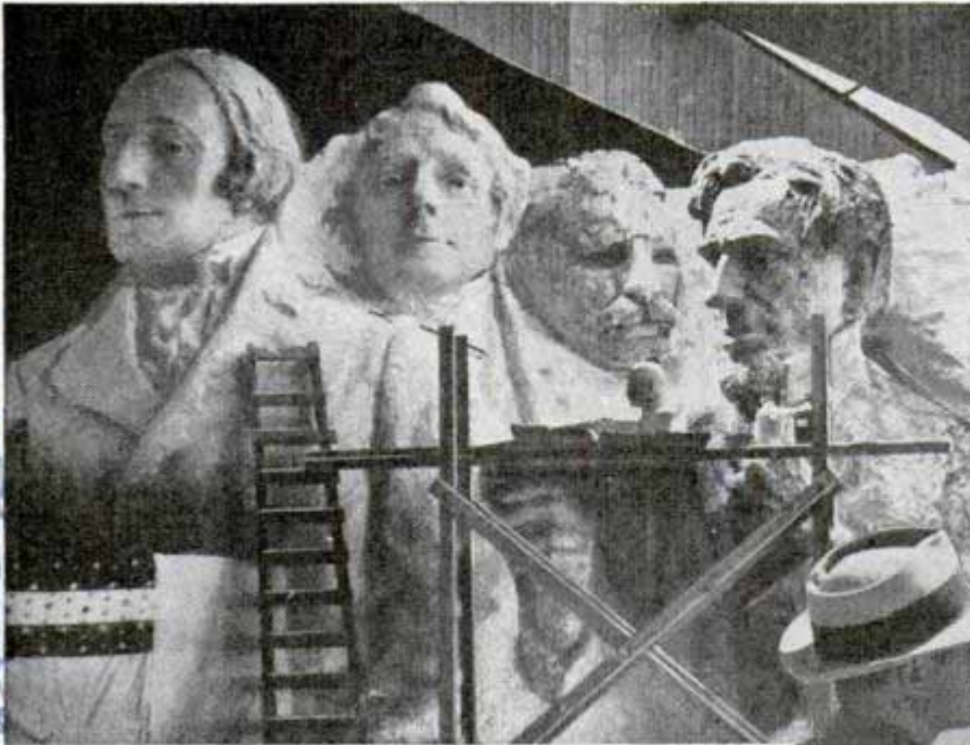
Huge models in studio are used in carving giant faces on Mt. Rushmore in South Dakota's Black Hills. One inch on the models represents one foot on the mountainside. The models aid in making measurements and taking readings
