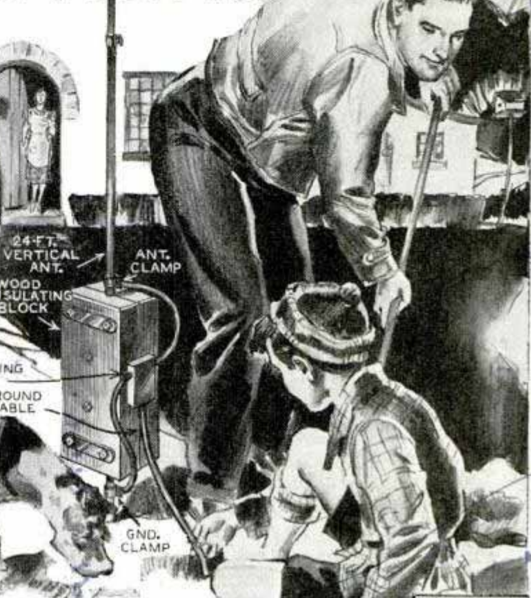
Left, compact antenna-receiver connector now available for running antenna and ground leads through building walls to inside plug and socket arrangement
