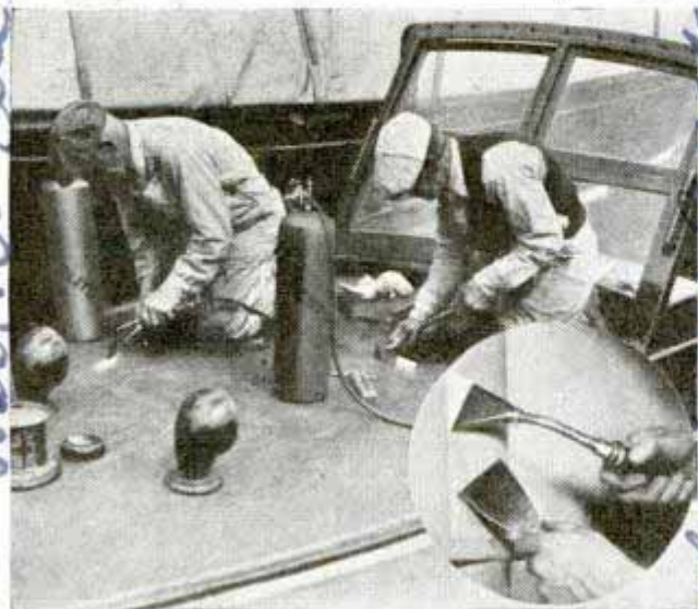
Using acetylene torch to burn paint off boat. Inset, working on curved surface
