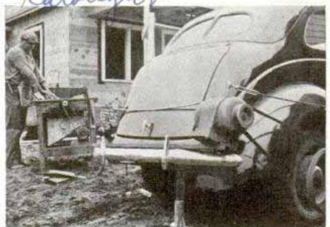
Wheel of car jacked up to operate generator that powers stationary machinery
