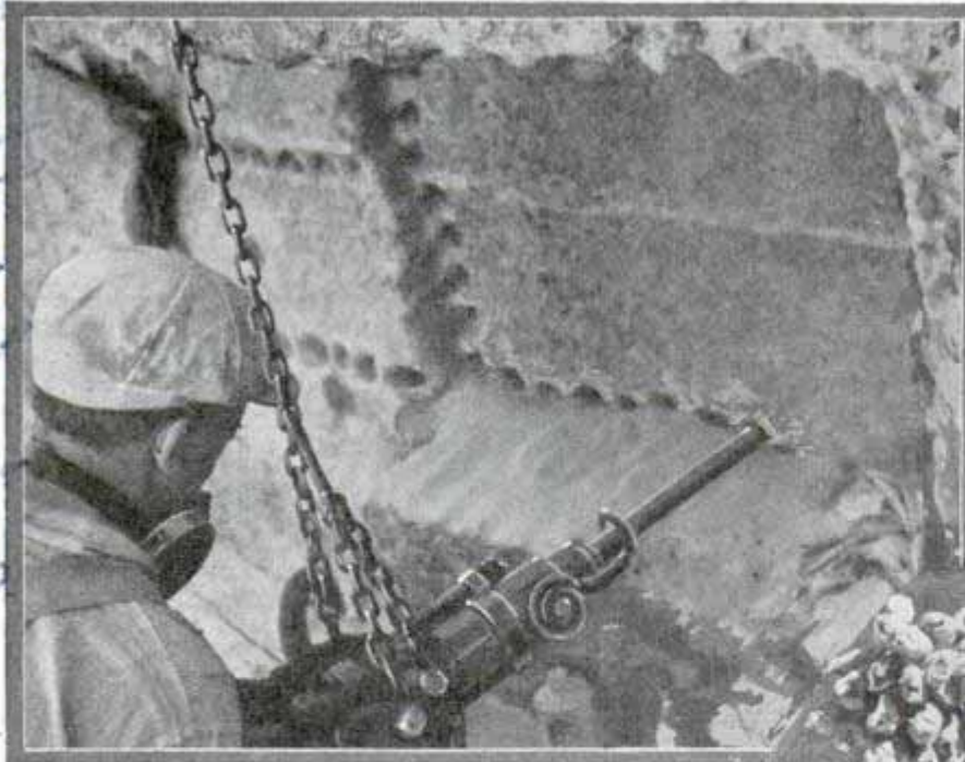
Above, jackhammer driller prepares holes for dynamite in the granite. Blasting then loosens the rock. Right, Lincoln Borglum, son of the Mt. Rushmore sculptor, Gutzon Borglum, holding bundle of small dynamite charges and a bundle of caps and fuses used in blasting
