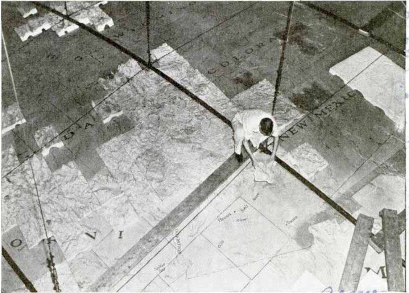
Mapmaker finds a place for a tiny segment of United States in the huge relief map, so accurately made that it conforms to curvature of earth's surface. It is built on steel frame sixty-three by forty-five feet
