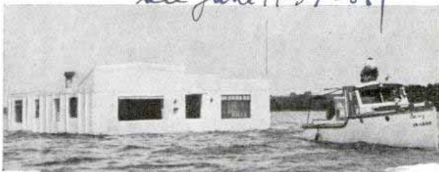
Nothing but its own buoyancy supported this forty-one ton all-steel house as it floated across the Illinois river in tow of a motorboat
