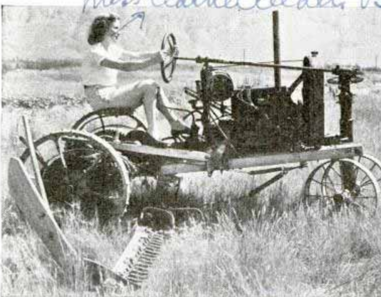
Grain mower built of odd parts is driven by automobile engine
