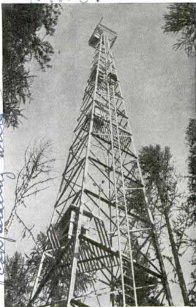
Weather instruments are stationed at five stages of this 150-foot tower to study "fire weather"
