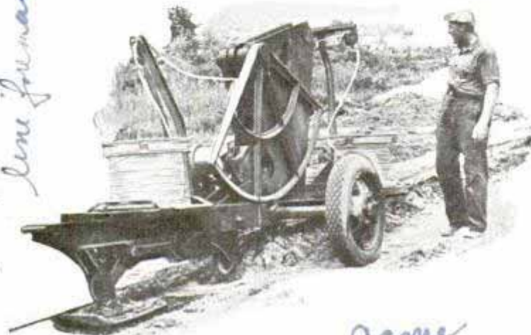
Telephone wire is fed into the ground from these spools as the plow turns up a furrow twenty-four inches deep
