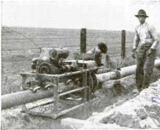
Pipe-coating machine traveling along the line, applying cement material
