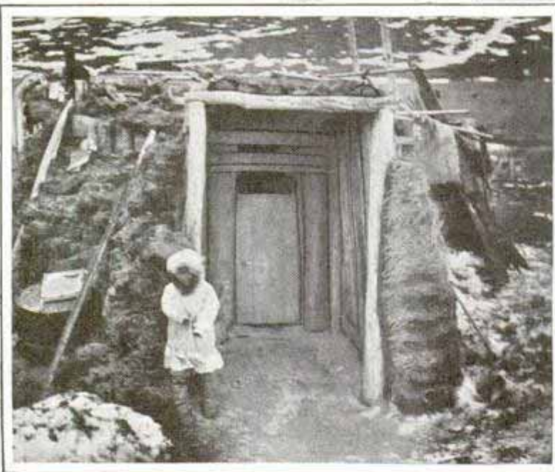
Top, sketches of the skin boat of the Eskimo and of the entrance to the igloo. On opposite page is the igloo, with its air-conditioning arrangement. Bottom, this page, vestibule to entrance tunnel of igloo. Note sod and driftwood construction. The little girl wears parka, with fur garments beneath
