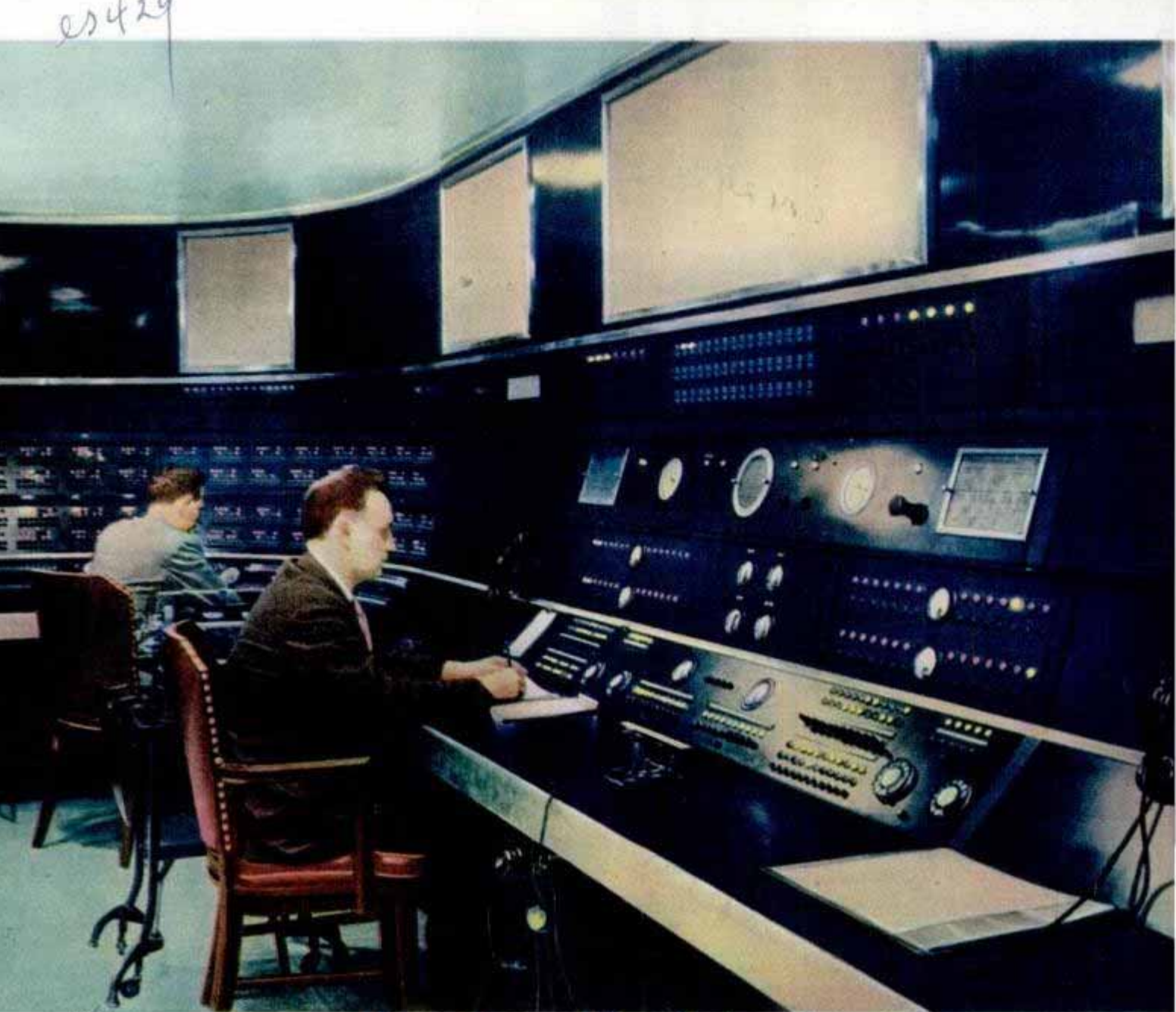
656 MAIN control board of a great broadcasting system. Here the ether jumpers are tuned in with events happening all over the world.
