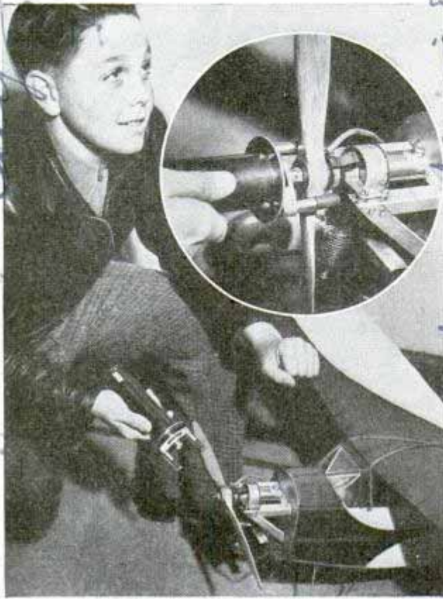
Coil spring inside "flashlight" case twirls prongs and "winds up" motor of model airplane
