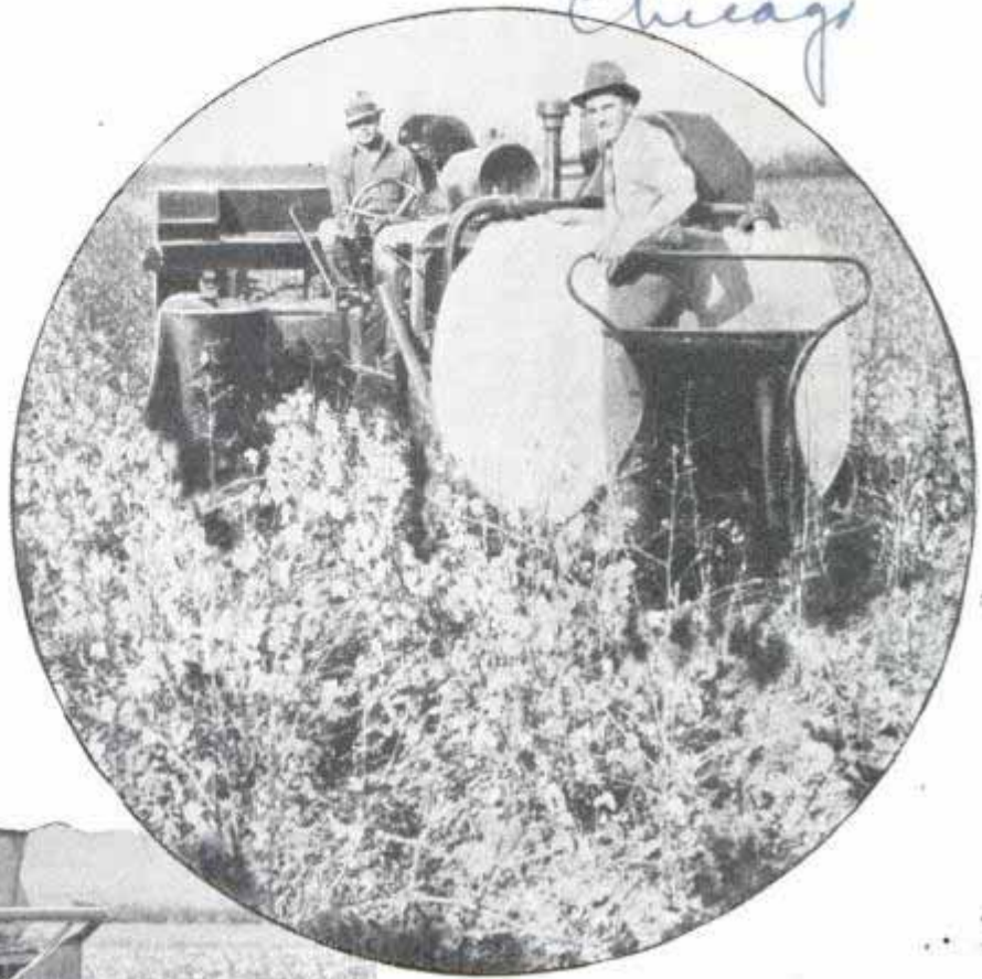
Picker at top deposits cotton in bags; left, basket collects cotton from conveyor. Below, another view of spindle-type harvester attached to standard farm tractor
