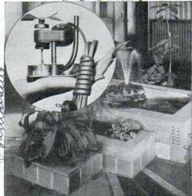
Inset, tiny pump rests in palm of hand. Below, fountain operated by midget pump
