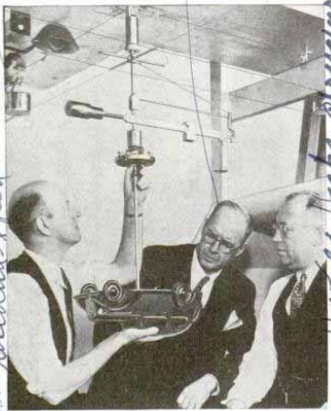
Scale model of car is suspended upside down in wind tunnel to test operating efficiency of body lines
