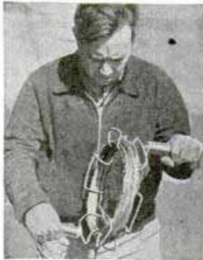
Wire reels you can make for winding rope and wire around the home
