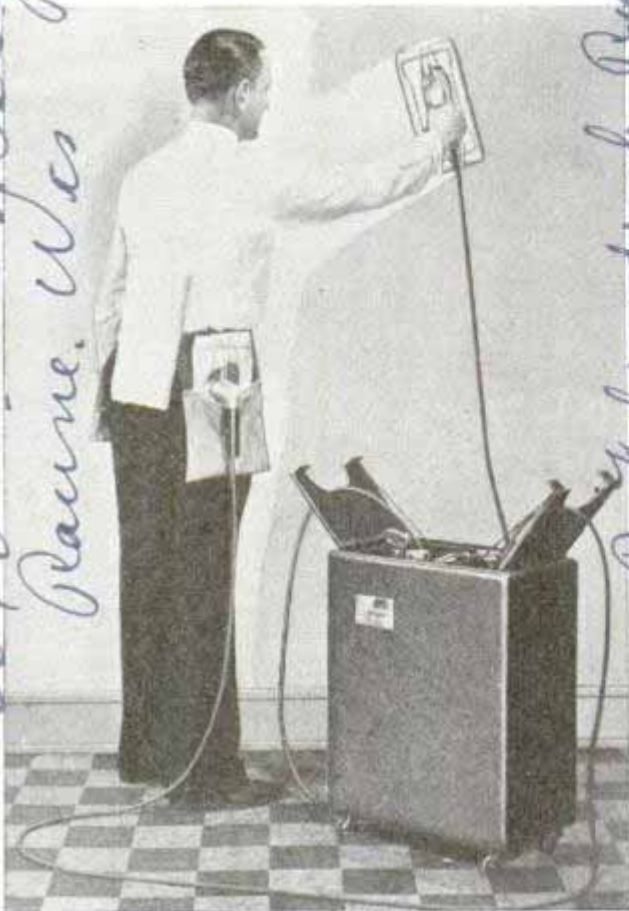
Cleaning walls with aid of machine which closely resembles modern radio receiver
