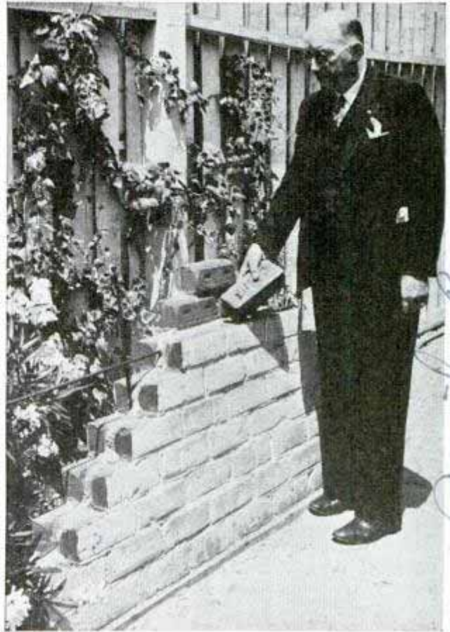
Garden wall being constructed with rounded-corner brick. Note reinforcing bars
