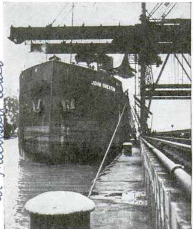
Unloading iron ore with the aid of clamshell unloaders such as the one shown at top of page
