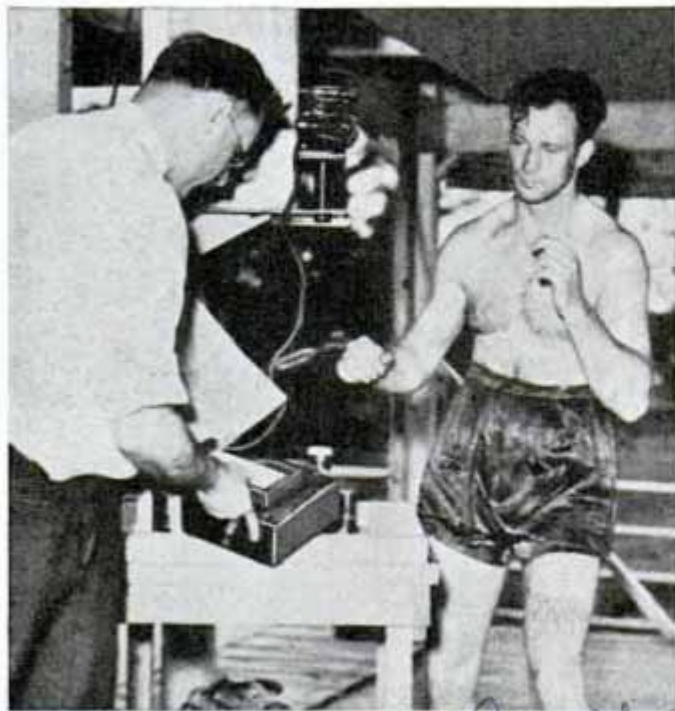
Professional boxer's fist travels past photocells at forty miles an hour; amateur's best was twenty
