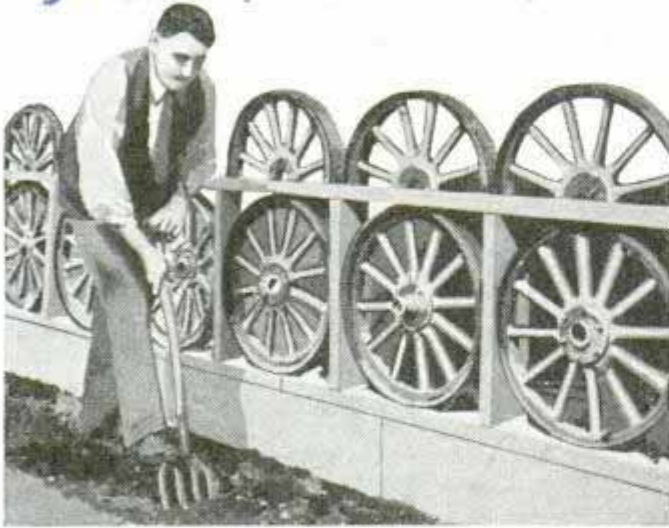
This garden fence at the rear of a San Antonio home is made of wooden-spoke wheels from early autos
