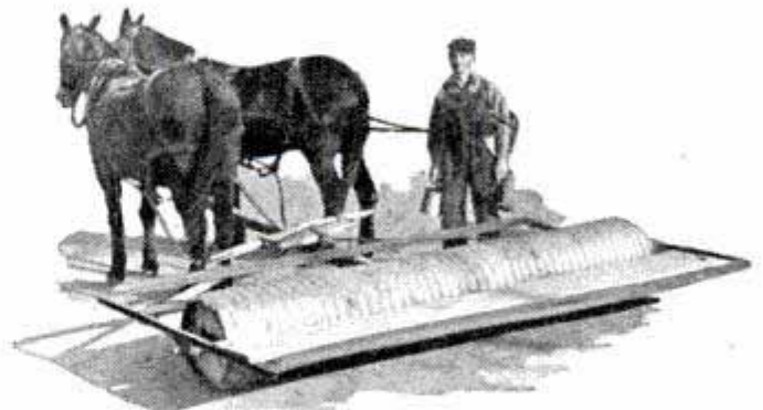
Corrugated steel culvert filled with concrete and provided with axle makes emergency land roller
