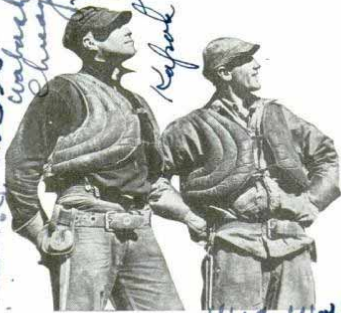
Workers wearing safety vests which support them if they fall from dam into river
