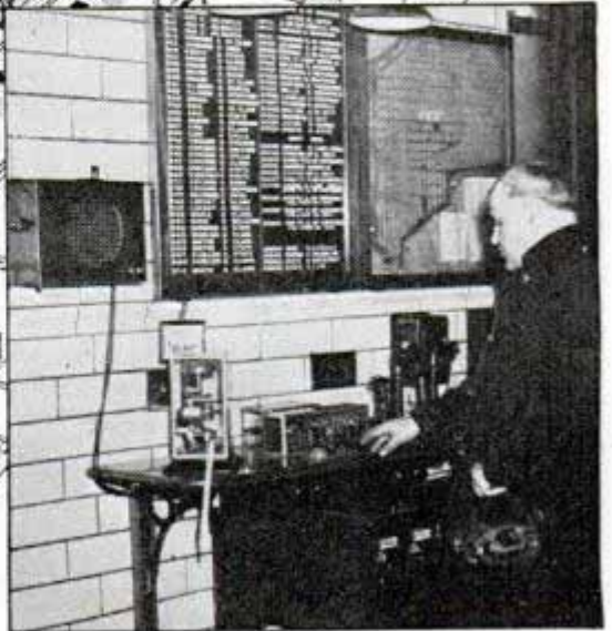
Seconds count in fighting fires, and loudspeakers are cutting twelve to twenty seconds from response time of city fire squads. Still alarm reaching central office, top, is dispatched to speaker in every station
