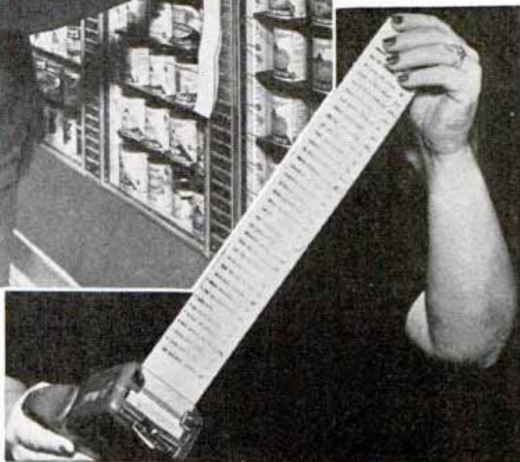
Pressing arm of magazine into various slots, as at left, customer obtains printed shopping list, below. Cashier totals bill and clerk fills order
