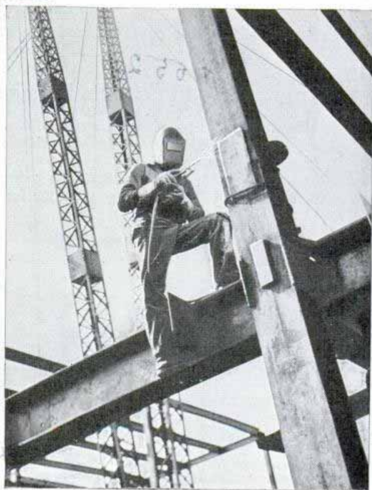
Left, welder at work. Special glass in helmet enables him to see through arc glare. Right, welding frame of industrial building
