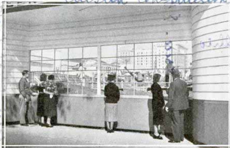
Passersby are shown watching construction crew, safe behind the window built into fence around the building project
