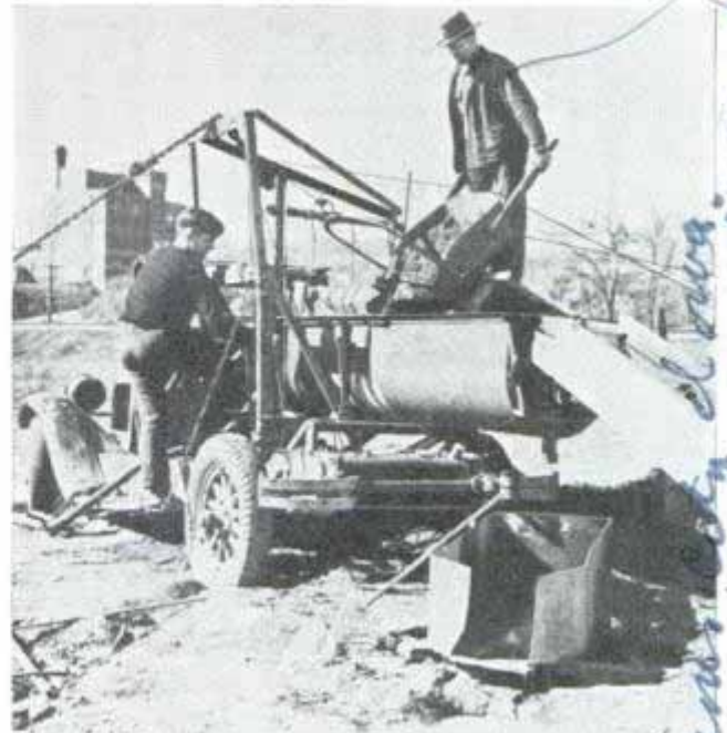
above Dumping scrapings from target range into machine which recovers the lead bullets
