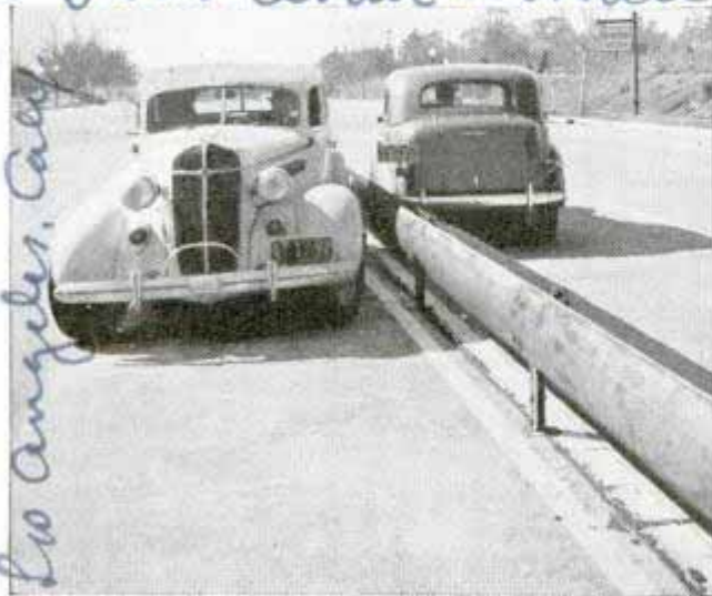
Kept from colliding head-on at center of the highway, two cars carom off from convex steel guard rail
