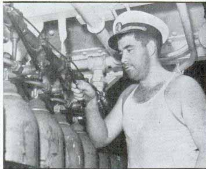
Above, operating valve which closes all watertight doors at once. Bottom, left, checking lubrication of bearings. Right, inspecting part of ship's fire-fighting equipment
