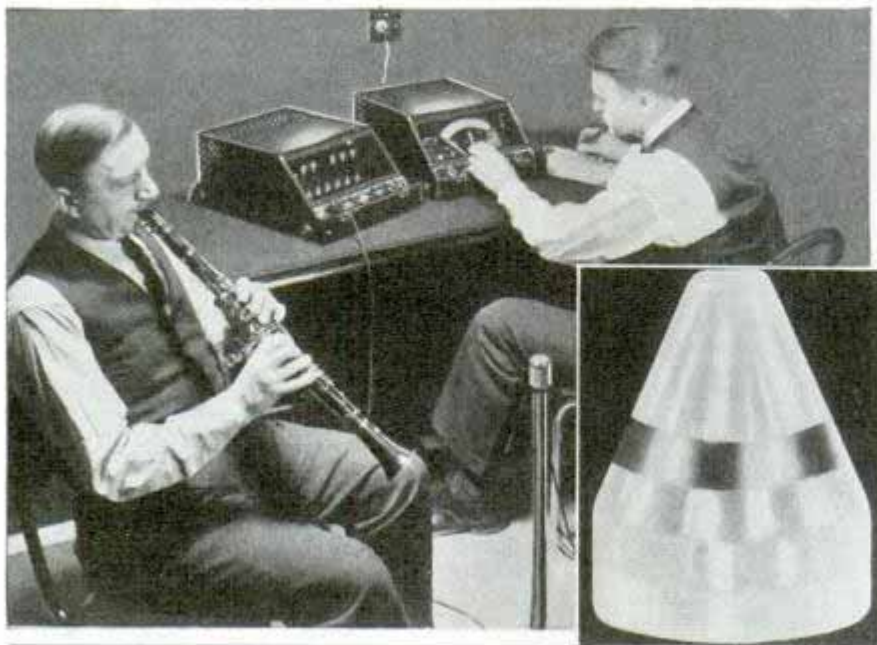
Testing tone of a wood-wind instrument with chromatic stroboscope. Inset shows pattern of one of the lighted windows seen in unit at left
