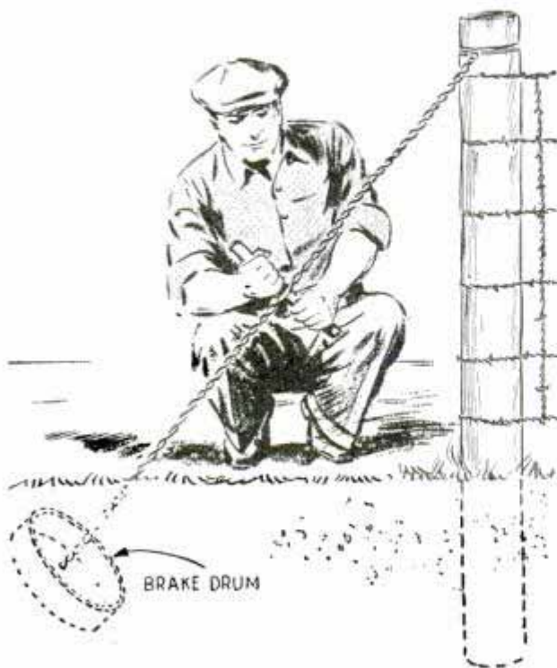
Brake drums provide good anchors for fence-post brace wires as they do not pull out of the ground
