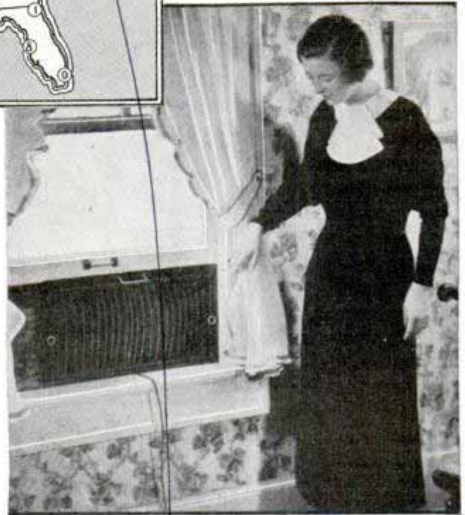
Top, ragweed pollen map, with points free from the pollen being marked zero. Bottom, room air filter for removing pollen from the air
