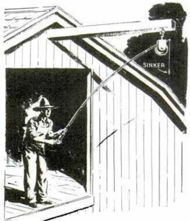
Push end of rod through pulley, unreel line to the ground and tie rope end to it and reel in the line
