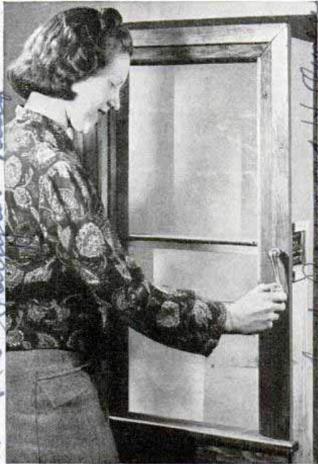
Turning crank to lift or lower either pane of window. It locks in position when crank is released
