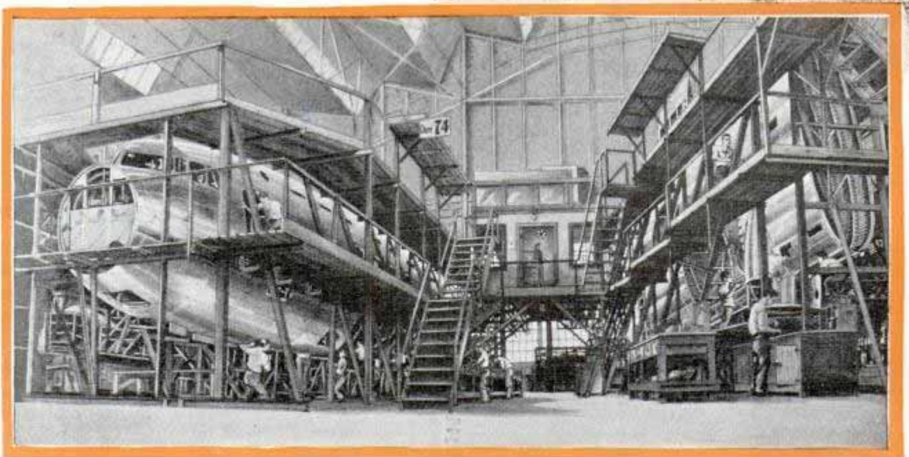
Bottom, view of workmen busy on giant fuselage and wings of Douglas transport, DC-4. The scaffolding forms a sort of dry dock in which the plane was assembled like a ship
