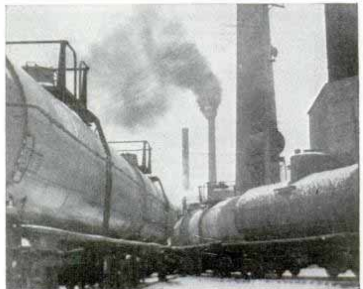
Part of fleet of anhydrous ammonia and alcohol tank cars at du Pont plant at Belle, W. Va.
