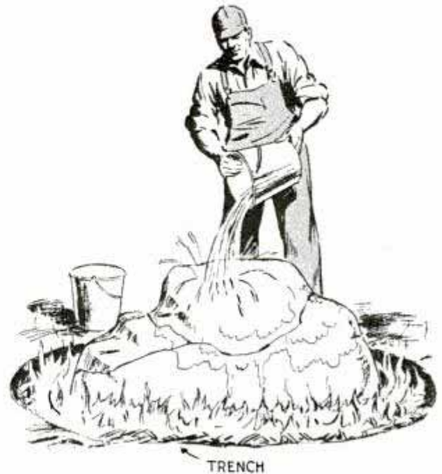
Large stone broken by heating it thoroughly and then throwing cold water over it
