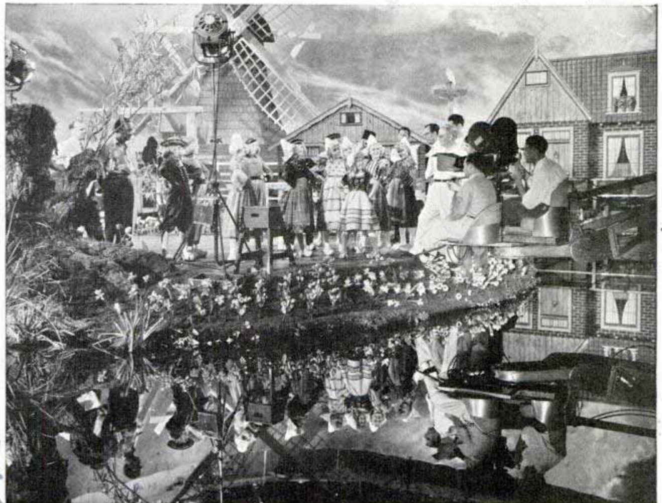
This scene from "Heidi" illustrates the use of oil pools for reflection shots. Note the clarity of the reflection. The camera crew is shown riding a boom over the pool
