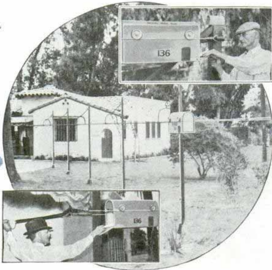
The mailbox of R. H. Bess at Downey, Calif., is really an electric trolley car. In the center it is seen traveling its aerial cable route from roadside terminal (upper right) to bring mail to front door, below
