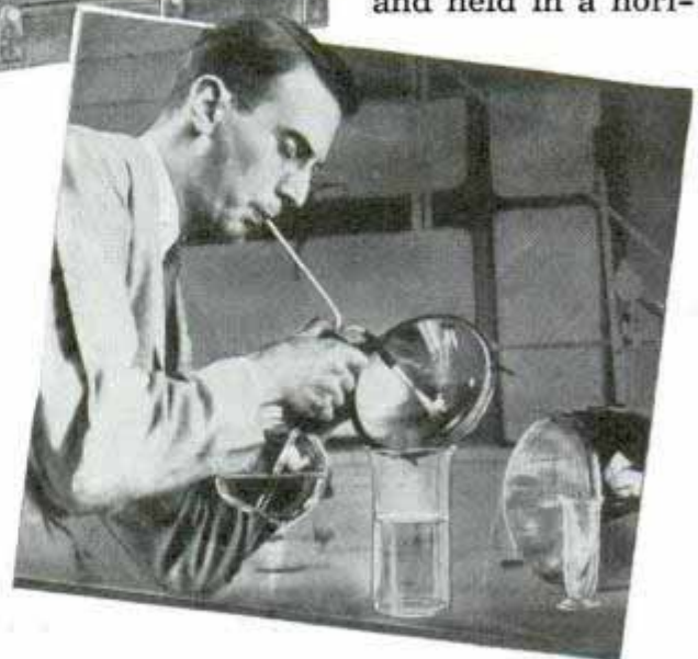
Checking silver surface coating of Plymouth headlamp. Silver is stripped off, precipitated and weighed
