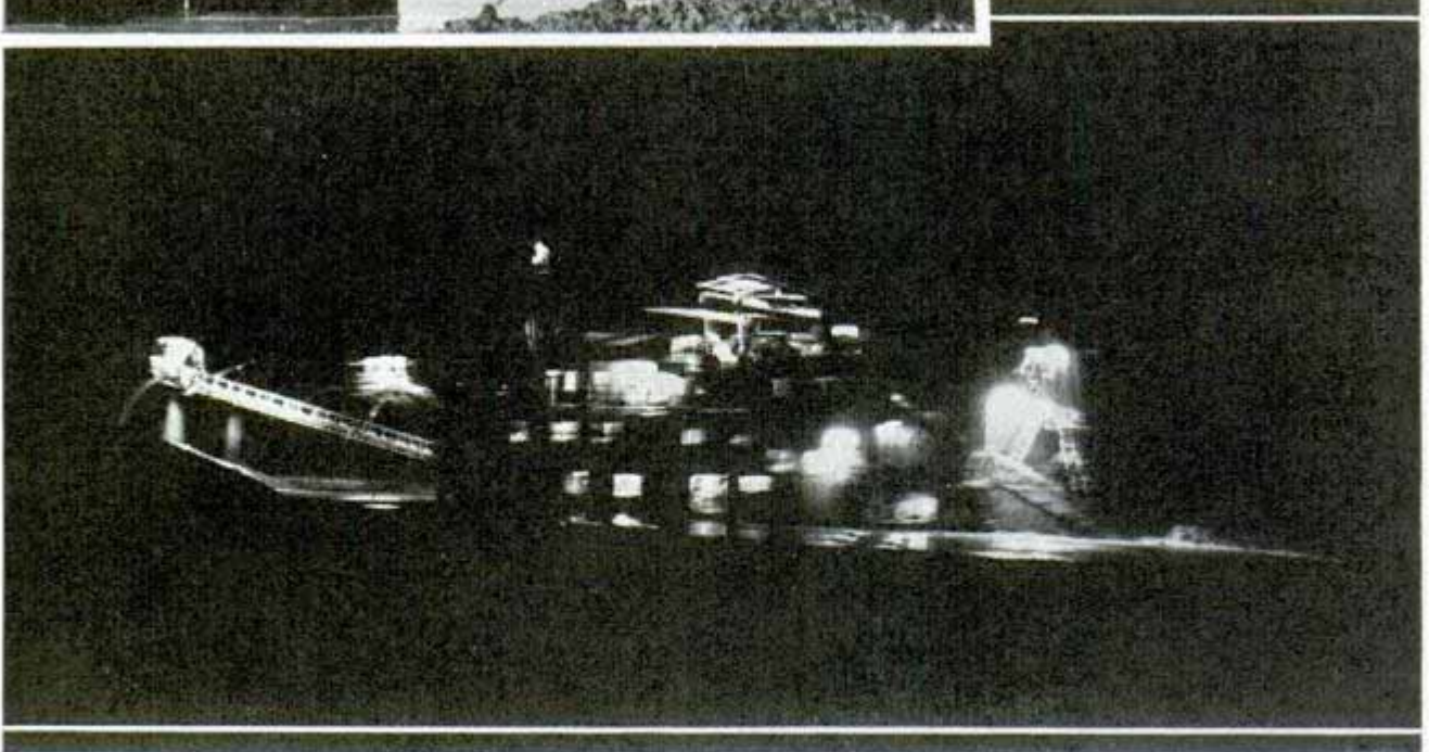
Top, bow gantry of giant gold boat, showing digging ladder raised to start new cut. Bottom, night view of a gold-dredging machine. These big machines weigh 2,200 tons
