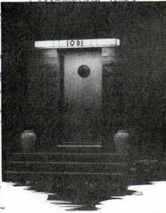
House numbers show up clearly against lighted box made of sheets of a translucent plastic material
