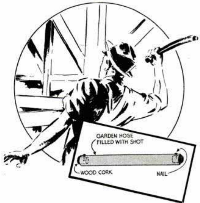
Dismantling a scaffold with a "loaded" rubber hose which distributes the blow and avoids splitting
