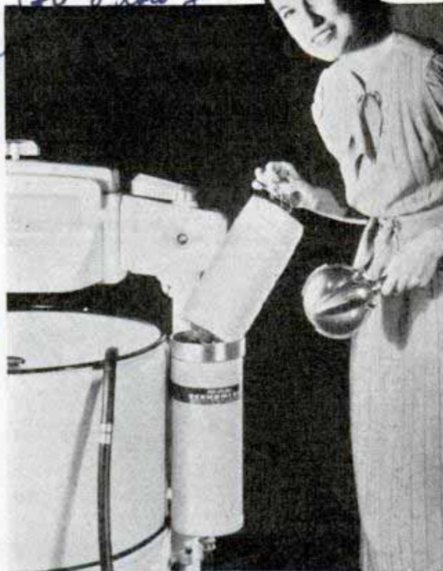
Inserting fresh cartridge in the water softener which treats water as fast as it flows into washer
