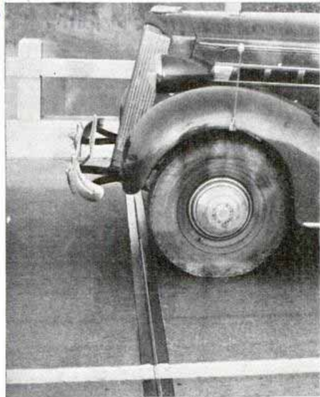
Showing automobile about to pass over expansion joint that makes riding easy
