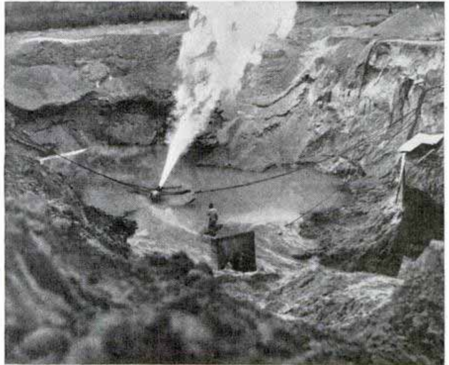
Earth slide on far side of crater helped smother flames of this oil well. Observe the pressure in the jet of burning gas escaping from casing
