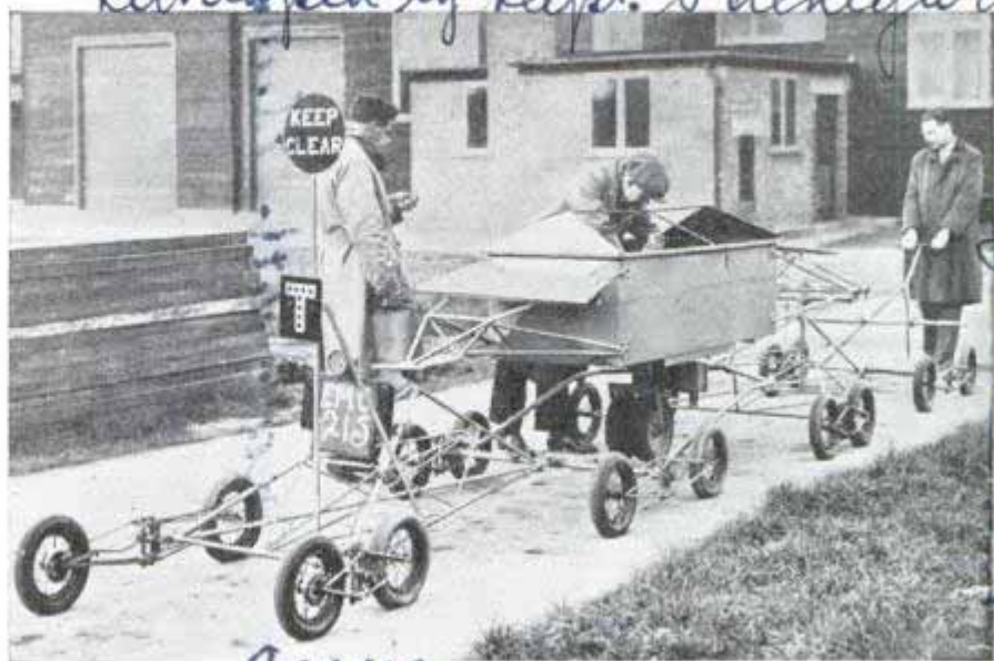
While one man propels this multi-wheeled road tester, another keeps watch on graph where irregularities in pavement are recorded
