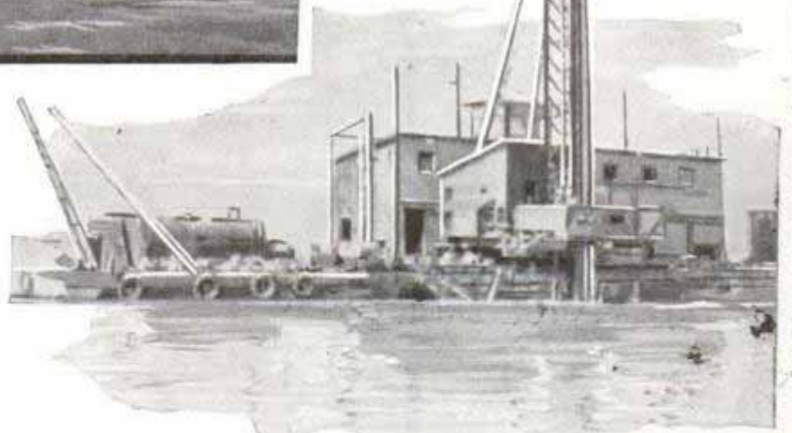
Top, explosive hurls water and rock into air. Right, preparing dynamite charge. Bottom, a drill boat in action. Note the eighty-foot tower supporting the hammer
