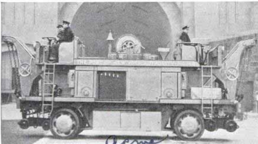
Ready for wreck or rescue in New York's Lincoln Tunnel is this gasoline-electric emergency truck which can be driven and steered from either end
