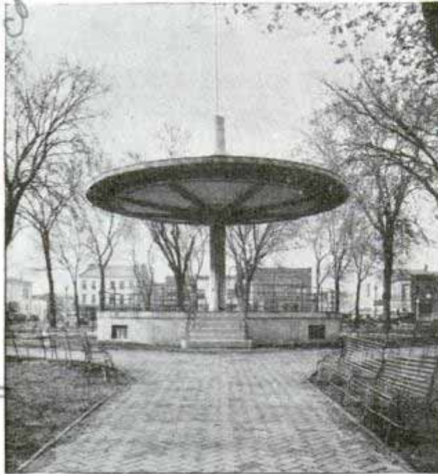
Umbrella-shaped roof of bandstand acts as megaphone while loudspeaker in pinnacle broadcasts sound
