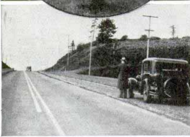
Drivers in state of Washington are warned of blind spot ahead by white line painted in opposite lane
