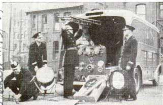
This English fire truck carries electric tools, loudspeaker and equipment for resuscitating victims
