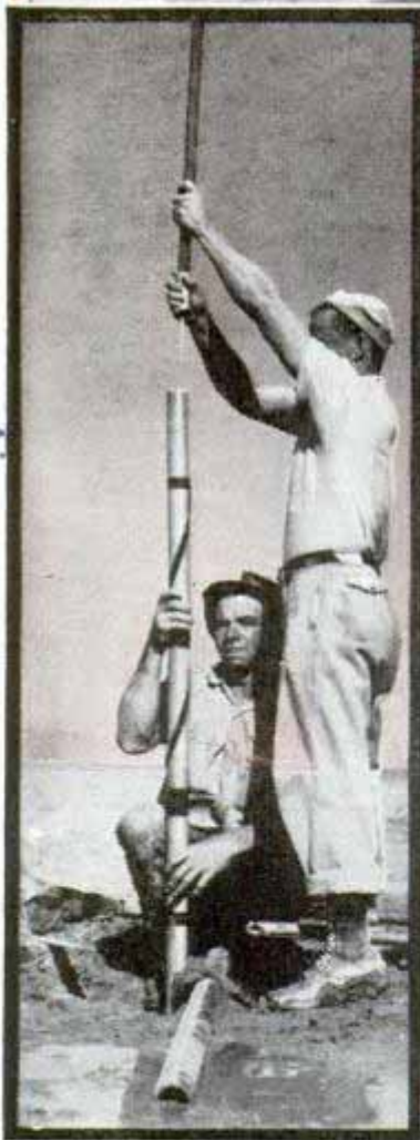
Top, interior of laboratory truck where seismic records are drawn on paper cylinder. Bottom, preparing to drive dynamite charge into hole. Drawing at right shows typical cross section of earth's crust
