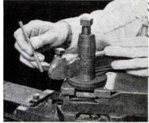
You can give lathe tool bits that extra keen, extra smooth edge by touching them up with an Aloxite Brand Abrasive Stick.
