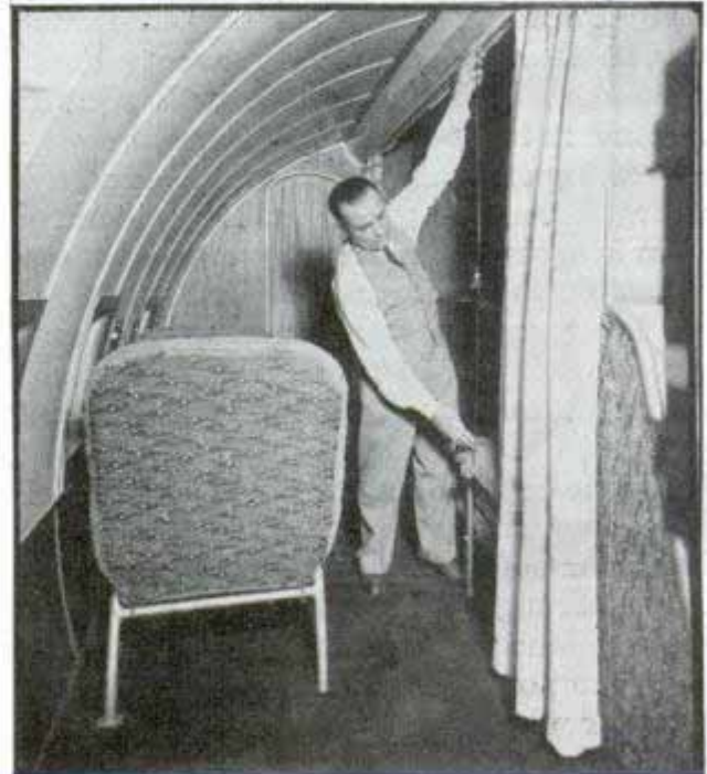
Top, passenger compartment, as seen from center aisle. Center, one of the giant engines installed in a wood and metal mock-up of nacelle. Bottom, engineer checking size of berth compartment
