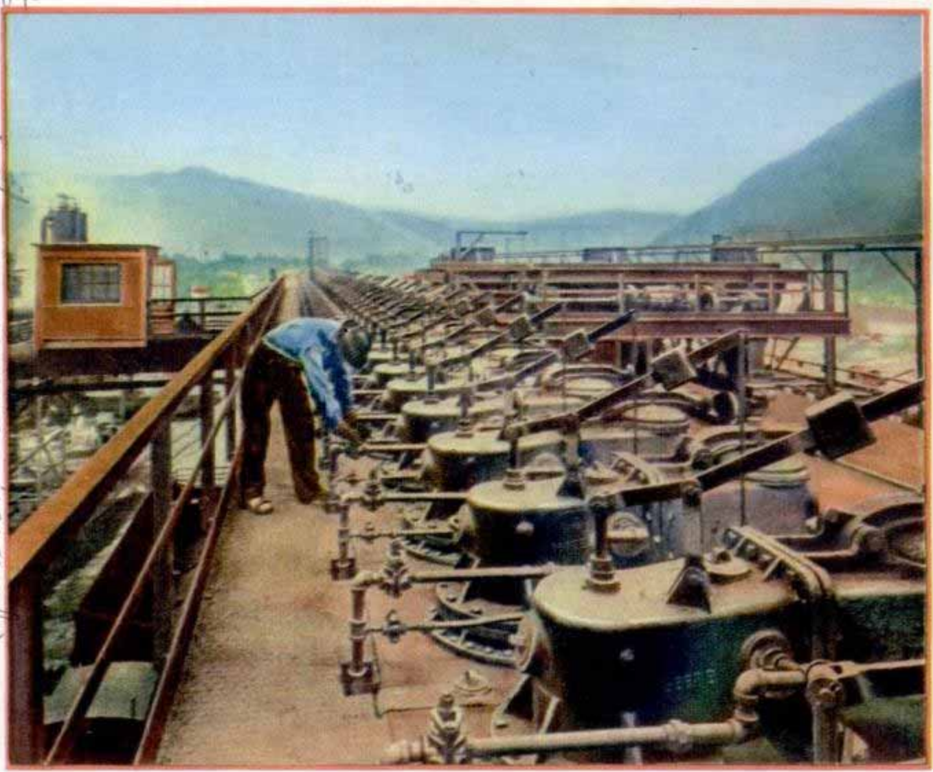
CHEMISTRY on a huge scale. At top of a coke-oven battery, the coal is charged into ovens and volatile matter is distilled off, leaving coke used in making "blue" water gas.
