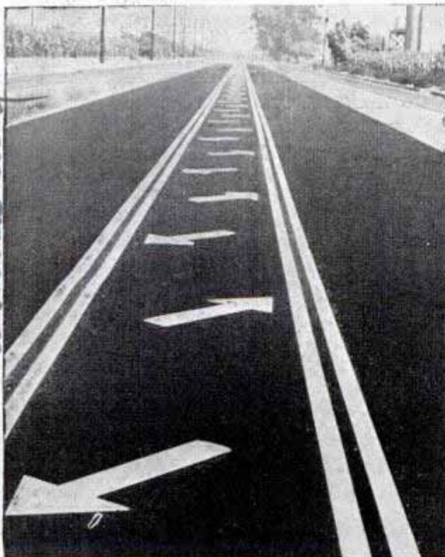
White pointers warn drivers to stay in their lanes, and are raised enough to make safety lane bumpy
