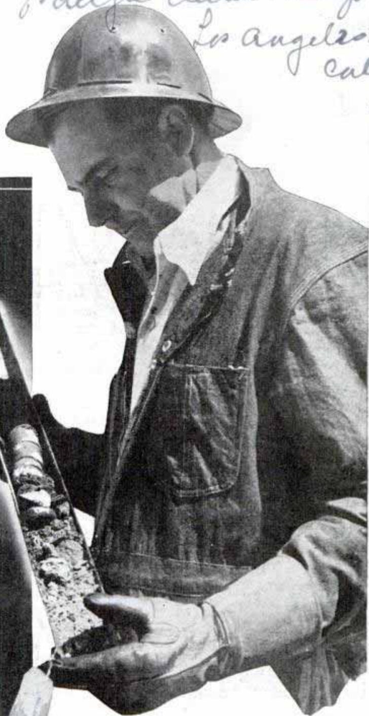
Left, night drilling scene. Right, samples of rock cut from bottom of well and brought to surface by coring machine that drops down inside drill pipe
