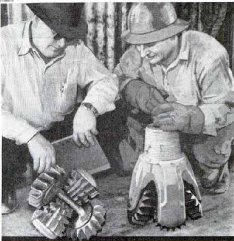
Top, derrickman descends from lofty perch in emergency cage. Left, split section of pipe recovered at great depth by means of wall hook. Bottom, bits used in drilling deep well
