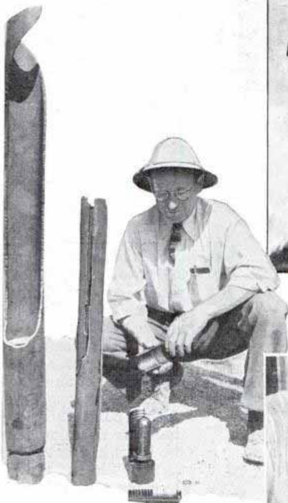
Top, derrickman descends from lofty perch in emergency cage. Left, split section of pipe recovered at great depth by means of wall hook. Bottom, bits used in drilling deep well
