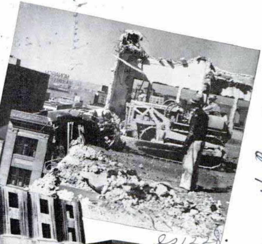
Top, tractor pushing debris over the side. Center, building in process of being wrecked. Bottom, lowering tractor to another floor
