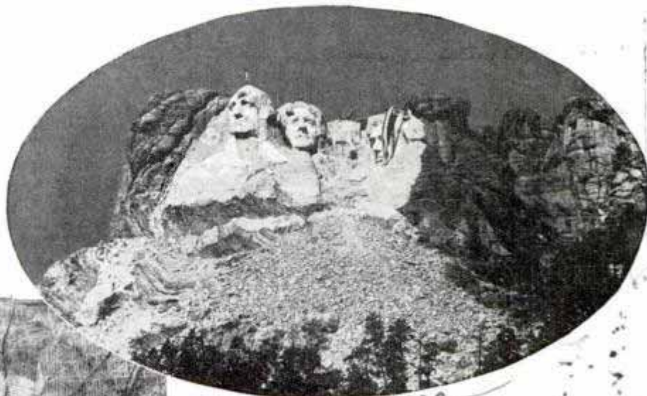
Right, general view of the Mt. Rushmore memorial near Rapid City, S. D. Below, close-up of workmen, under the direction of Gutzon Borglum, carving the head of Abraham Lincoln
