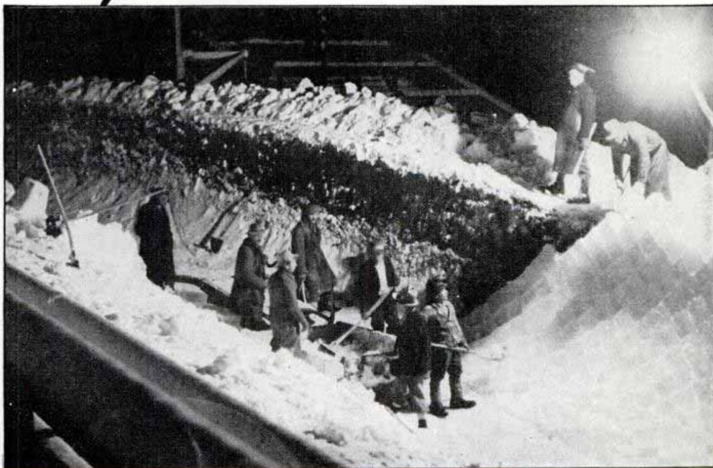
Top, up a wall of ice on a run in Germany. Bottom, building a run by laying ice squares on the turns. Course is watered to freeze the squares uniformly
