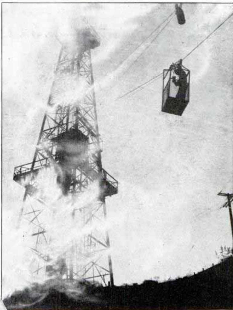
Top, derrickman descends from lofty perch in emergency cage. Left, split section of pipe recovered at great depth by means of wall hook. Bottom, bits used in drilling deep well
