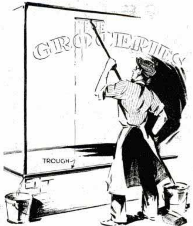
Gutter at bottom of show window drains dirty water into a bucket and keeps it off sidewalk
