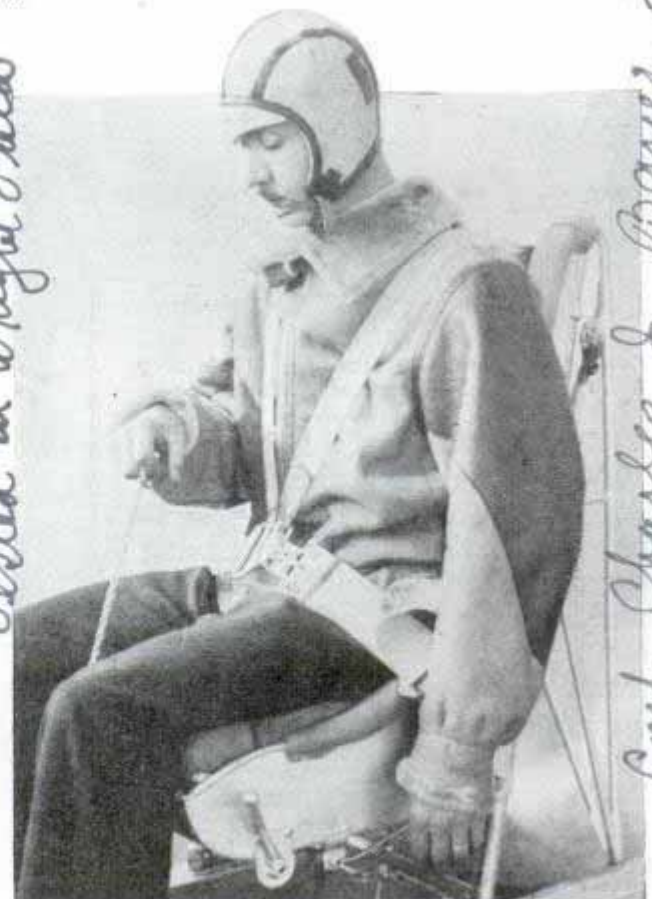
Quick pull on chain tightens belt in emergency and pilot can free himself by flicking lever in buckle
