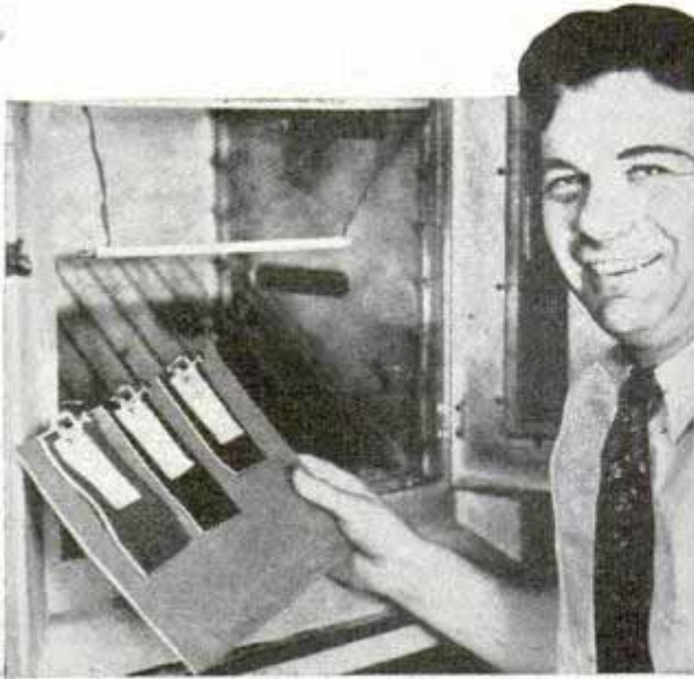
Ready to test automobile leather samples with cigarette papers in oven
