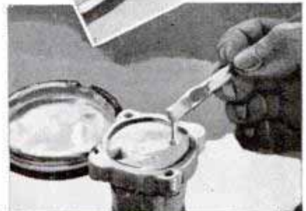
SCREWS IN ELECTRICAL FIXTURES HELD PERMANENTLY IN PLACE . . .
