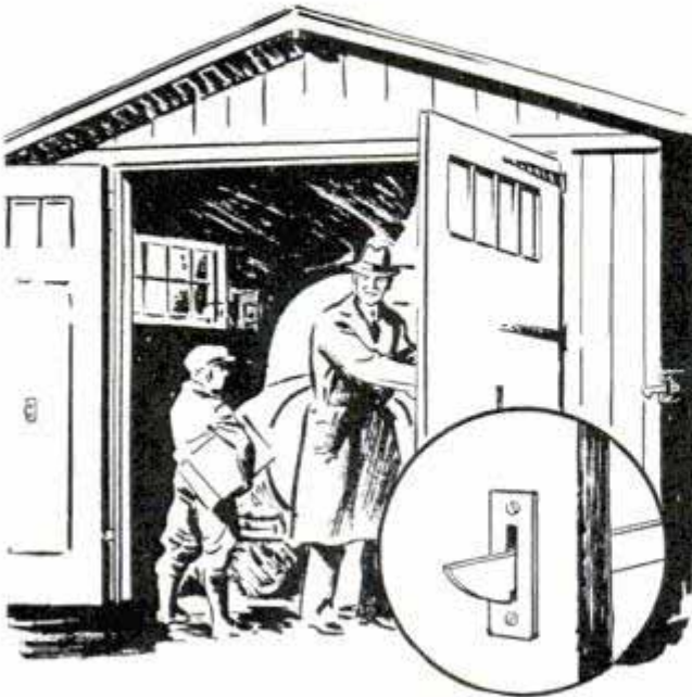
When these doors are opened against the side of the garage they are automatically engaged by latches
