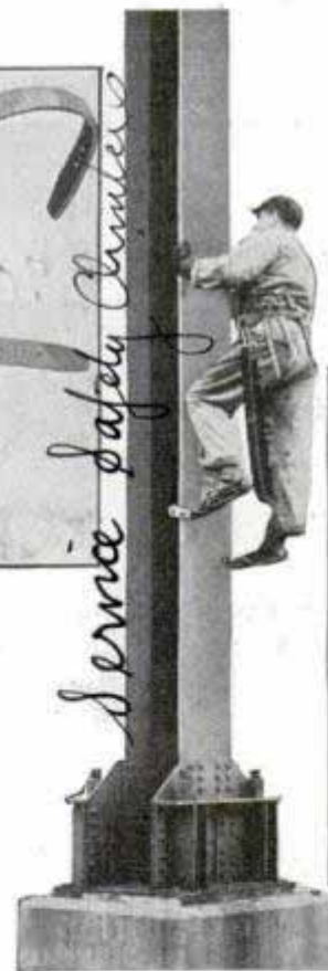
Climbing irons for scaling steel girders in use. Inset, views of the irons
