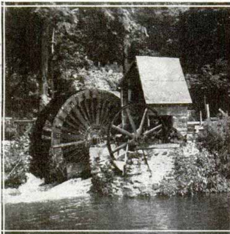
Nine-foot water wheel drives direct-current ten-kilowatt generator supplying power for electric cooking and lighting at inn
