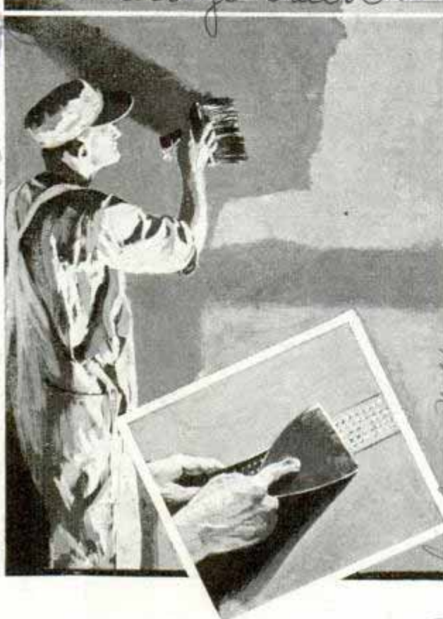
Slapping cement over recessed joint, workman applies fibrous tape and then smooths cement over it
