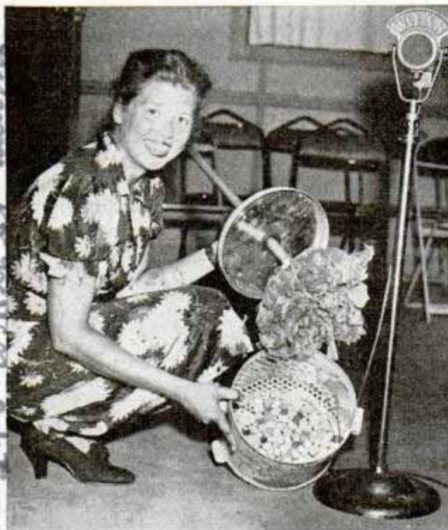
Tiny wooden cubes beat dust out of mop and it collects in bottom of can instead of flying in window
