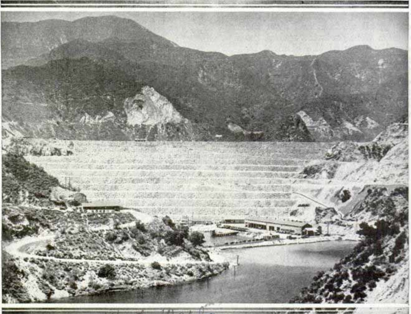
Terraced earth and granite dam is three-quarters of a mile wide at top, spanning San Gabriel canyon near Azusa, Calif. Its base is nearly 2,000 feet thick and there is room on top for a forty-foot road
