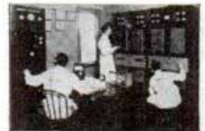
The KXBY Transmitter room which you will actually operate as part of our "Experience-while-Training" Plan.
