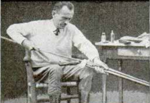
Here is the correct method of cleaning a shotgun—from the breech
