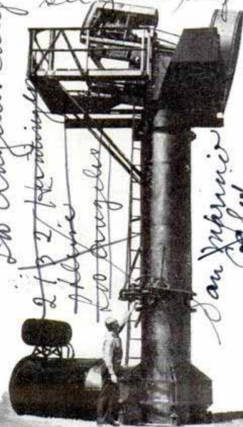
Hot air from boiler at base is shot up thirty-foot stack and blown over orchard by oscillating fan
