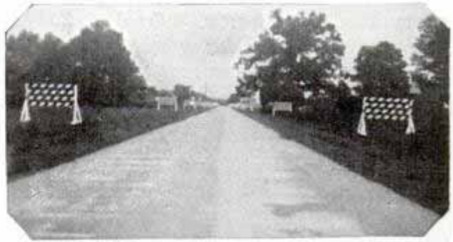
Road signs which appear to close in on driver as car approaches intersection
