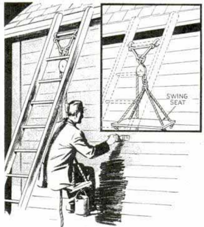
This workman paints a wide strip from top to bottom of building without getting off his seat
