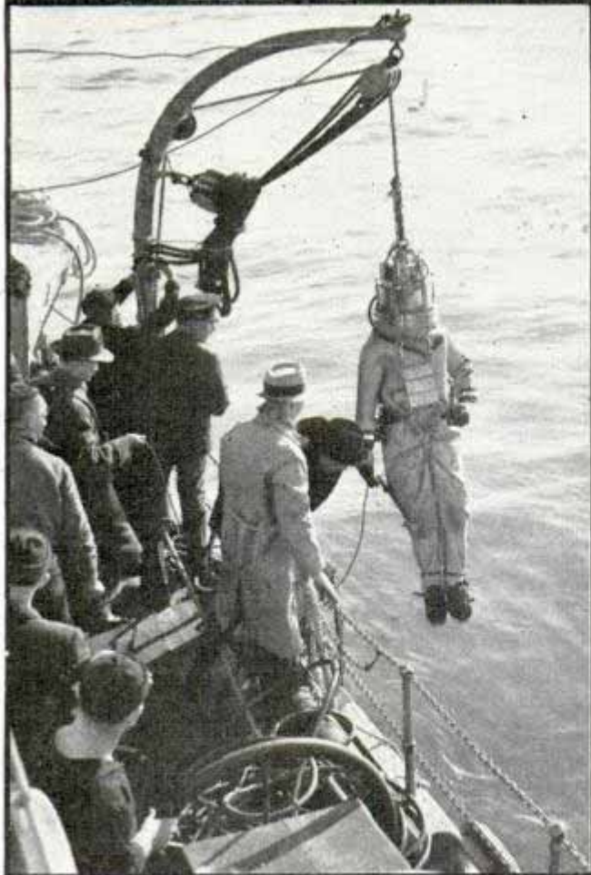
Top, air escaping from diver below. Bottom, Diver Nohl being lowered over side
