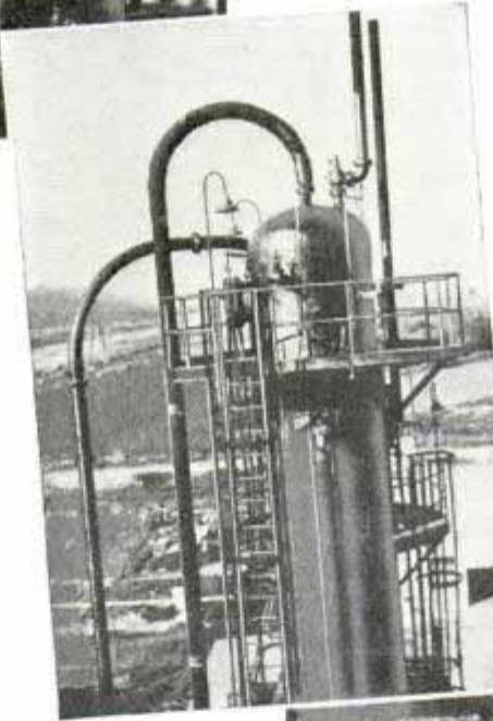
Above, driver testing power of new high-octane gasoline. Right, top of cracking tower in which evaporated petroleum molecules are broken apart into gasoline molecules
