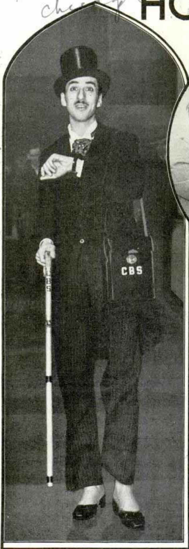
Wrist watch of walking radio reporter is microphone; cane contains antenna and leather case holds batteries. In circle, broadcasting sound of milking
