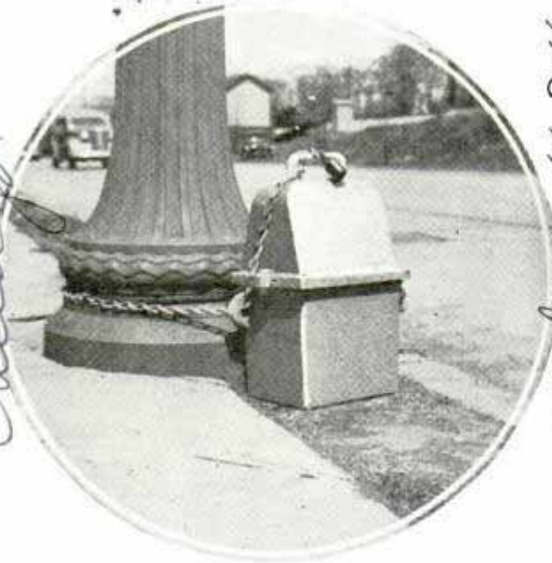
Chained to pole is traffic recorder which receives impulses as vehicle crosses strip laid on pavement
