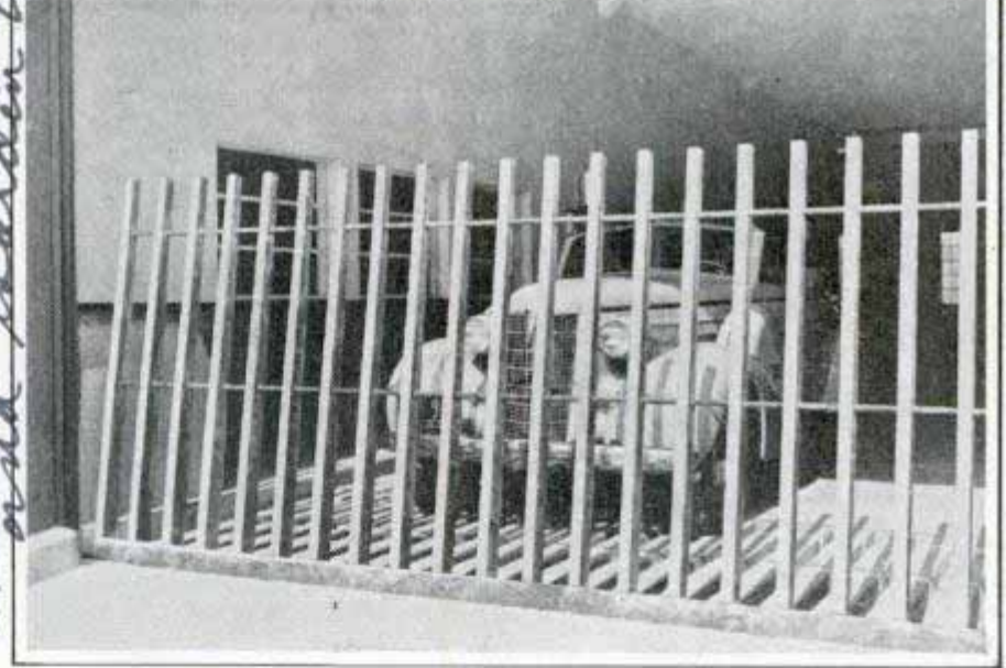
Top, a customer drives in to make a deposit at tiny window at left. Bottom, steel gate which rises from roadway to halt escaping bandits
