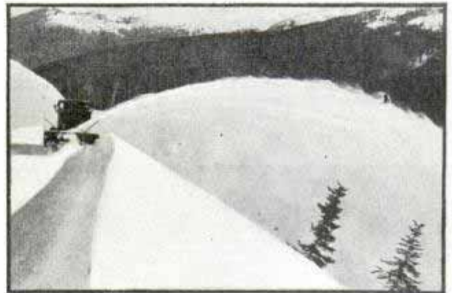
Courtesy U. S. Bureau of Public Roads Rotary snowplow throwing snow 150 feet down slope as it clears Berthoud Pass
