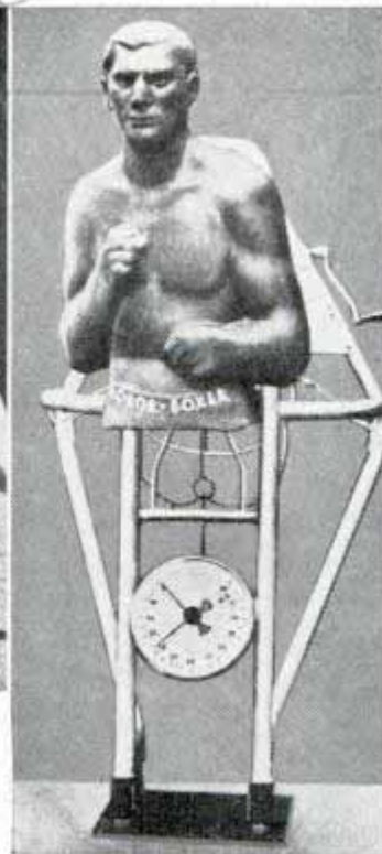
Left, boxer in training with robot sparring partner which weaves and rebounds in unexpected ways. At right is the robot with meter registering power of boxer's punch
