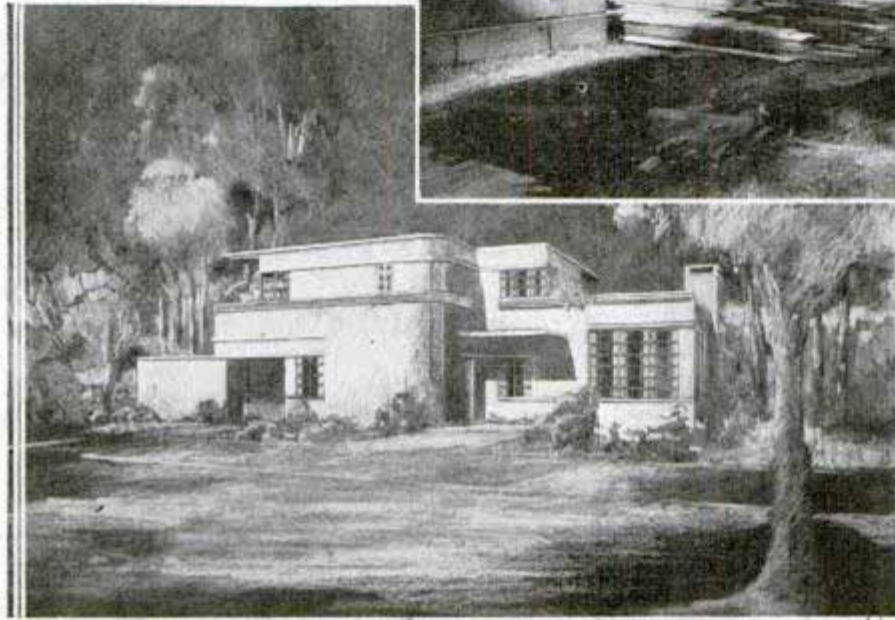
Above, house of lightweight concrete under construction, showing beams and posts of concrete instead of traditional wood framing. At the left is architect's drawing of the completed house. This light concrete is made of cylindrical pellets of clay and shale fired in a kiln
