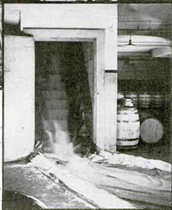
Top, sweeping out water. Center, unloading salvage apparatus. Bottom, emptying water from building
