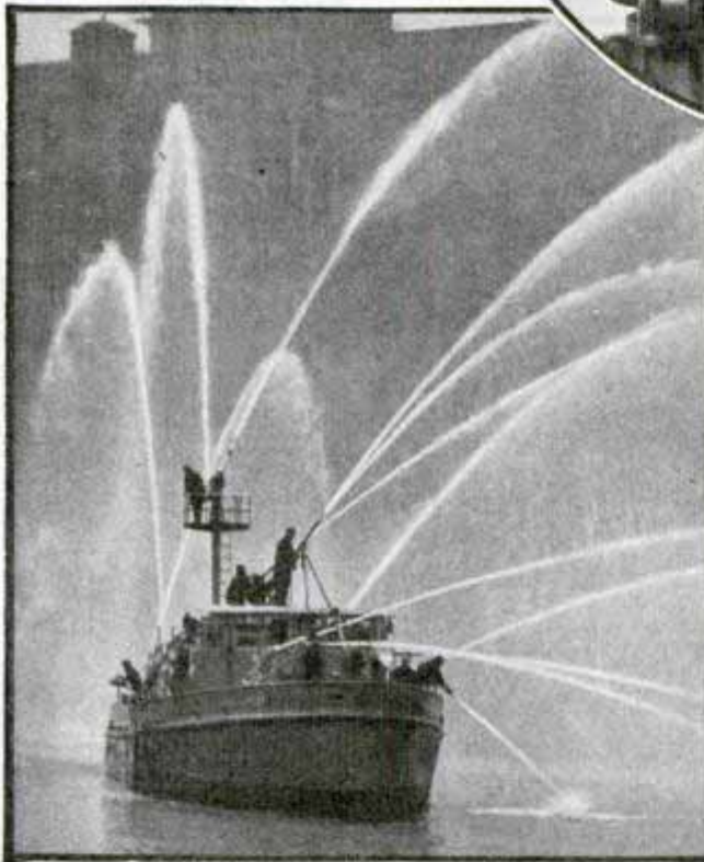
Three views of new fire-fighting boat. Left, more than a dozen streams of water at once. Center, controls for one of the nozzles. Right, tower which may be raised or lowered hydraulically in a few seconds
