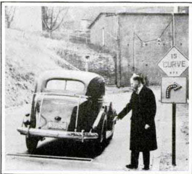
Switch set in roadway operates traffic signals at dangerous corner ahead
