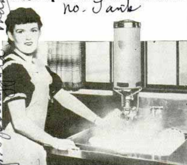
no. Tank Instant hot-water heater over sink saves cost of installing usual dual pipes for hot and cold water
