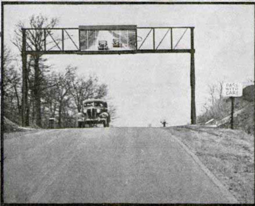
Left, prism installed above dangerous hilltop. Drawing shows how motorist watching prism can see cars approaching beyond the crest of hill
