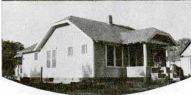
Church in Aurora, Mo., before, during, and after it was transformed into a six-room bungalow
