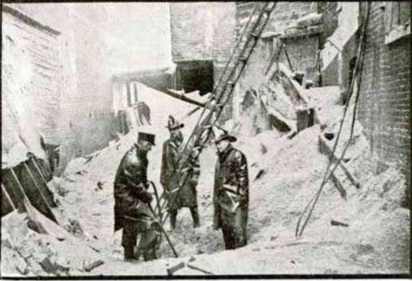
Top, demonstrating explosive characteristics of dust. Center, apparatus used by government engineers in studying heating of hay. Bottom, ruins of plant in which malt dust exploded at Buffalo, N. Y.
