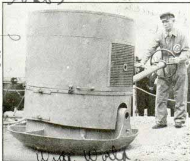
Workman guiding the heavy tamper which maneuvers over gravel road pounding its surface smooth
