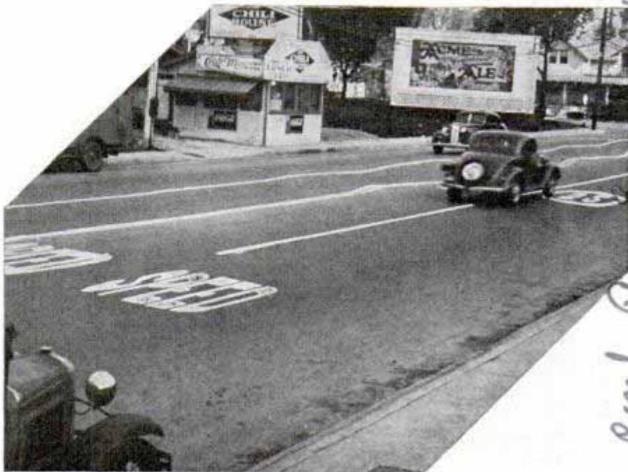
Lettered in white, the word "Speed" in each traffic lane catches eye of motorist and a few feet farther white figures tell him the speed limit
