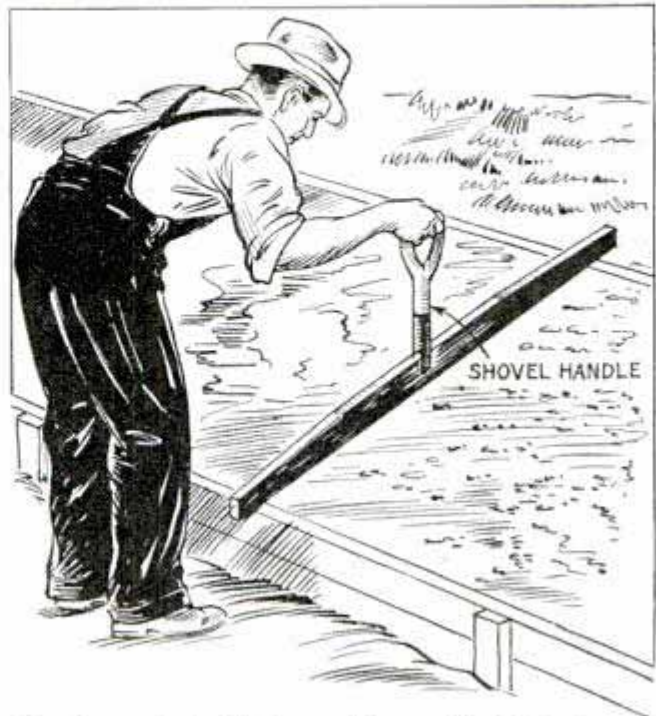
Handle on straightedge enables worker to test newly poured concrete surfaces without kneeling
