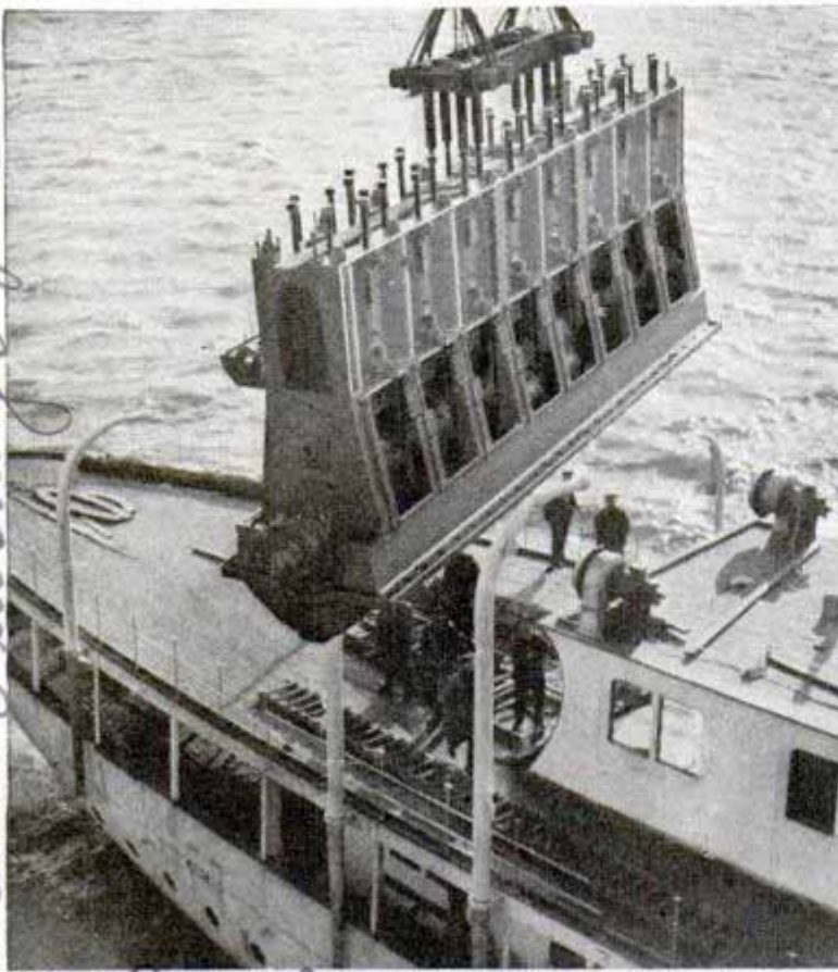
Here is one of the two Diesel engines. Weighing forty-five tons, it is being handled by special floating crane
