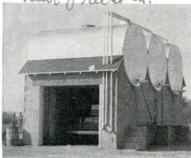
Garage built by oil dealer has three tanks for its roof, the seams made leakproof by elastic compound
