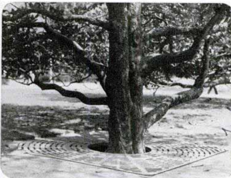
Tree in Washington, D. C., protected by grating which serves as sidewalk but allows water, air and light to reach base
