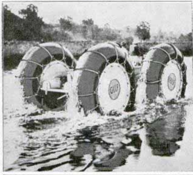
Three views of "marsh buggy" in operation. Top, circle, and bottom, left, the vehicle navigating in deep water. Top, left, the buggy emerging from the water to travel marsh or highway without changes in its equipment
