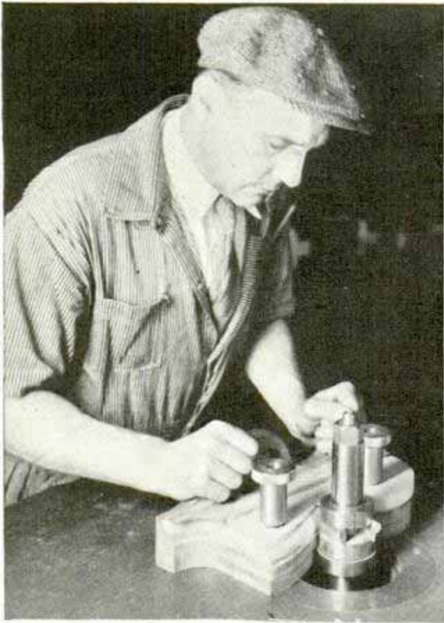
Shaping test, above, for southern hardwoods and, right, testing relative effectiveness of fire-retarding chemicals for wood
