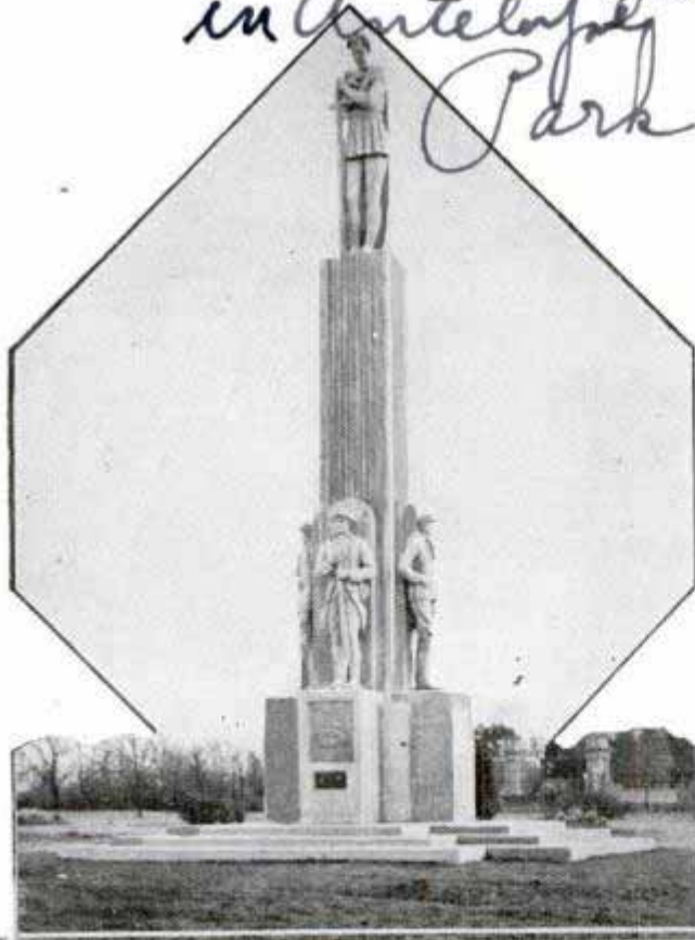
This thirty-two foot memorial is constructed of concrete and crushed marble
