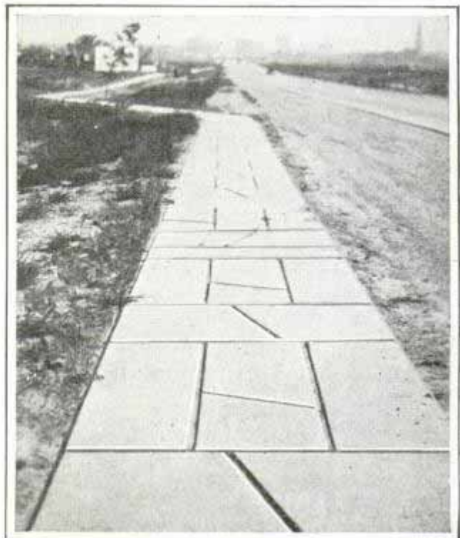
This flagstone sidewalk was made by using dividing strips between the concrete forms
