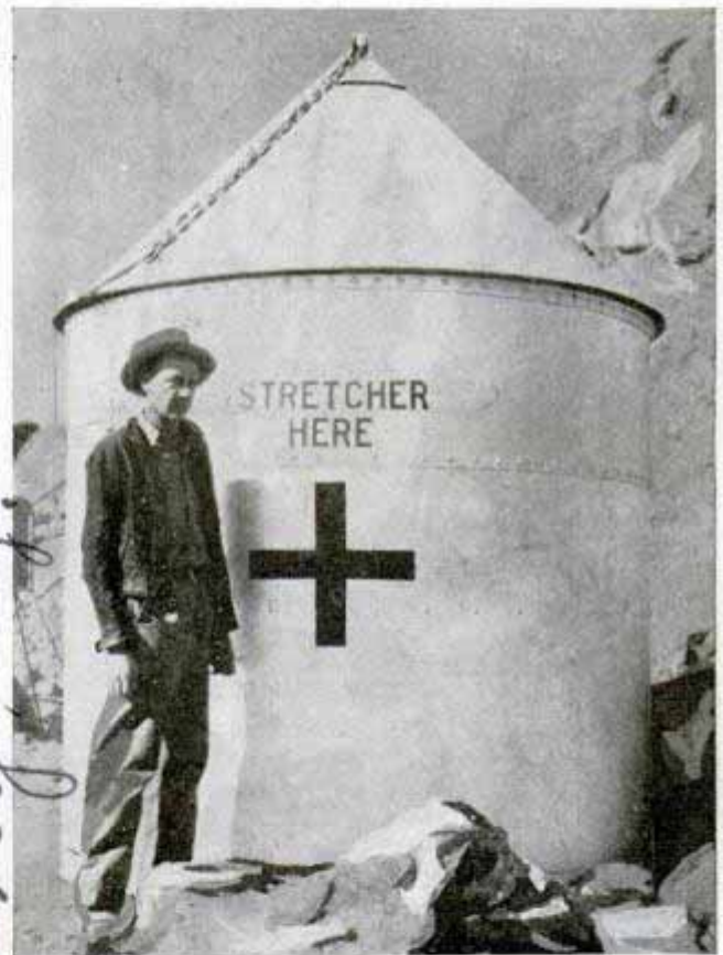
One of the steel shelters in open mine. Note that it also serves first-aid purposes
