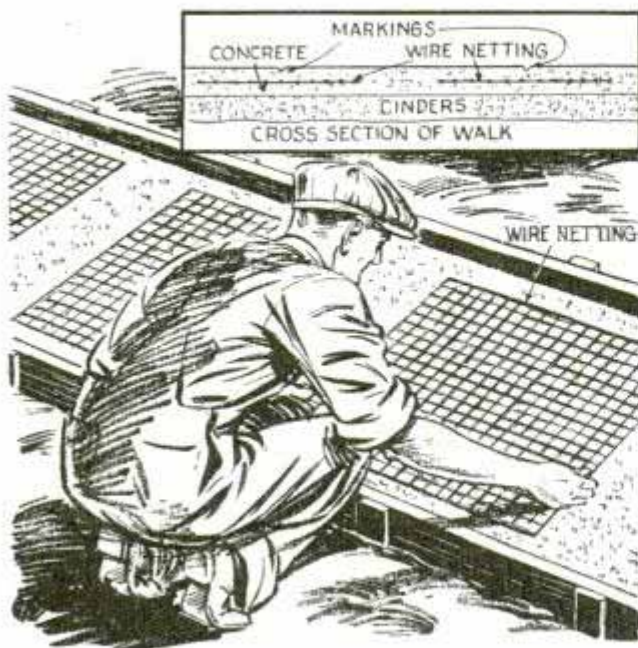
Wire mesh imbedded under expansion joints of sidewalks to avoid uneven raising of the sections
