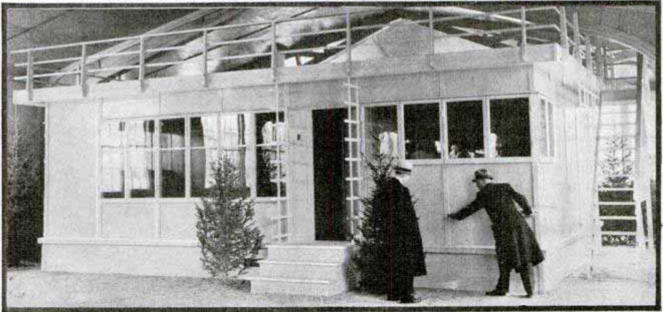
Top, measuring comparative amounts of spring and summer wood in specimen. Below, demonstration low-cost, prefabricated, all-wood house covered with panels of glued plywood
