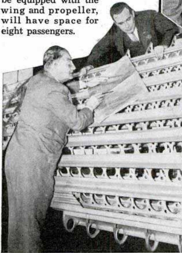
White wood Top, comparing new lightweight, metal propeller with old wooden type. Bottom, section of wing, said to be almost invulnerable to gunfire.
