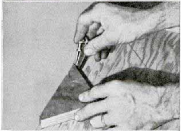
FITTING CABINET INTO CORNER
