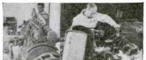
Diesel Generating Unit. Diesel Converted Ford Auto
