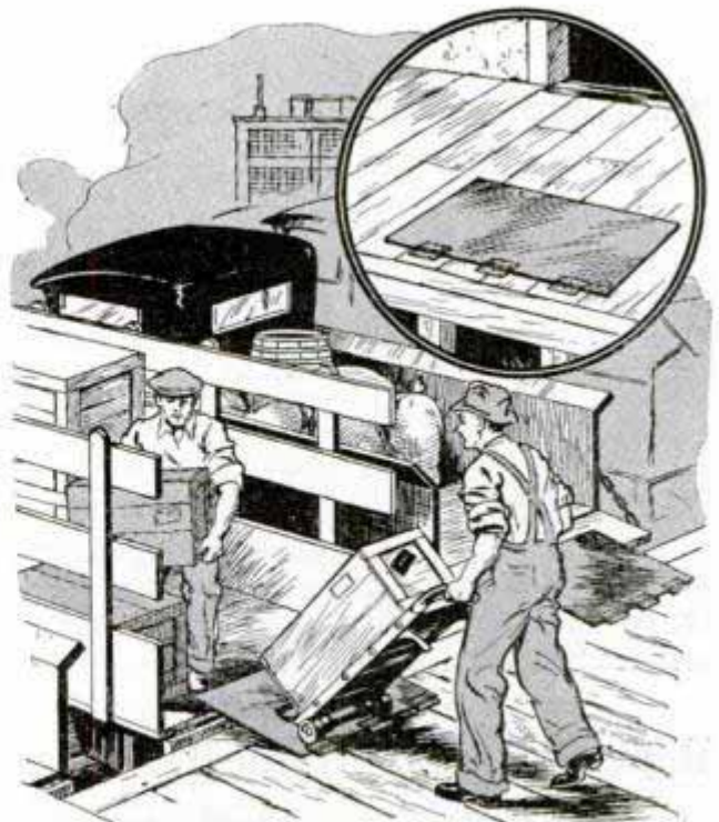
Heavy steel plates between trucks and loading platform provide smooth surface
