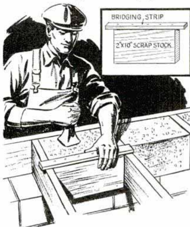
"Walling out" over foundation between the floor joists with concrete of stiff consistency
