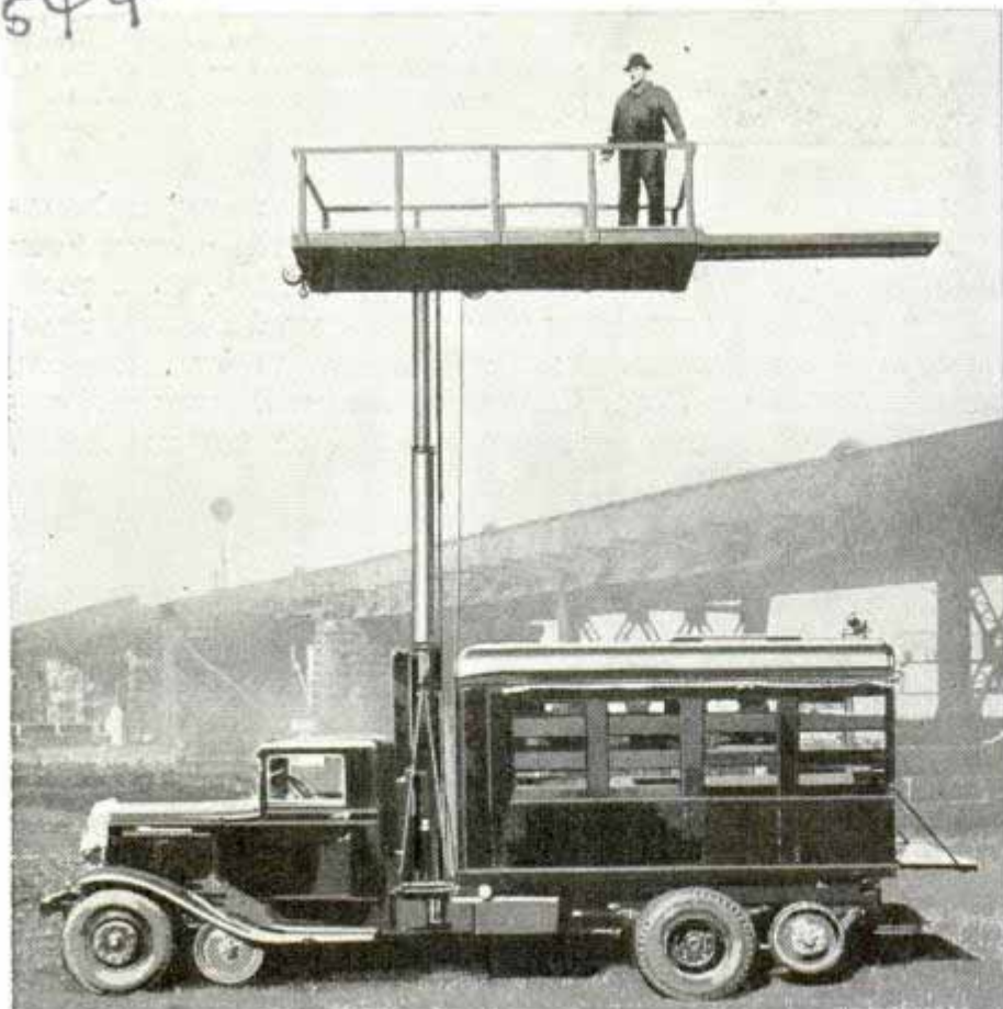
Trouble-shooting truck for electric railroad rides on rails or road
