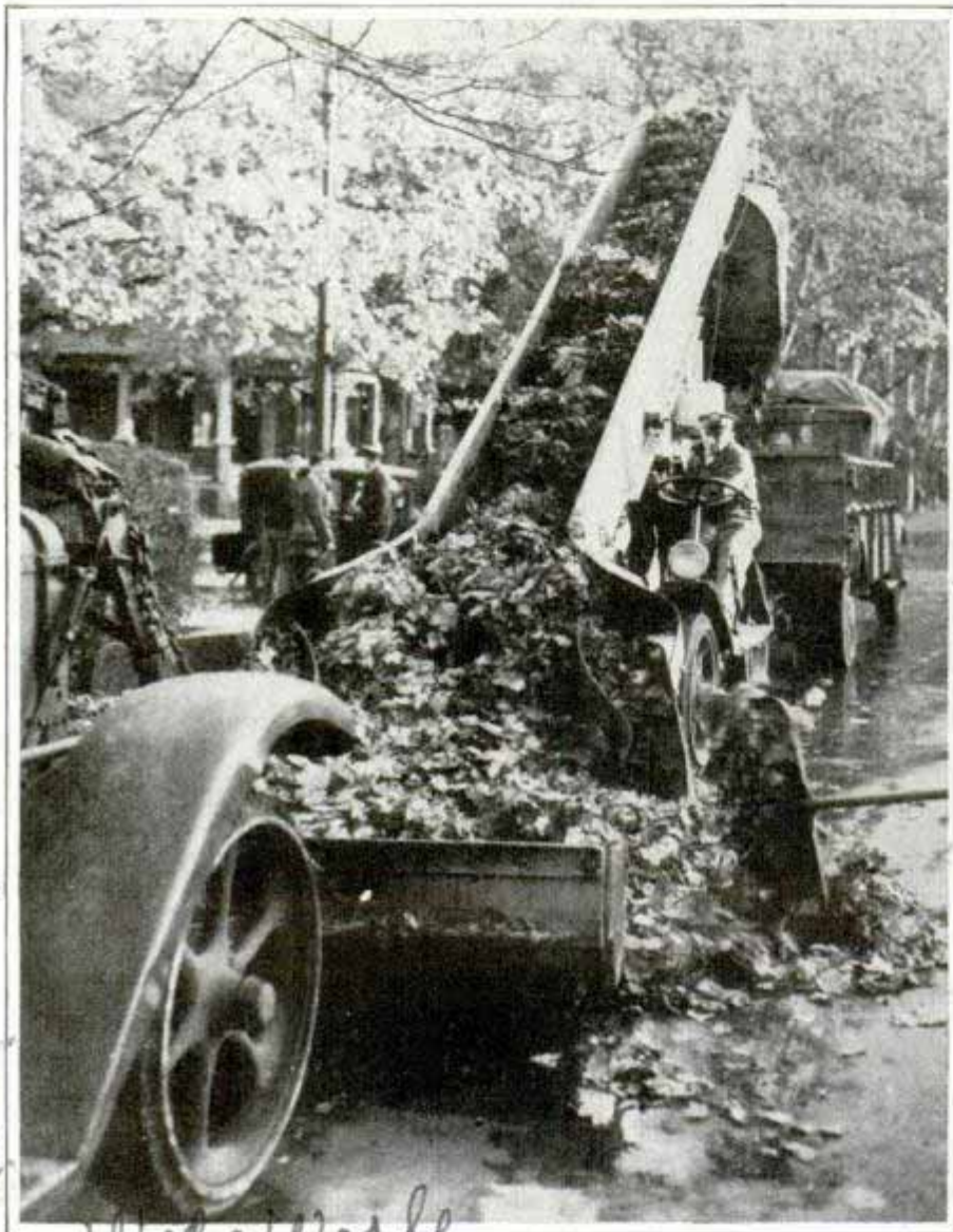
Brooklyn keeps its automatic snow-loader at work out of season, using it to load trucks with piles of fallen leaves
