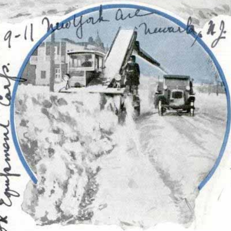
Top, a "V" plow mounted on a flatcar. Bottom, automatic snow-loader clearing a city street. Revolving disks feed the snow piles to an endless conveyor which loads two trucks per minute
