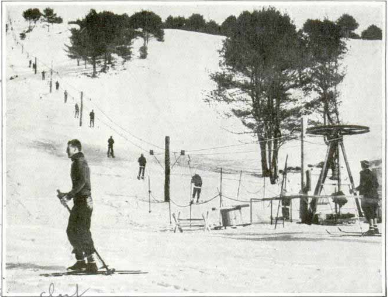
This is one way to make skis more popular. Skimming down a mountainside takes skill but little effort; climbing up takes plenty of effort, so a cable was installed at Hanover, N. H., to haul skiers to the top
