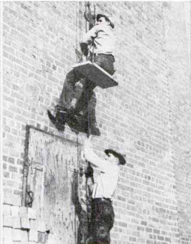
Stack worker on the job. This particular stack is more than 500 feet high. Right, worker preparing to ascend. Note small seat on which he sits to repair brickwork hundreds of feet in the air
