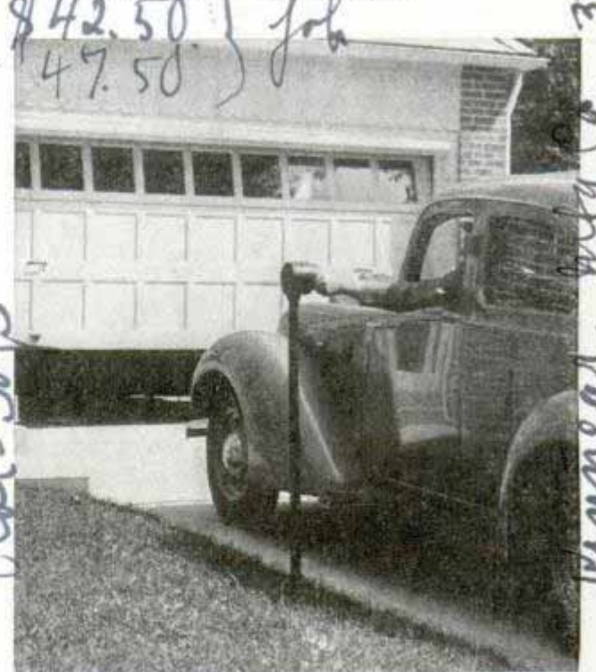
Motorist opening his garage door by pressing electric button after turning key in post beside driveway
