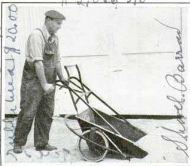
Workman loading the shovel-nosed wheelbarrow
