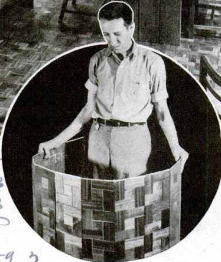
Parquet floor in room shown above was made of two by six foot sections, one of which is illustrated below as it came from factory, prefinished and ready for laying with special adhesive
