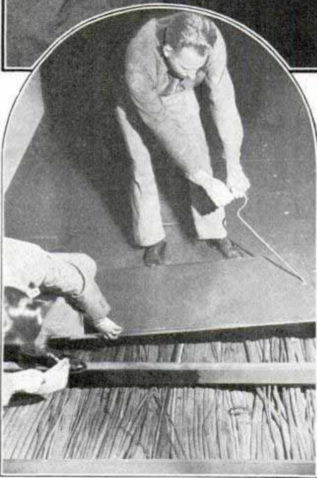
Studio engineer at controls during rehearsal of air program. Below, lead-coated cables laid beneath the floor connect control room with broadcasting studios throughout Radio City
