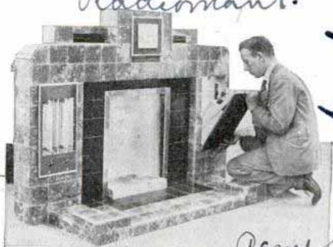
Installing radio receiving set in mantelpiece
