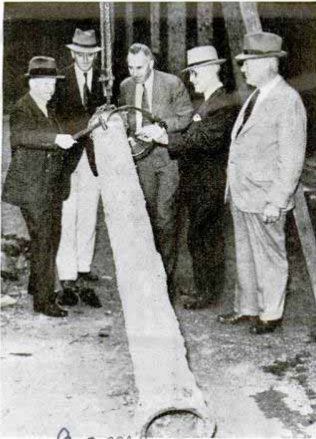
Officials examining old water main which had been in service for a century
