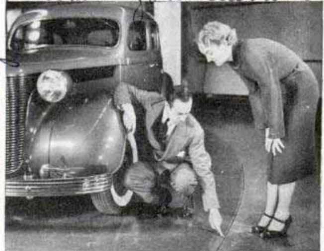
Pointing to separation between floor and revolving platform in auto showroom
