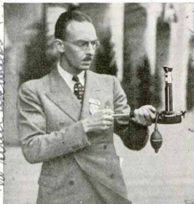
Taking a sample of air with meter which analyzes it and shows amount of dust
