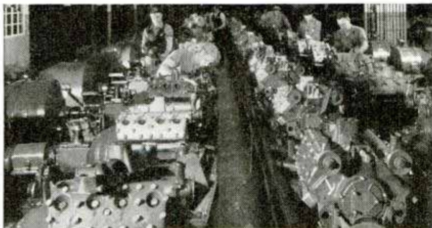
(Above) Reconditioned engines are block-tested and given the same rigid inspections as new engines.
