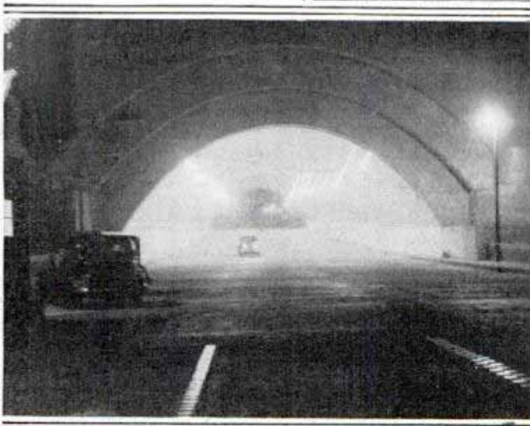
Air view of the San Francisco-Oakland bay bridge as it appeared just before being opened to traffic. Below, night view of tunnel through Yerba Buena island, connecting the San Francisco span with that on the Oakland side. The tunnel is seventy-six feet wide
