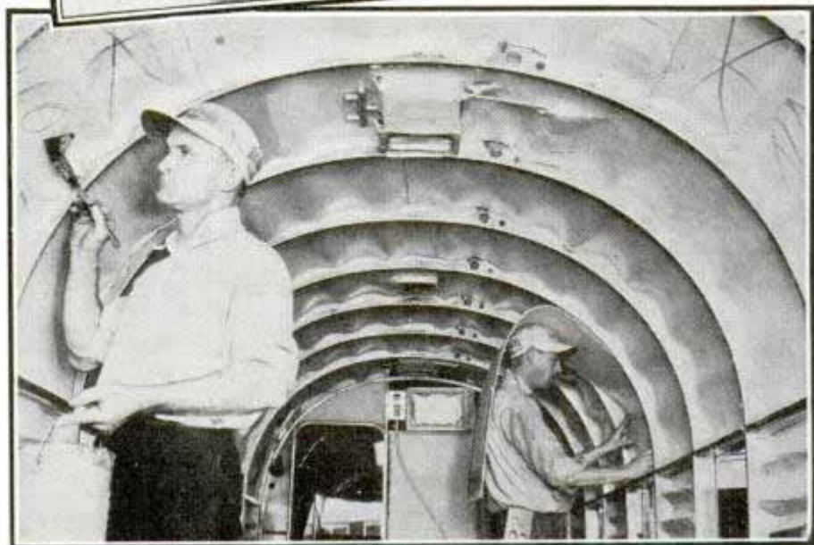
Top, noiseproof wall withstands fire for an hour. Center, taking outside temperature of wall. Below, soundproofing an airplane cabin
