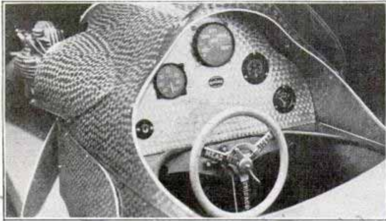
Top, drawing of the snow sedan as it would appear on winter sports course. Center, the "bronco," a motor bike equipped with tractor tread at rear and runner at front. Bottom, driver's compartment of the speedy power sled which is capable of 150 miles per hour on ice. Its steering wheel controls the front runner
