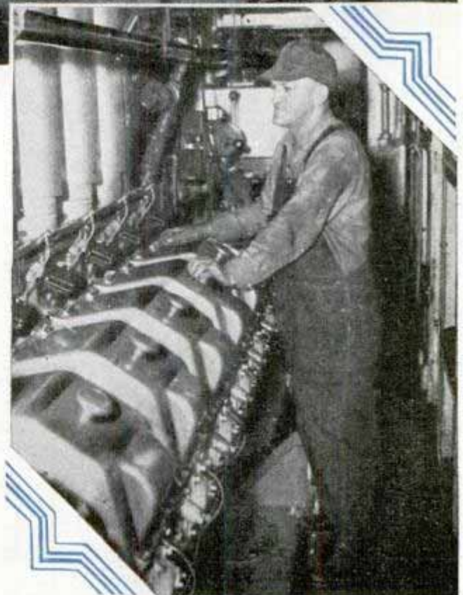
Power plant of the "City of Denver" and engineer at controls of this modern streamliner
