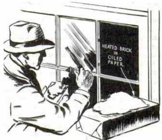
Glazier keeps putty soft on cold days with the aid of a heated brick
