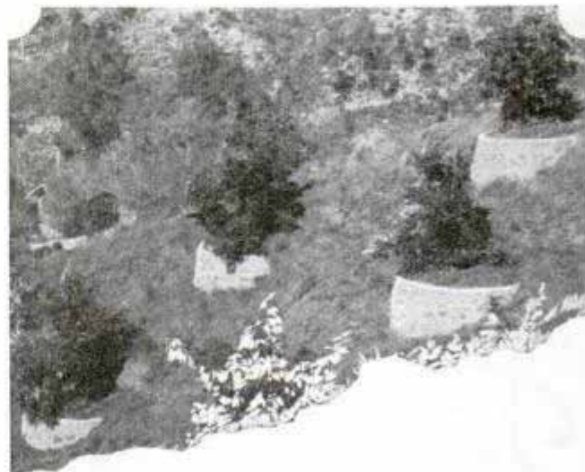
Half-circular walls on the downhill-side of these trees check erosion and help hold moisture
