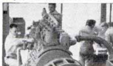
Students servicing Fairbanks-Morse Diesel power generating unit.
