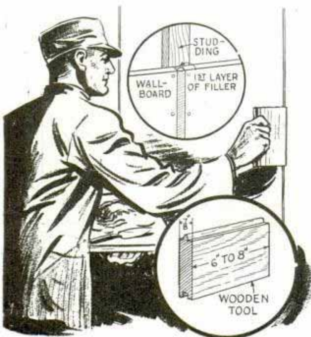
With this tool, it's easy to press filler firmly into joints between wallboard panels
