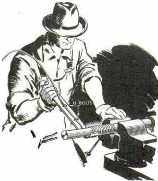
You can do a neat job with this winder, which has an adjustment to gauge the tension on the wire
