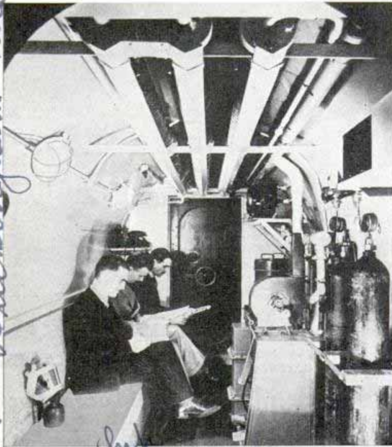
Self-sufficient chamber built by London concern to shelter employees during gas attack. It has oxygen, food, and water
