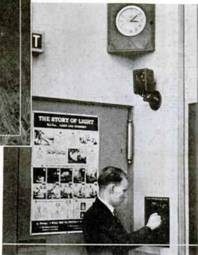
Top photo courtesy Westinghouse Lamp Co. Top, beetle trap and light. Below, under clock is photoelectric cell which turns on lights in school-room when outside light becomes weak
