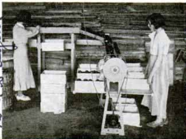
Tomato grader in operation. This type handles 1,000 pounds of tomatoes per hour
