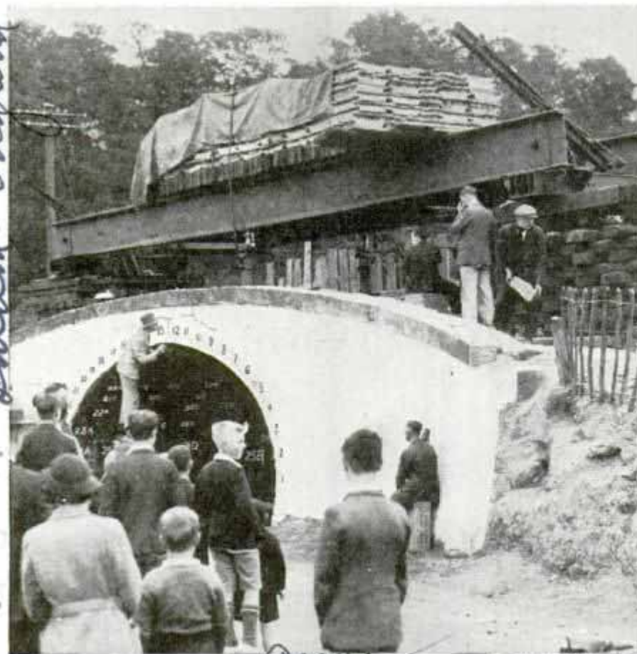
Old bridge at moment it was subjected to load of ninety tons. Note cracks in the arch. Shortly after picture was taken, it crashed
