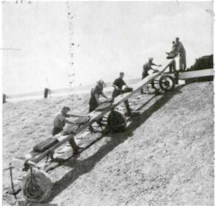
Sodding incline with aid of odd carrier. Note how sod is pushed down table to point where worker removes and lays it on ground
