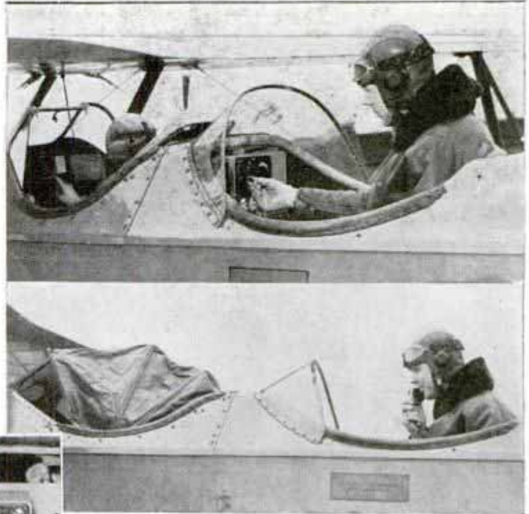
Top, student and instructor ready for flight. Bottom, student under blind-flying hood. Left, control board by which instructor guides student
