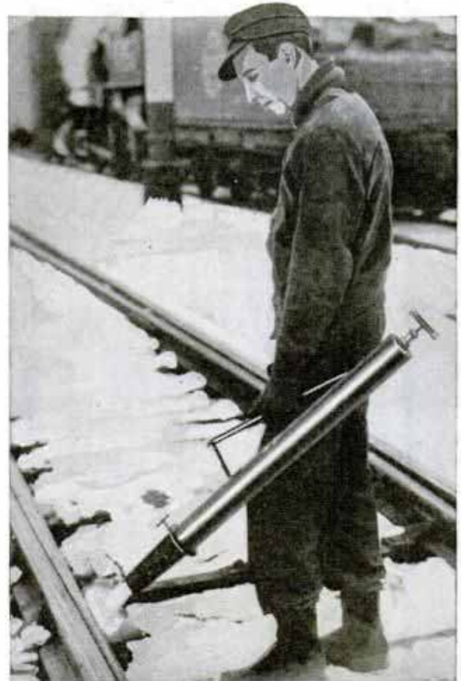
This torch quickly clears switch of snow and ice and it's handy for burning weeds
