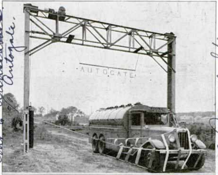
Big truck being halted by crossing gate which "stretches" 100 feet to bring vehicles to gradual stop. Note harness gripping front of truck
