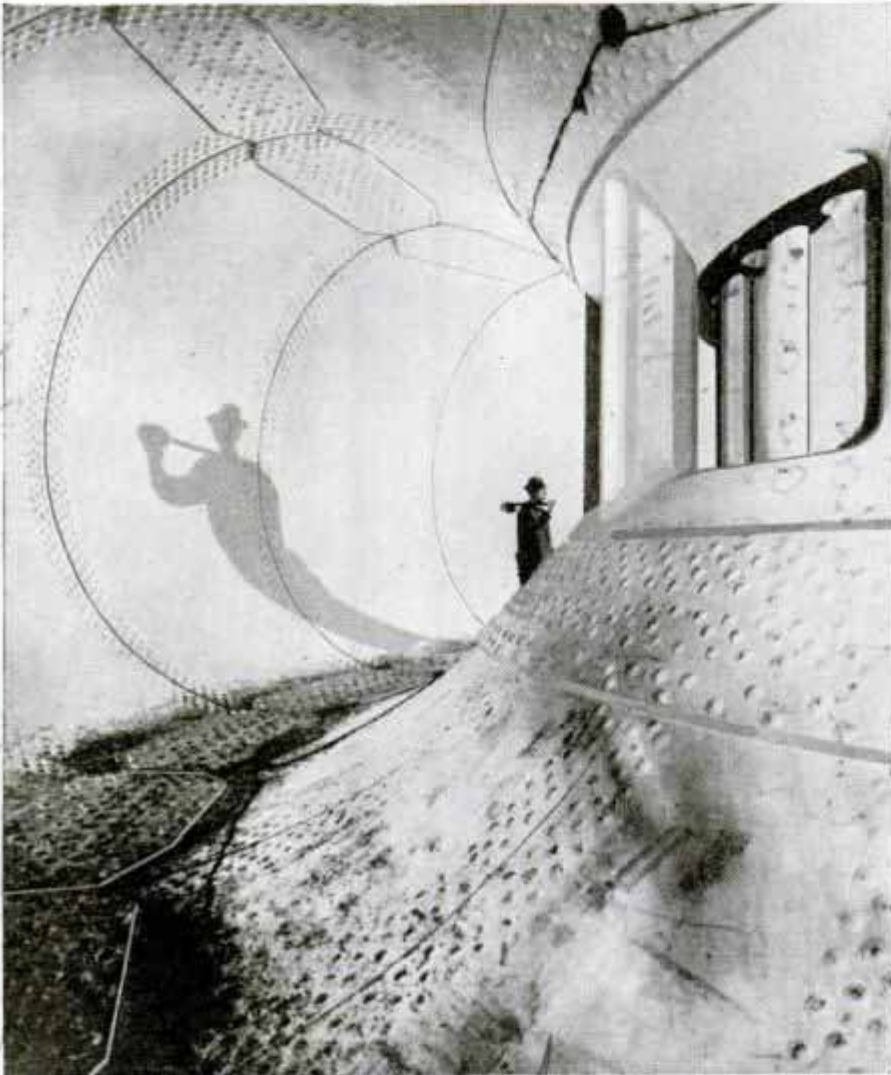
Lights cast weird shadows inside this vast tunnel, the scroll case through which Tennessee river water will flow to the Norris Dam turbines
