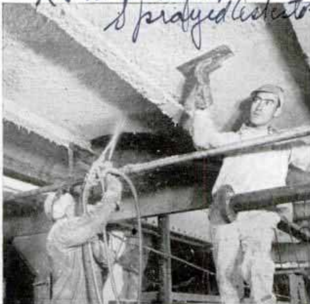
Applying a coat of asbestos on walls and pipes
