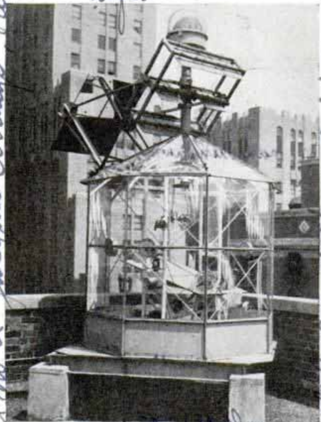
Wide World This odd arrangement of mirrors reflects sunlight into rooms on dark courts and airshafts
