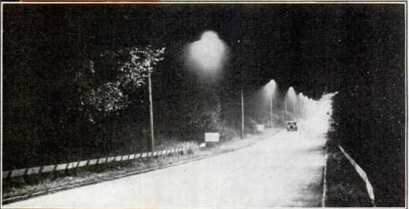
Road illuminated with 400-candlepower incandescent lamps and reflectors. Left, types of fatal and non-fatal accidents
