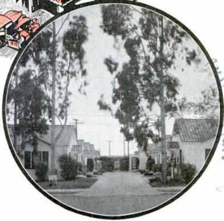
Motor court in Santa Monica, Calif. Note the U-shaped court and the substantial construction of the individual cottages in this lodge
