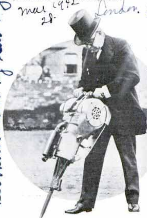
Official trying out the noiseless road drill which is operated by gasoline engine
