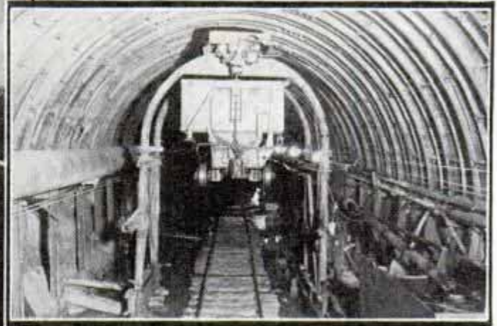
Left, end of siphon section. Right, "cherry picker" which enables cars to pass. Below, mechanical hands which pat concrete and wheeled concrete hopper
