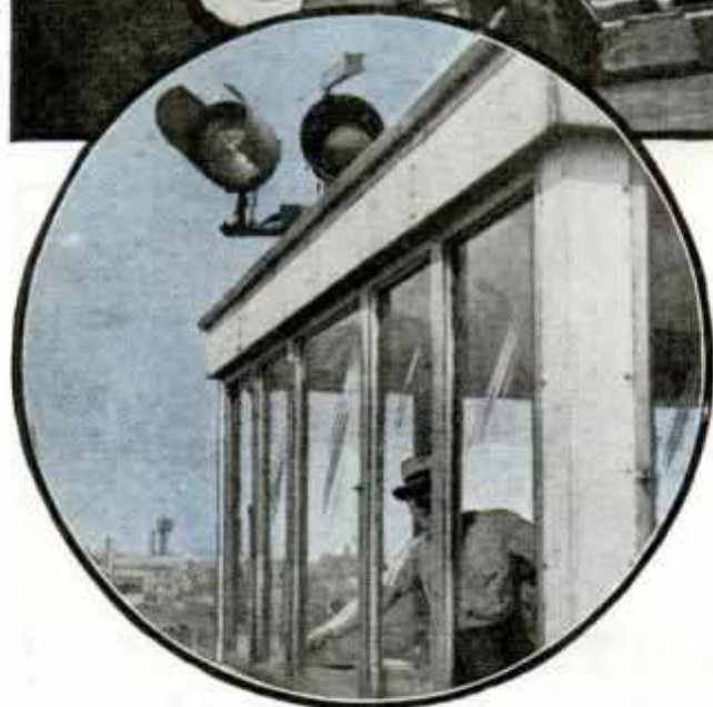
Stop-and-go light on control tower, and electric oil heater developed by TWA mechanics
