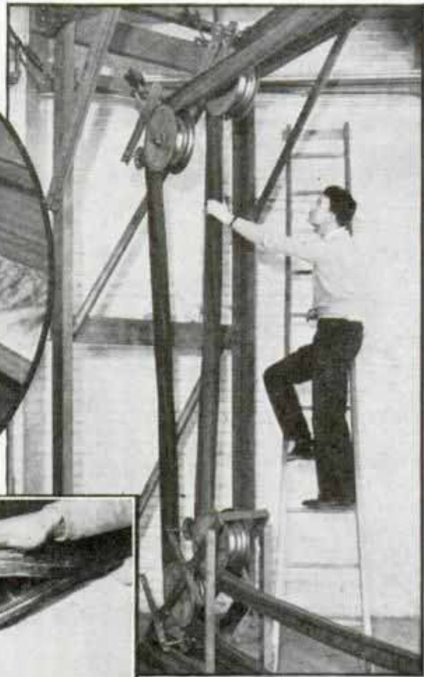
Above, rubber pipe line in industrial plant. At left, how its two halves open, discharge their load, and seal themselves together again. Chain embedded in each side of pipe reinforces it
