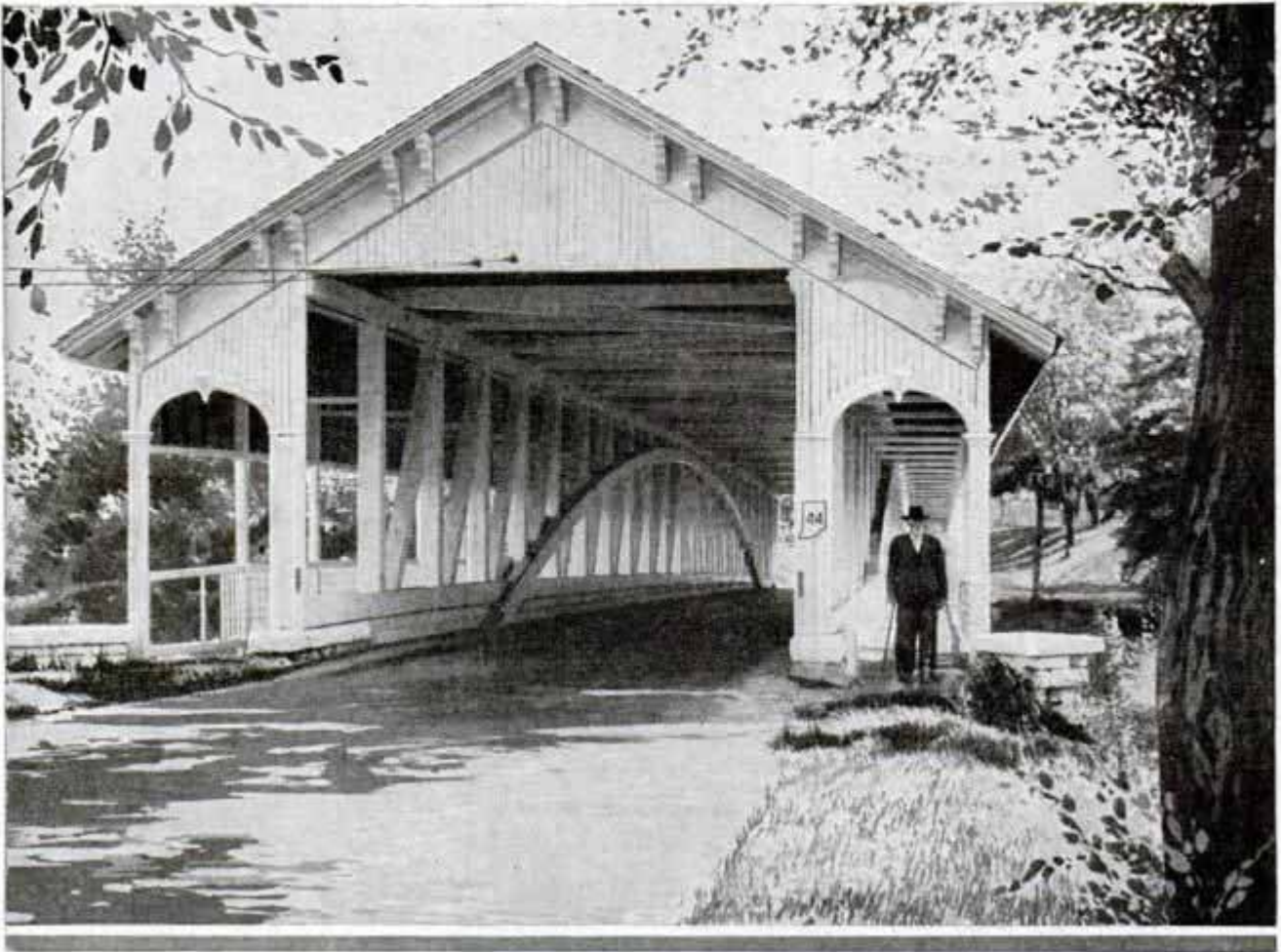
One of the few remaining covered wooden bridges. This one is more than fifty years old and is still in service near Rushville, Ind.
