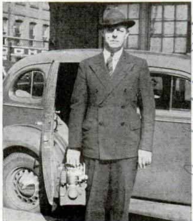
Air-cooled gasoline motor generates electricity to light a small house. It weighs forty pounds
