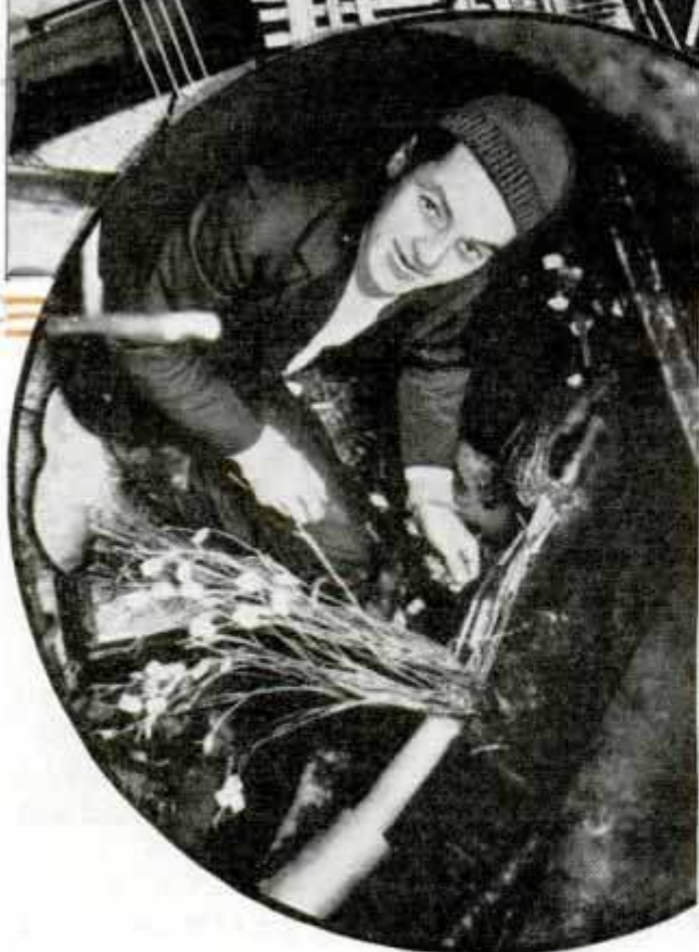
Top, this freak accident made work for maintenance men. Below, repairman splicing a damaged telephone cable after flood
