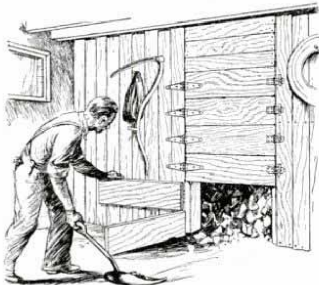
This coal-bin door opens in sections to remove fuel from any level desired
