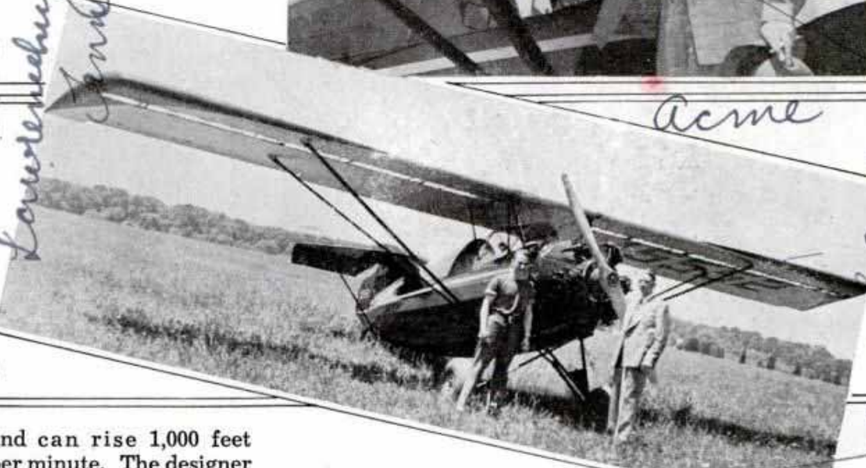
Plane with air slots in wings which permit some of air to pass through. The designer claims that this feature increases the lifting capacity of the wings and stops any tendency of the craft to go into a spin
