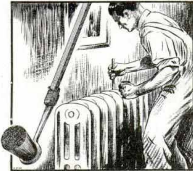
Restricted places behind a radiator are easily painted with a shoe-polish brush
