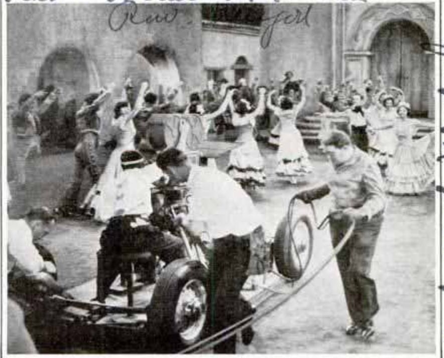
Rolling this camera dolly back and forth keeps the dancers in proper focus. A twelve-inch variation calls for a retake
