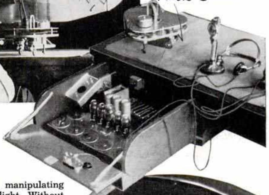
Left, instructor directs student pilot by telephone as he watches maneuvers of model plane. Below, radio and phone set with which instructor simulates actual flight signals. Bottom, instrument board of plane
