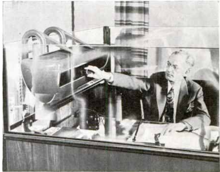
Glassed-in office space, open at top, is an "oasis" of comfort on hottest day as an air-conditioning unit suspended on side supplies cool air
