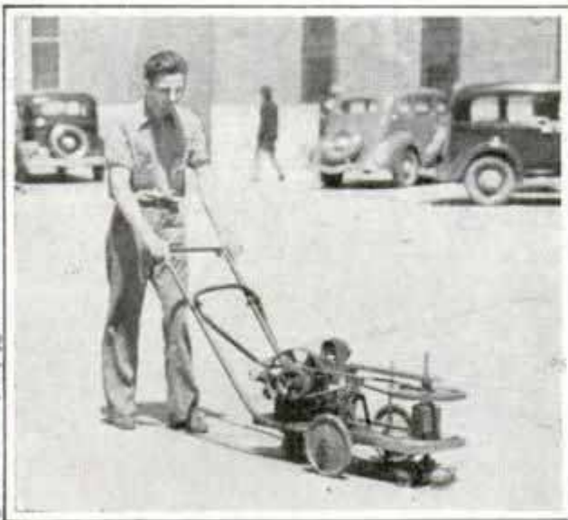
Revolving brushes on homemade street cleaner sweep line where traffic lane is to be painted
