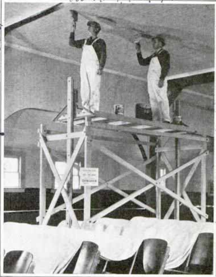
Elevating scaffold for painters and decorators with platform which is moved up or down by turning two cranks. It can be assembled or knocked down in less than an hour
