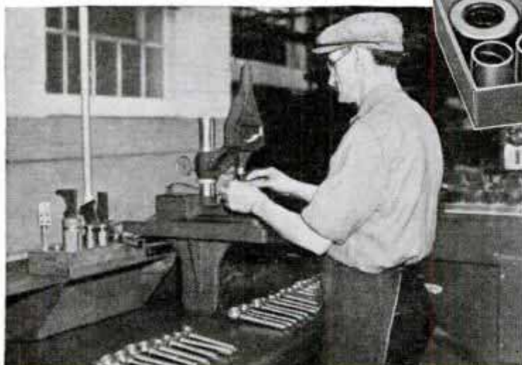
Inspecting spindle bolt diameter on visual indicator which has 1000 to 1 magnification—1/1000 inch looks like 1 inch on scale.
