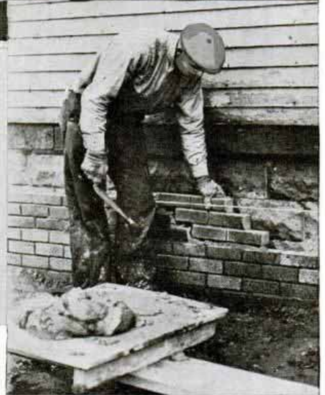
Top, making six-in-one brick unit, and the resurfaced house. Below, wall section showing insulation space, and laying the brick veneer wall
