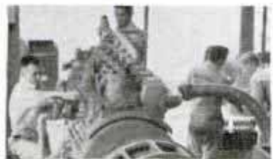
Students servicing Fairbanks-Morse Diesel power generating unit.
