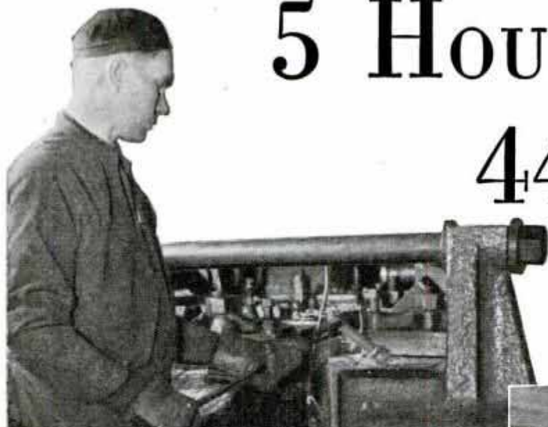
Forging spindle bolt heads.
