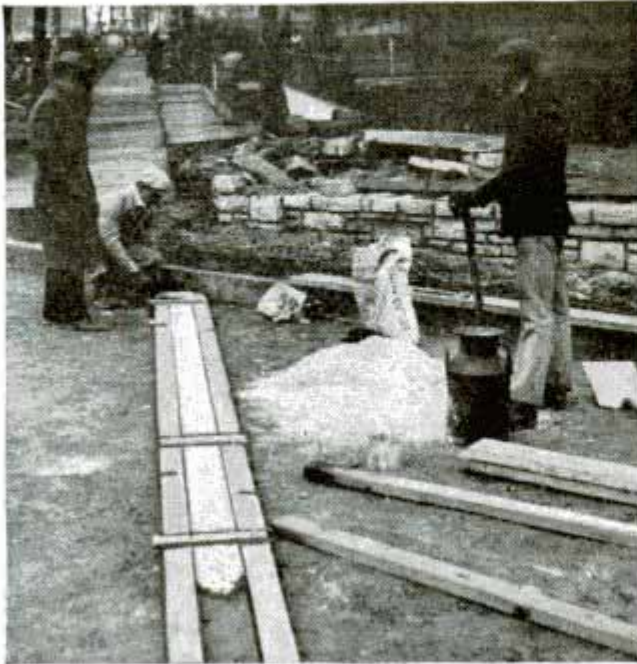
Inlaid lines of white cement contrast sharply with darker street paving so that they are easily seen
