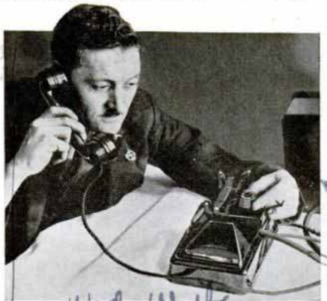
Turning knob on telephone, deaf listener can amplify voice in receiver to suit his ear
