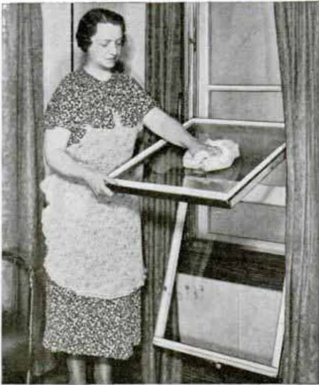
Both sashes can be brought down and tilted inward to a position convenient for washing either side
