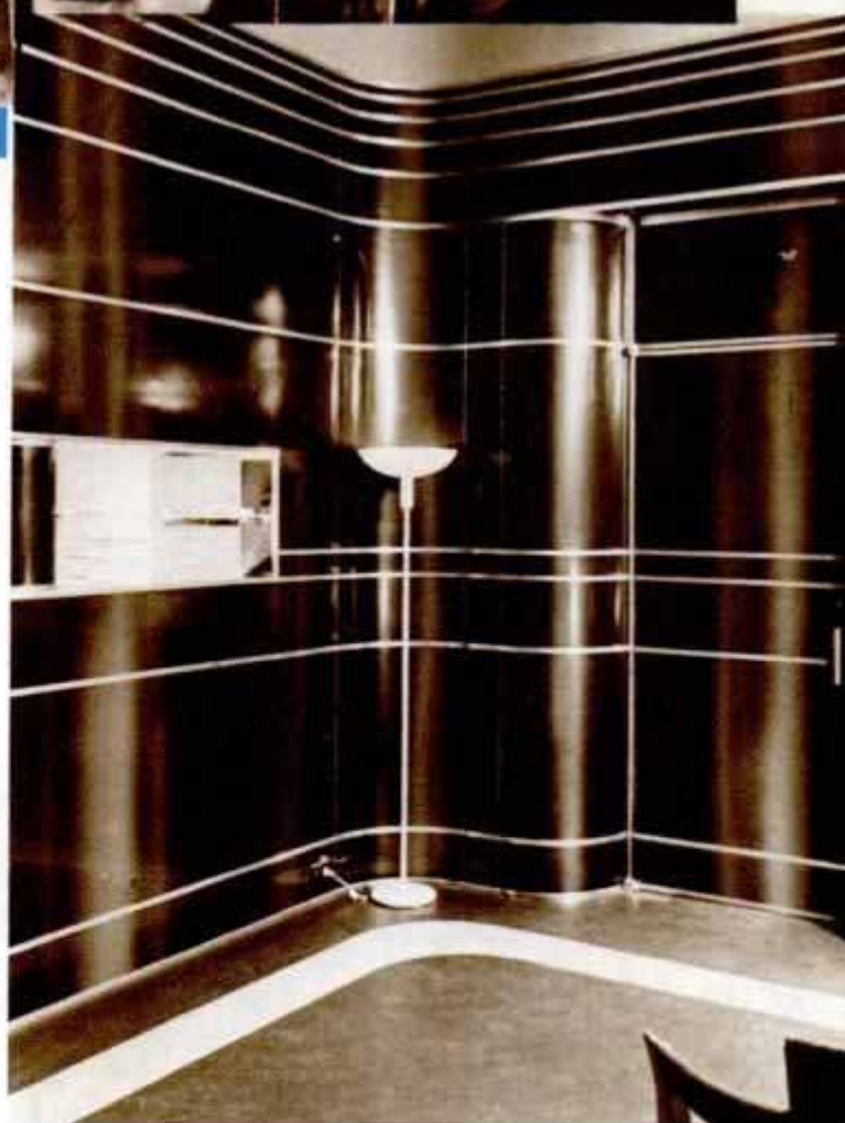
DOUBLE radius corner constructed of prefabricated porcelain enameled sections. Top, laboratory technicians testing raw materials used in making porcelain enamel.
