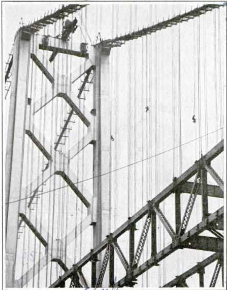
Like flies caught in a giant spider web, these workmen hang suspended as they paint the cables of the San Francisco-Oakland bay bridge
