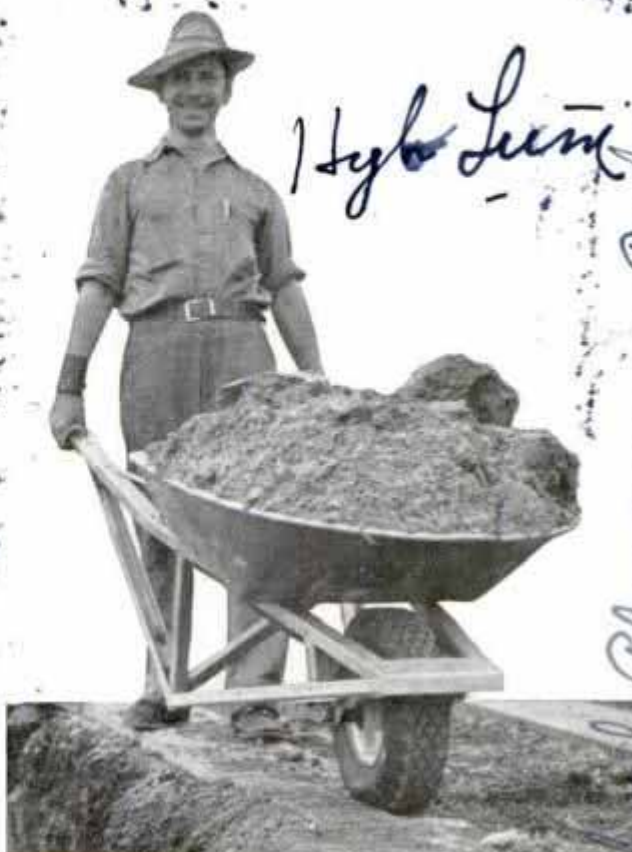
Hyb Lum Heavy pneumatic tire on aluminum wheelbarrow helps balance the load and reduce shock
