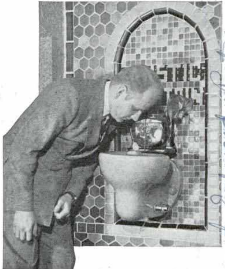
Electricity from body is picked up by antenna in fish bowl, shown near the man's head, causing the fountain to flow
