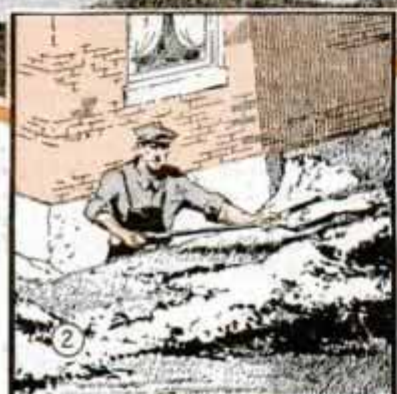
TRENCH IS DUG NEXT TO WALL FOR TILING
