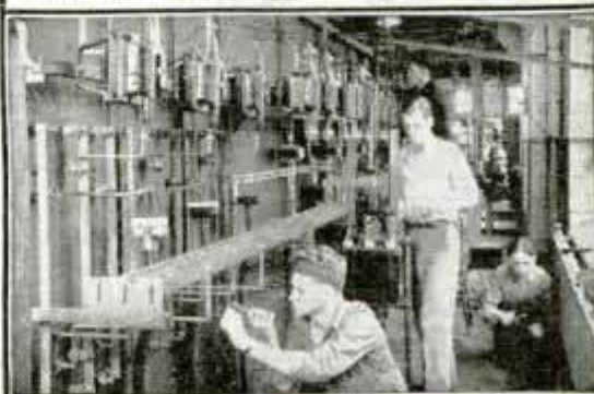
A Real Switchboard in the Coyne Shops
