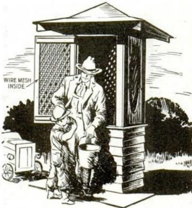
Screen wire tacked over lattice work inside the housing keeps out birds and insects
