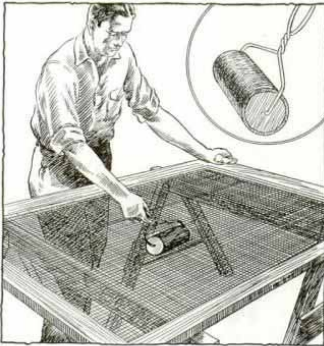
Roller is saturated with paint and then run back and forth over the screen wire
