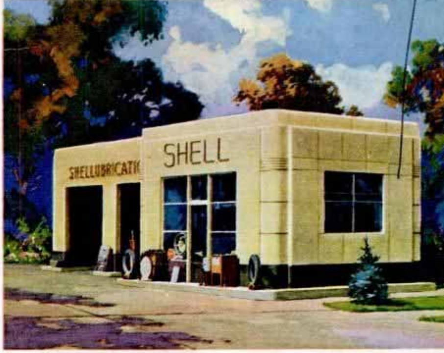
MAIN laboratory room of Chicago Vitreous Enamel Product Company's "Lusterlite Laboratories." Porcelain enameled walls and columns in graduated shades of blue show its possibilities as a building material. Indirect lighting is a feature. Below, filling station of porcelain enameled metal.
