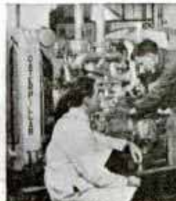
Adjusting Starter on Caterpillar Diesel.
