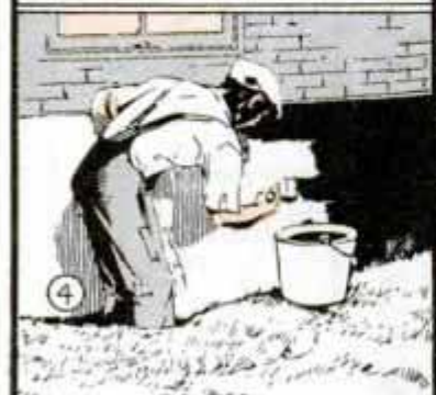
CRACKED AND POROUS CONCRETE WALLS GIVEN TWO COATS OF HOT TAR
