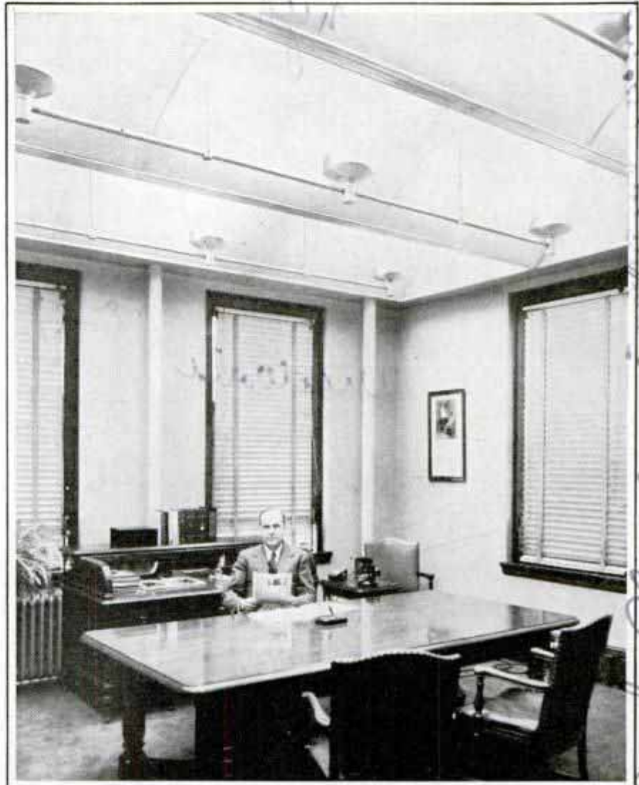
Note fluted or arched sections into which ceiling is divided. This treatment has been found an aid to efficient indirect lighting
