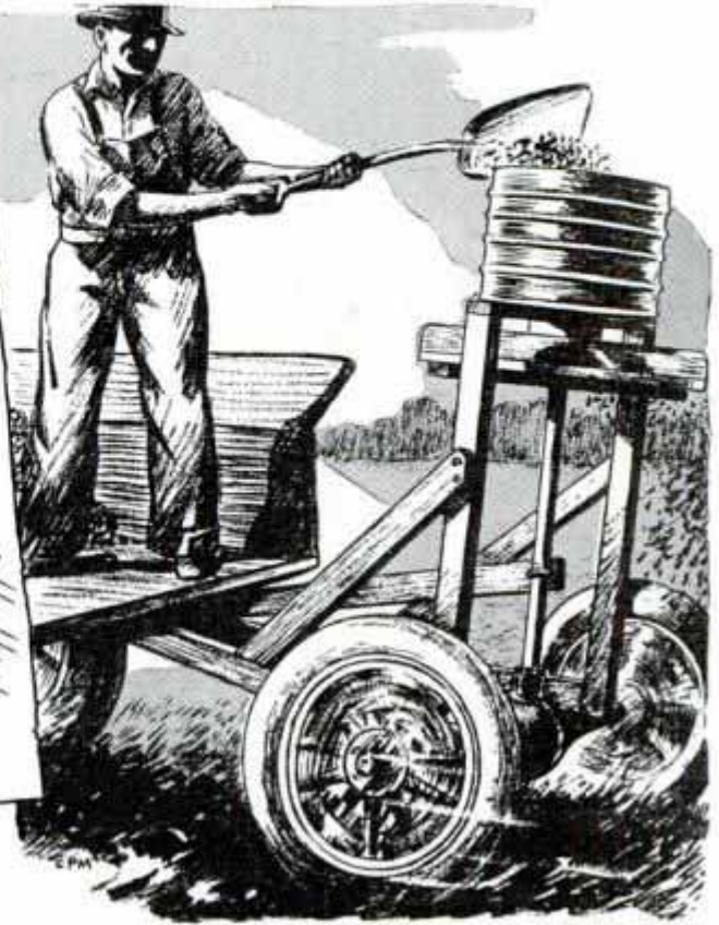
An old rear-axle assembly is about all you need to build this poison-bait spreader
