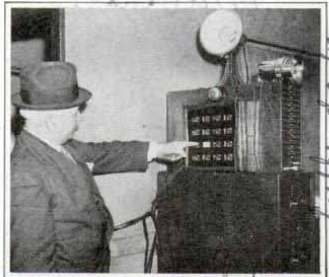
Indicator in warden's office flashes and siren sounds to warn of attempted escape
