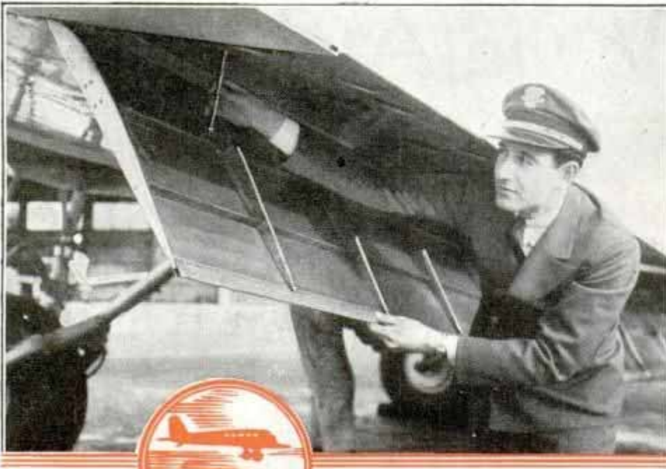
Left, testing air-brake wing flap by which speed of air liner is reduced for landing. Below, inspecting rubber de-icing sleeve on fin of tail group
