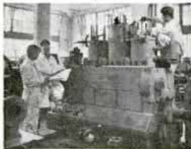
Assembling Enterprise Diesel
