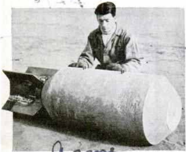
Dummy bomb made of concrete which is used for training army flyers
