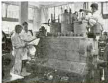
Assembling Enterprise Diesels.
