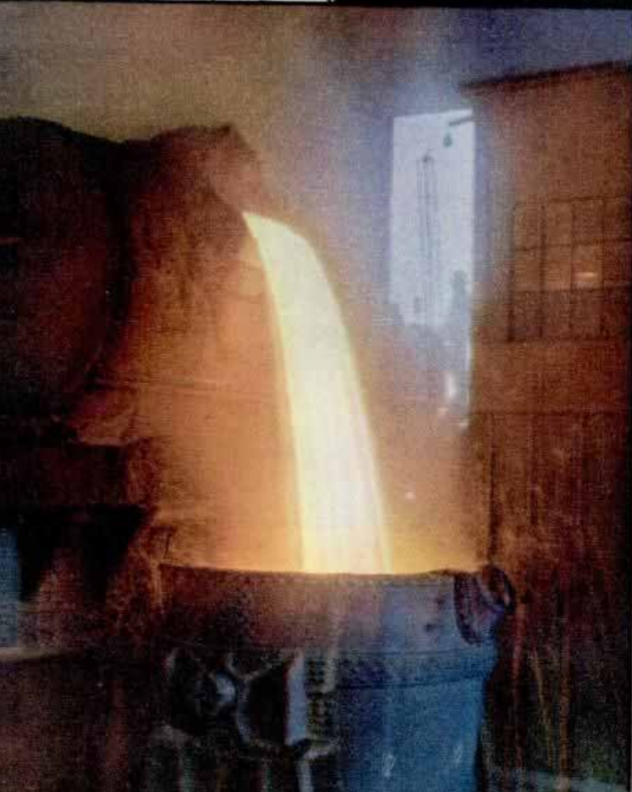
PONDEROUS ingot, above, being passed back and forth through mighty rolls to reduce it to a twenty-foot slab. Left, stream of molten metal spilling into ladle from "hot car."
