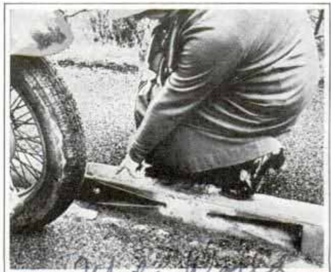
Reflector in each of the V-shaped recesses serves as warning to motorists
