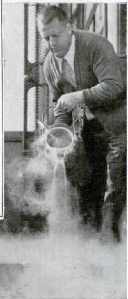
Pouring out a container of liquid air which steams like boiling water
