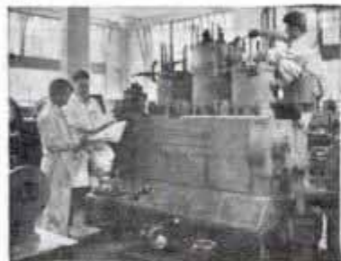
Assembling Enterprise Diesel.
