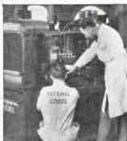
Checking Pump on McCormick-Deering.
