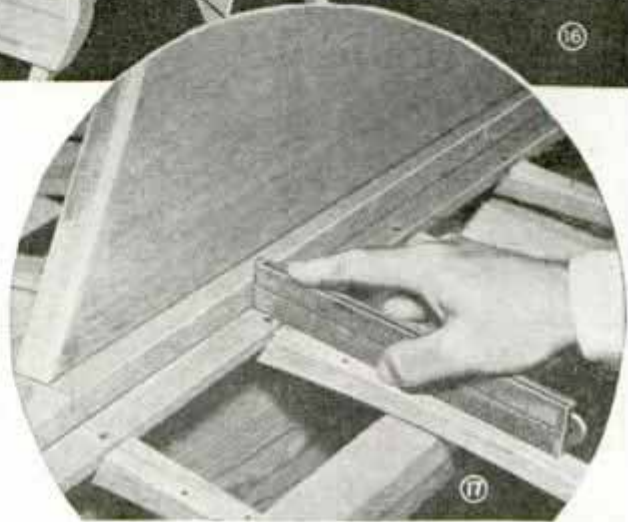
Here's the way you progress with the hull. Above you see the keel, ribs and transom in place and the stem being fitted. Below in Fig. 17 is a very important detail. The bevel of the keelson must coincide with the slope of the filler block so that you get an even bearing for the plank
