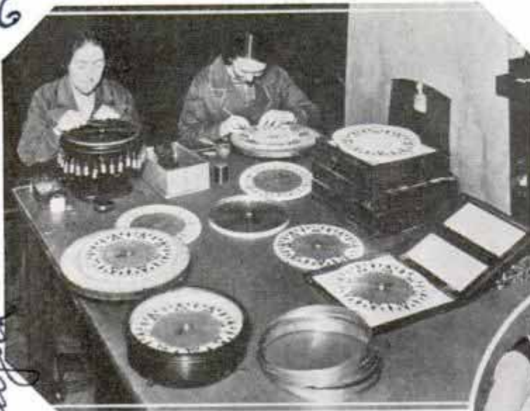
Stitching compass points on silk. Right, finishing shockproof pedestal for "Queen Mary's" compass
