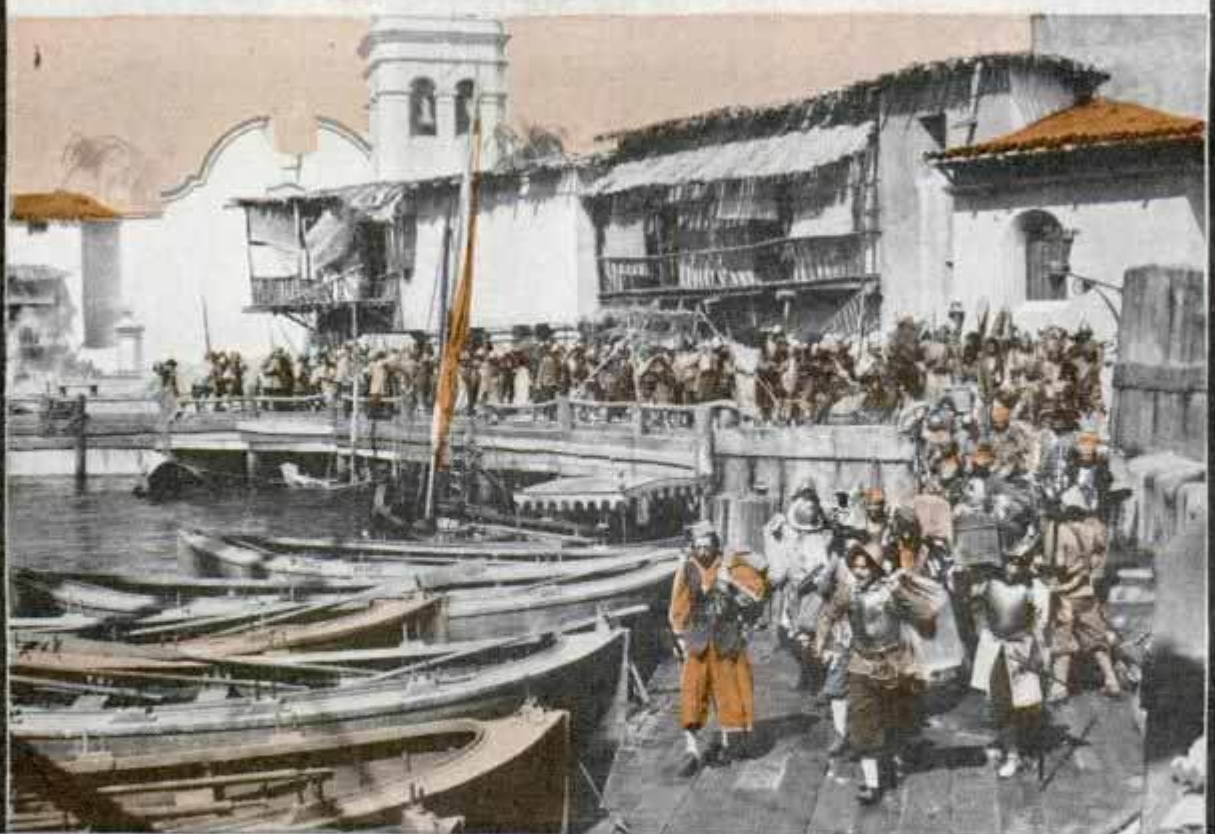
Two views of a sea-coast town built on a back lot in Hollywood for a recent production. The boats rest in real water which fills the concrete basin
