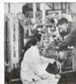
Adjusting Starter on Caterpillar Diesel.
