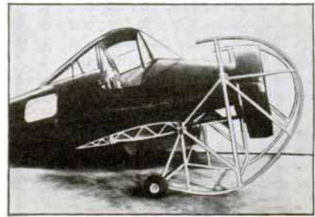
Metal "cage" around nose of plane allows pilot to somersault on field in testing new cabin designs
