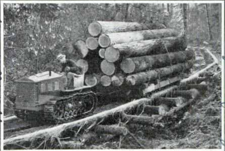
Wood railway with poles serving as rails used in logging operations. The wheels of the log car are grooved to fit the poles
