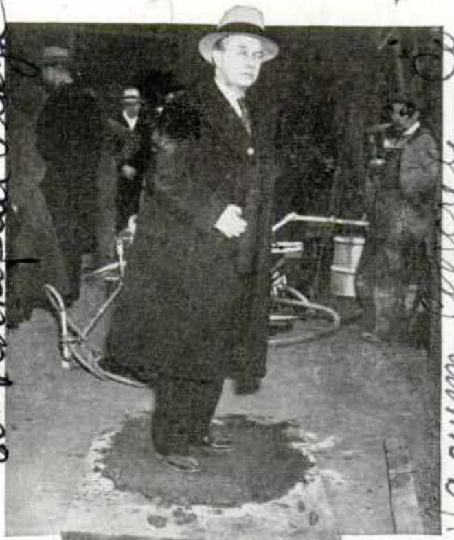
Standing on concrete dried by new process
