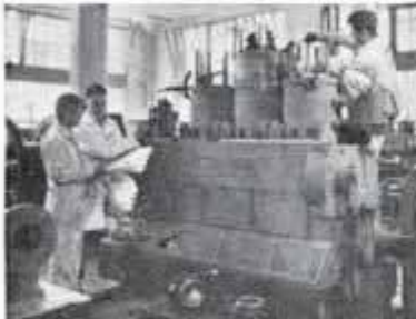
Assembling Enterprise Diesel.
