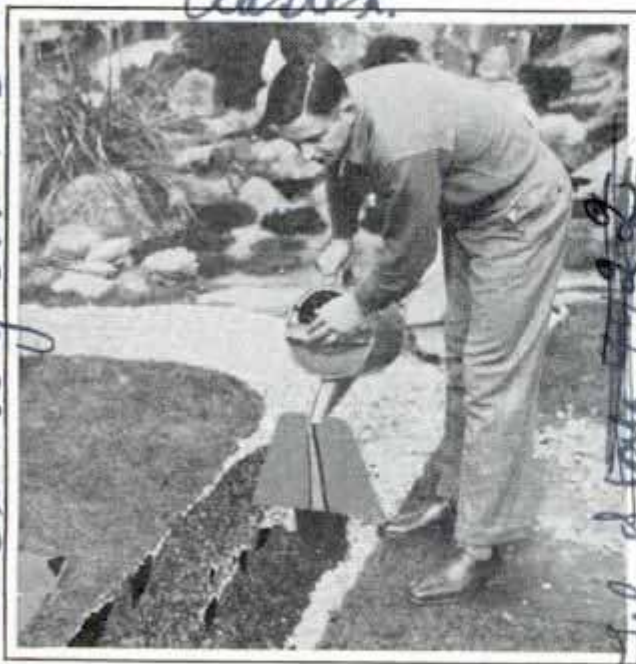
It takes no special equipment or skill to pave your garden path by pouring cold asphalt
