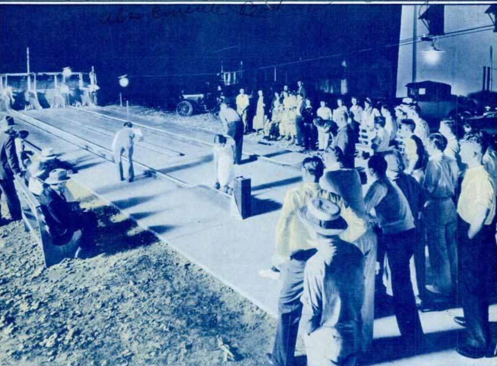
CONCRETE has brought bowling out-of-doors, as evidenced by this night scene on alley of man-made stone at Miami, Fla.
