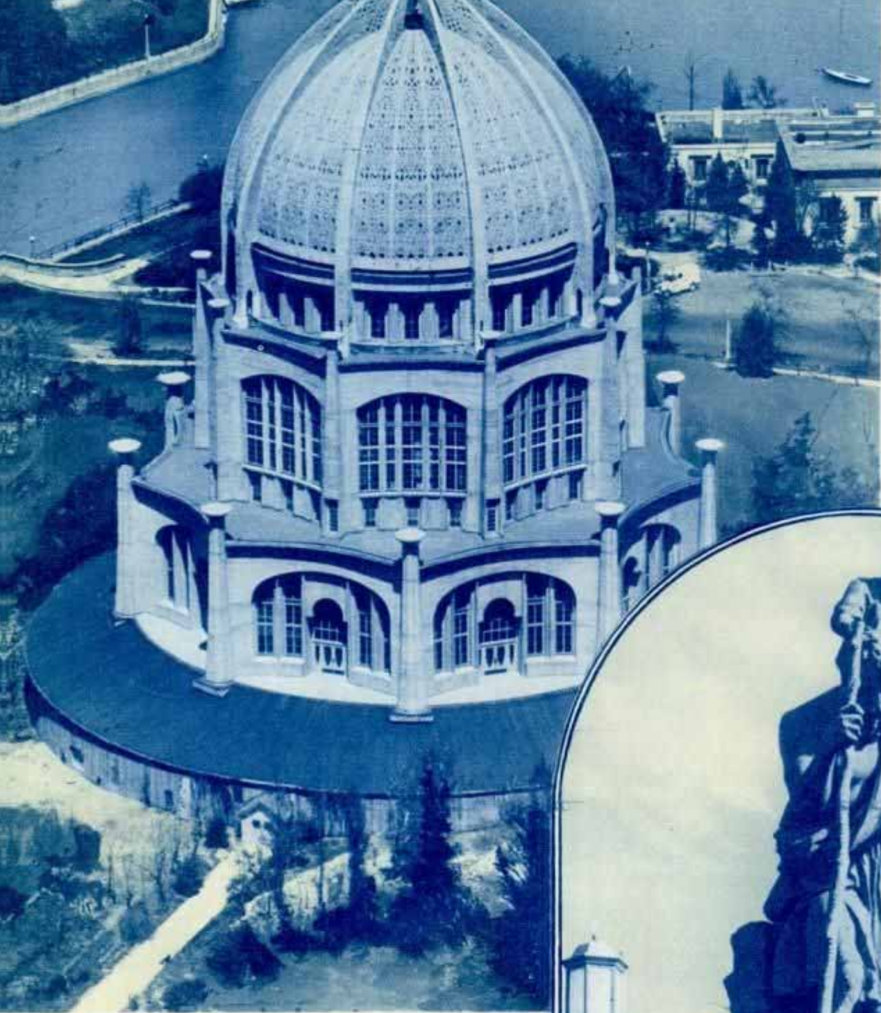
Bahai THE BEAUTIFUL Temple of Light near Chicago whose tough, rugged sinews of concrete, jeweled with crystal-like frag- ments of quartz, are so delicately molded as to give the appearance of a piece of fine lace, as can be noted on the dome. The entire structure, out- side and inside, eventually will have the same appearance as the dome. Right, note how the lines of nature have been reproduced in concrete in this statue of St. Christopher.
