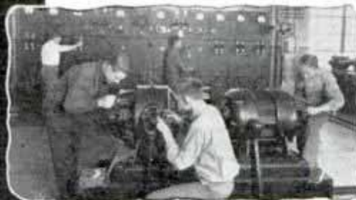
Students repairing motor generator set, and operating one of our power switchboards.
