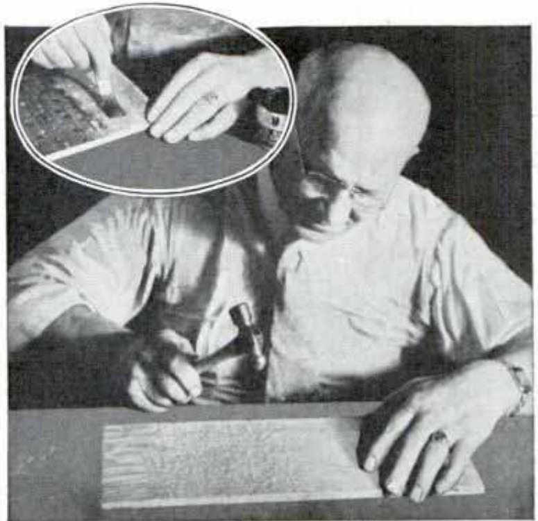
Dented wood given coats of shellac, aluminum bronze powder and black paint has appearance of hammered metal
