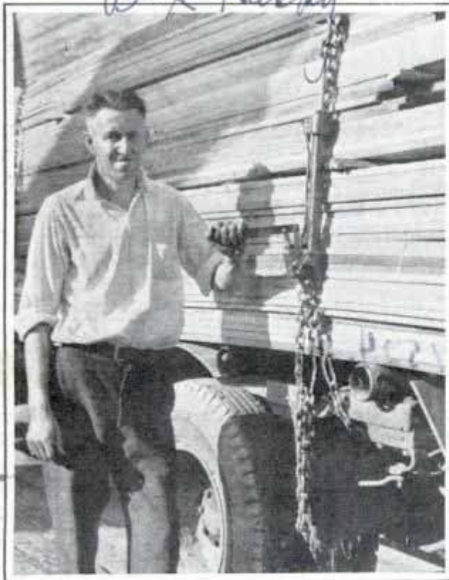
Handy hydraulic hoist shown in place, ready to lift loads up to one and one-half tons
