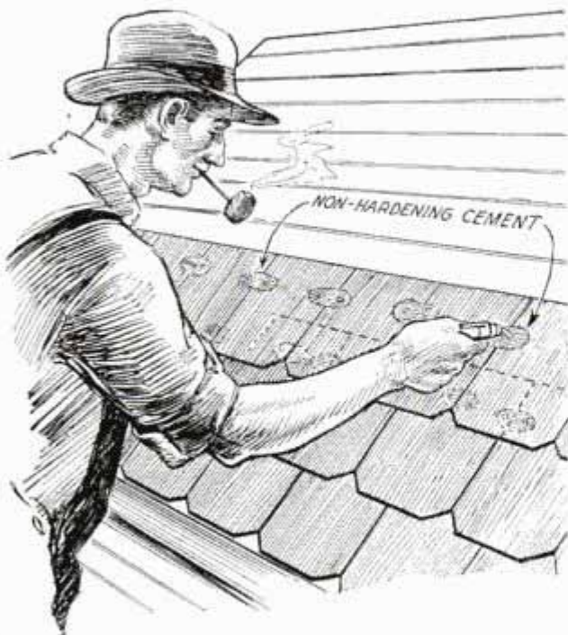
Cement protects nail heads in slate roof against corrosion which allows wind to loosen shingles
