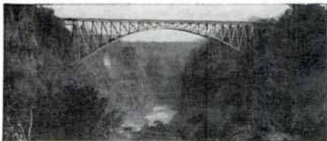
Steel Arch Bridge, Victoria Falls, Africa.
