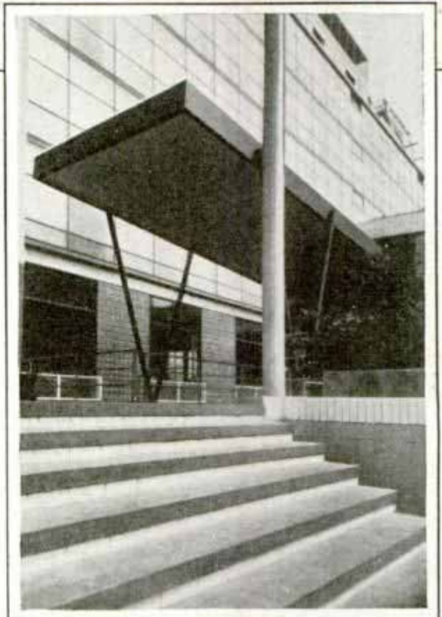
Raised Foundation for Paris Dormitory and Salvation Army Building in Paris
