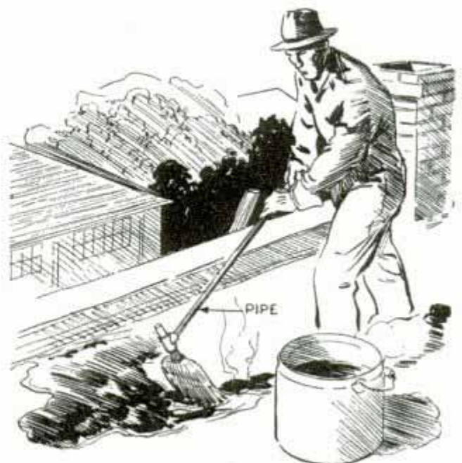
Interchangeable Handle Made of Pipe to Utilize Old Brooms for Spreading Tar on Roofs
