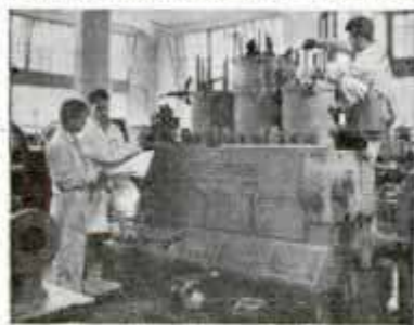
Assembling Enterprise Diesel.
