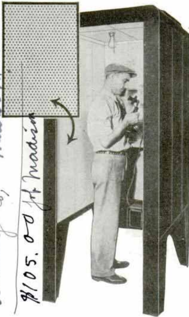
Walls of Perforated Metal Backed by Balsam Wool Absorb Noise and Make Doors Unnecessary
