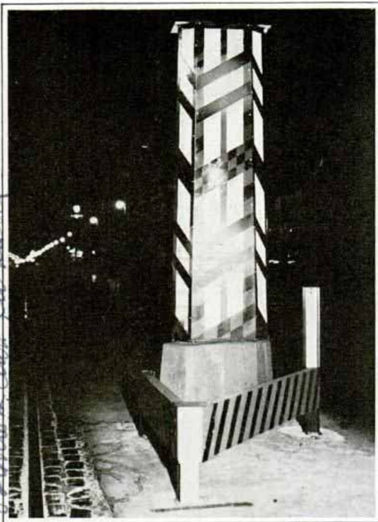
This Illuminated Safety-Island Guard Is Visible for Long Distances; It Is Equipped with Non-Glare Sodium Lamp
