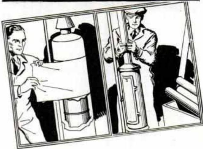
Insulate the Tank to Keep Water Hot as Long as Possible; Non-Corrosive Vent Pipe on Water Heater Will Outlast Many Common Ones
