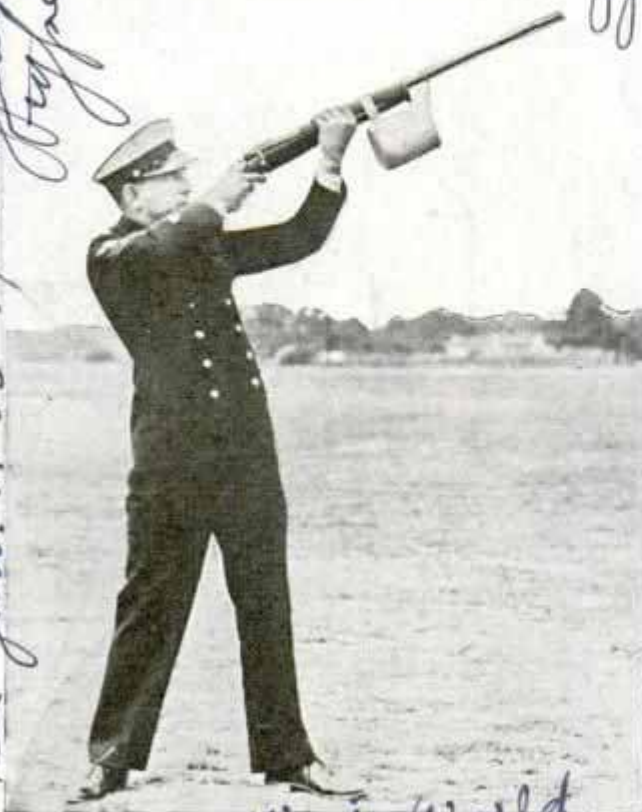
Wide World. Rifle Used Instead of Cannon by Coast Guard for Firing Line from Shore to Ship
