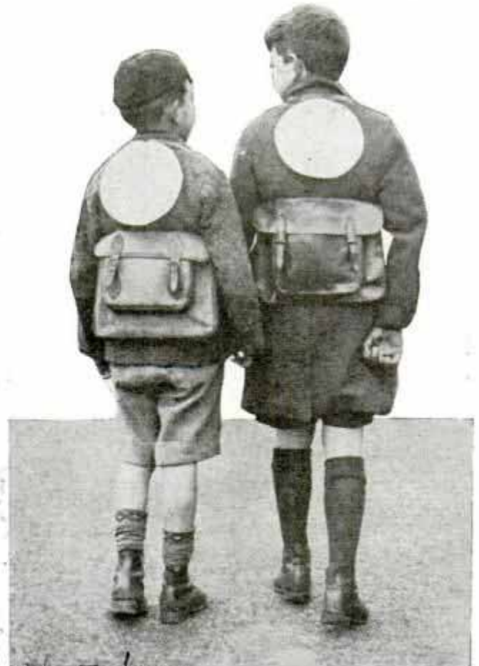
These White Disks Reflect Auto's Light and Protect Children on Dark Roads
