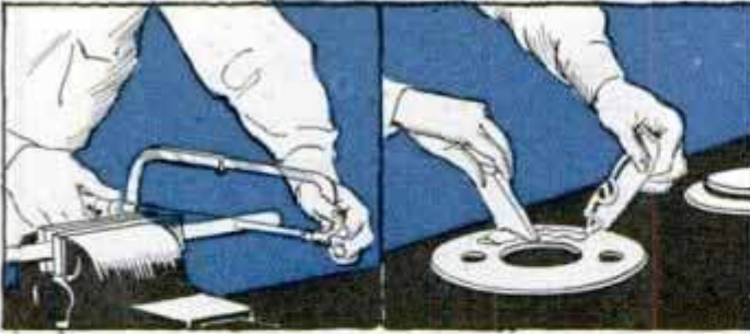
Tubing Must Be Cut Off Squarely to Size; Right, Cementing Aluminum to Wood with "Liquid Solder"
