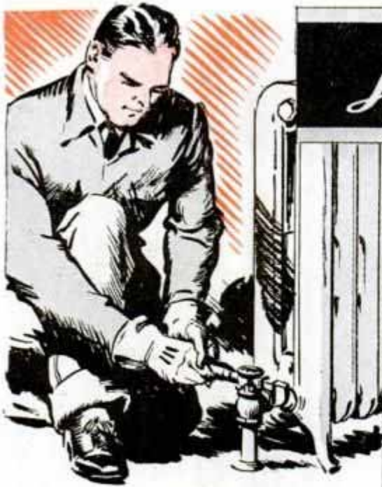
Radiator Valves Should Be Well Packed to Prevent Escape of Steam or Hot Water, Which Necessitates Adding "Raw" Water to Boiler
