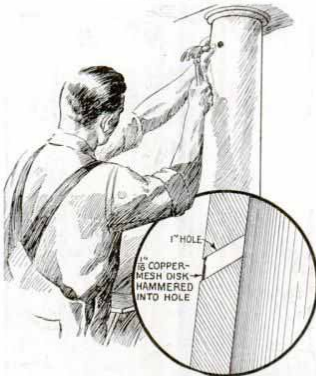
Holes Drilled in Porch Columns Allow Air to Circulate Through Them and Prevent Decay
