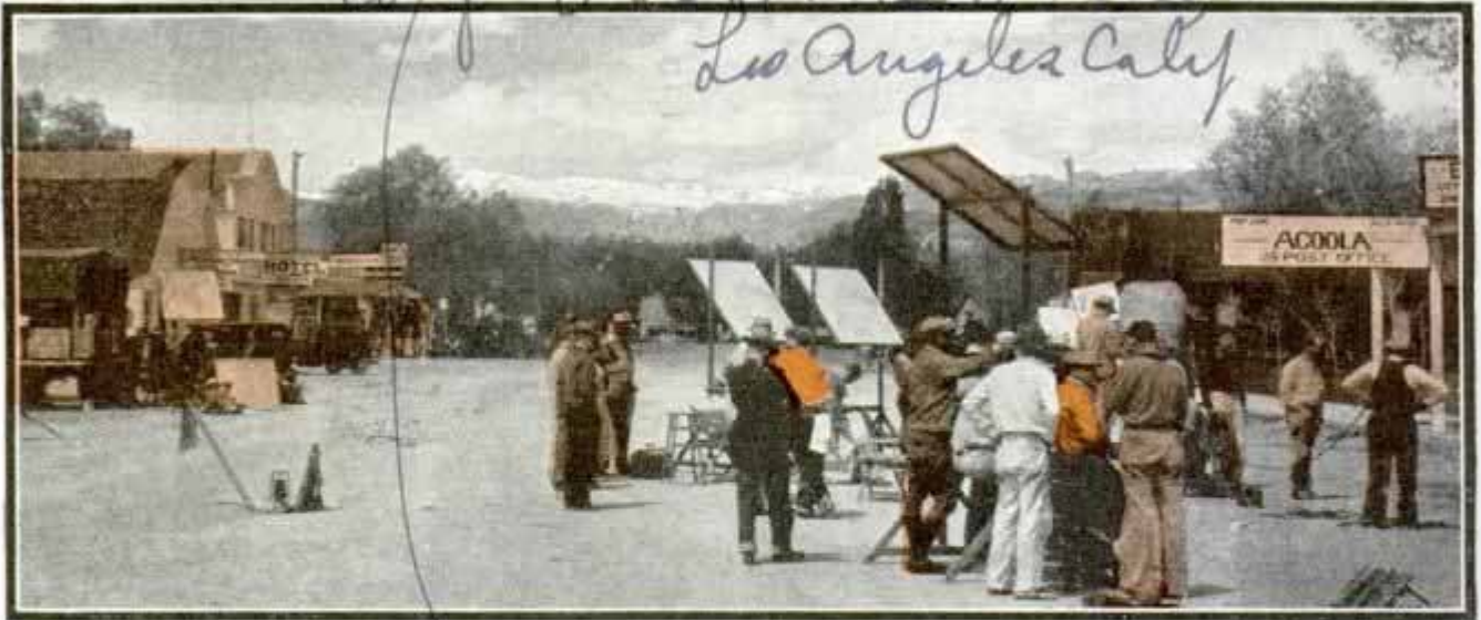
Fox Company on Location at the Little Town of Bridgeport, Calif., 8,500 Feet Up in the High Sierras
