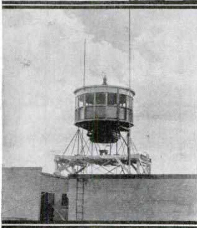
Top, High-Speed Camera with Twelve Lenses to Photograph Lightning from Tower, Shown Below
