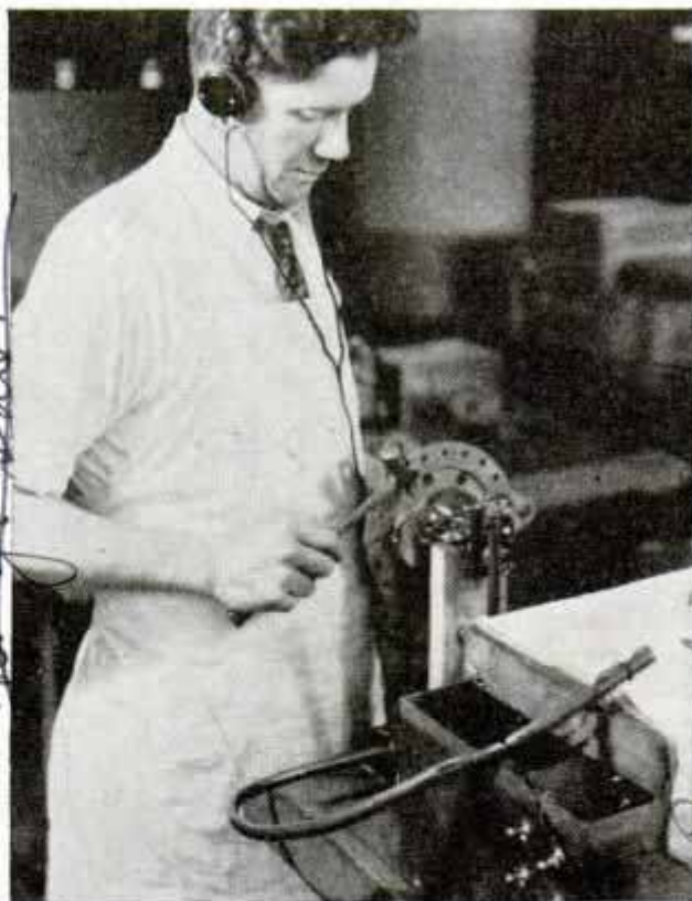
Sound Tests of Refrigerator Cylinder by Radio Receiver Reveal Hidden Defects
