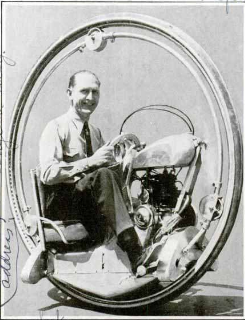
Builder with His Odd-Looking Vehicle That Runs on One Wheel; Note Small Motor Used for Propulsion
