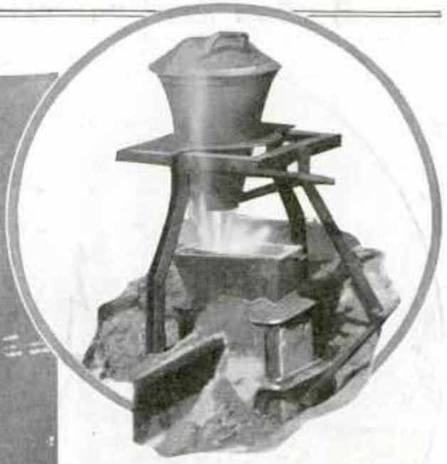
Above, Molten Steel Pouring from Crucible into Mold around End of Rails, Thermit-Welding Them into Solid Ribbon of Steel; Left, Thermit Weld Was Used to Repair Breaks in This: Huge Casting, Twenty-Two Feet High and Fifteen Feet Wide
