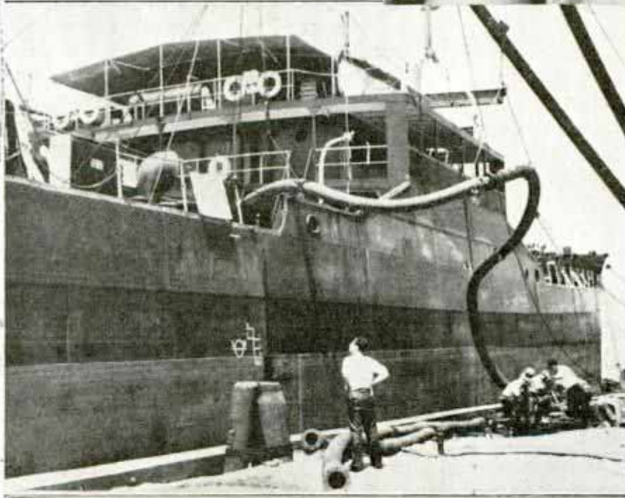
Left, Tanker Unloading Petroleum at Mammoth Oil Port in New York City That Has Facilities for Accommodating Hundreds of Craft Annually; Above, Part of Terminal's Extensive Pipe-Line System
