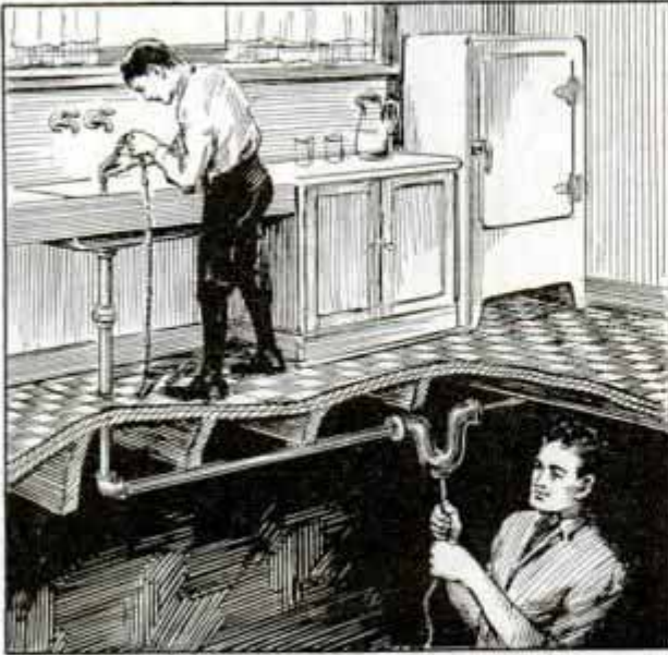
Old Piece of Chain Used to Clean Out Drain Pipe, Which Ran Horizontally under the Floor
