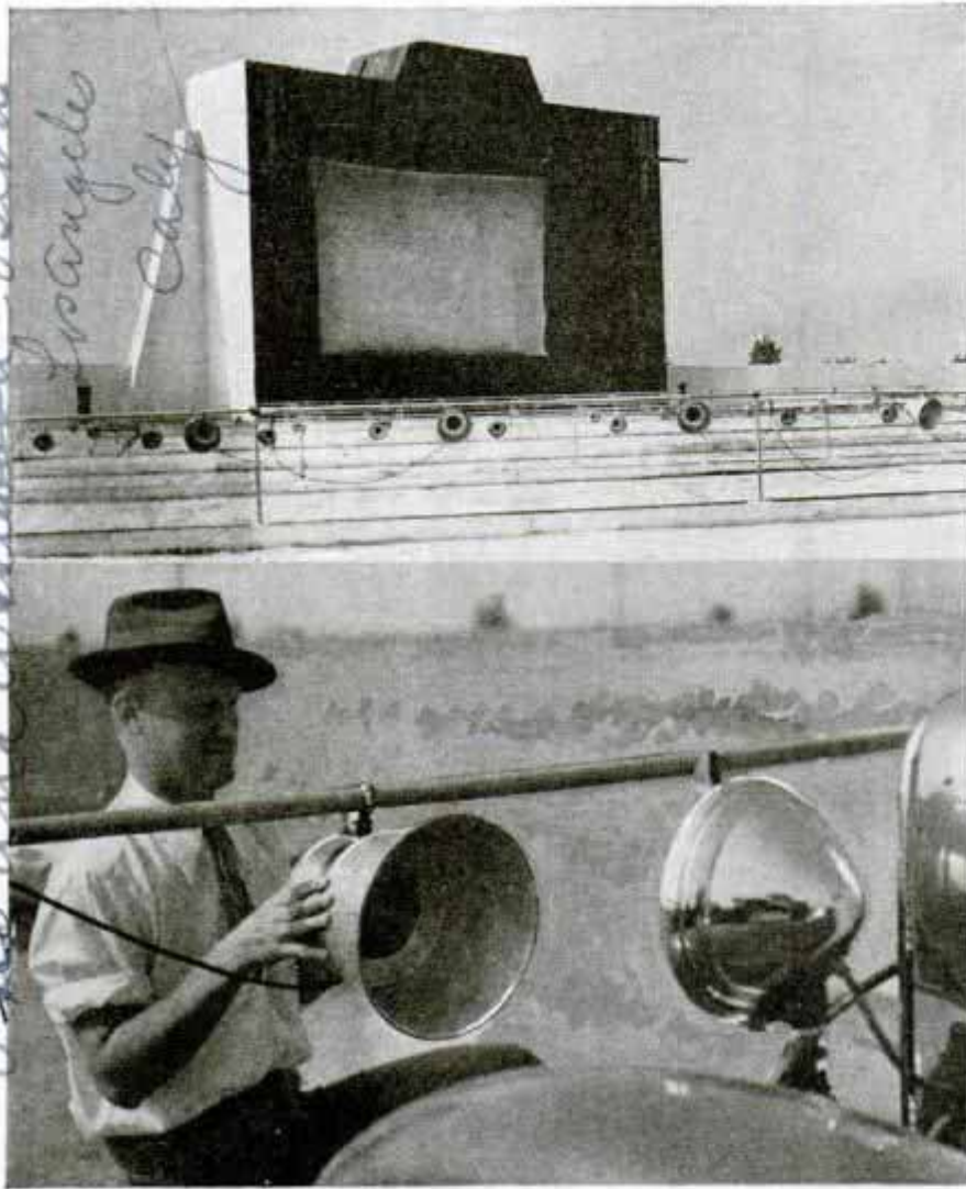
Top, Screen 2,000 Square Feet in Area at Drive-In Theater; Below, Bucket-Shaped Individual Speakers Attached to Railings in Front of Parking Rows Bring Sound to Each Car
