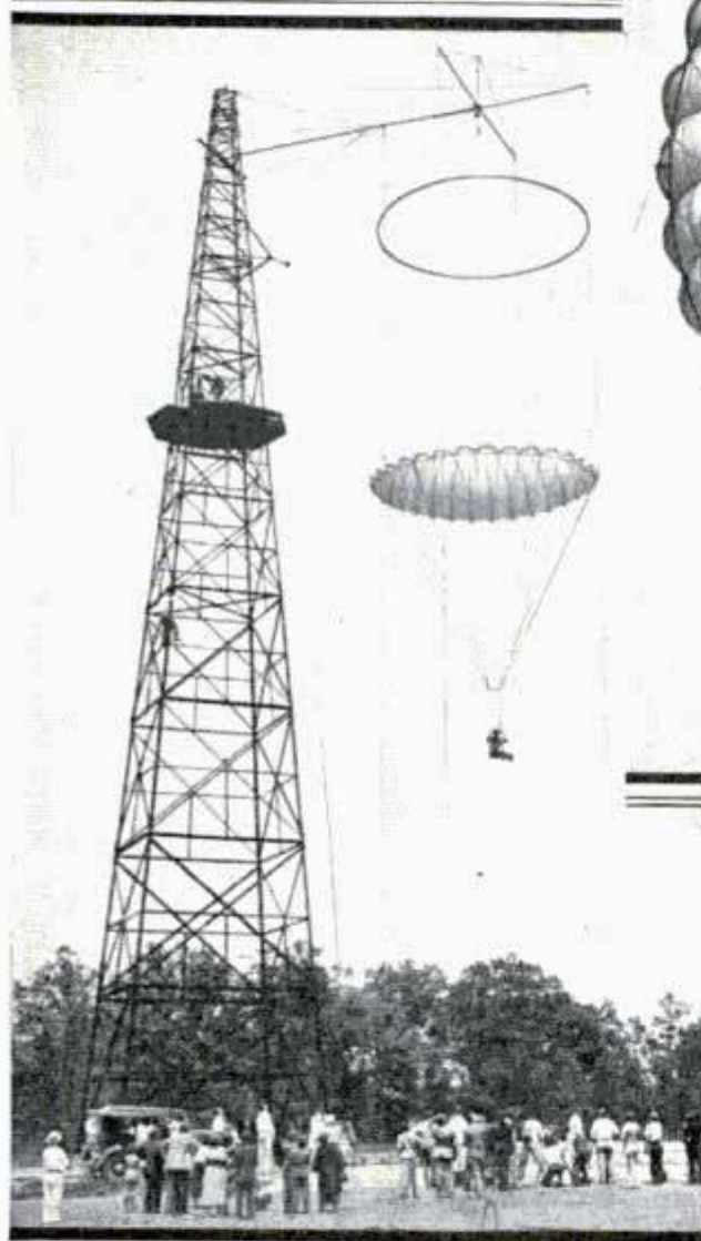
Left, Student Makes Practice Jump after Being Hauled Up by Cable; Right, Closeup of Parachute
