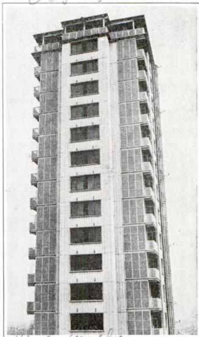
Sixteen-Story Apartment House Skyscraper in Paris Suburb Built of Steel Units and Cement
