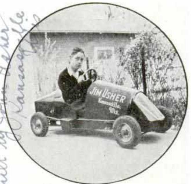
Automobile Starting Motor Operating on Two Six-Volt Batteries Drives This Tiny Car
