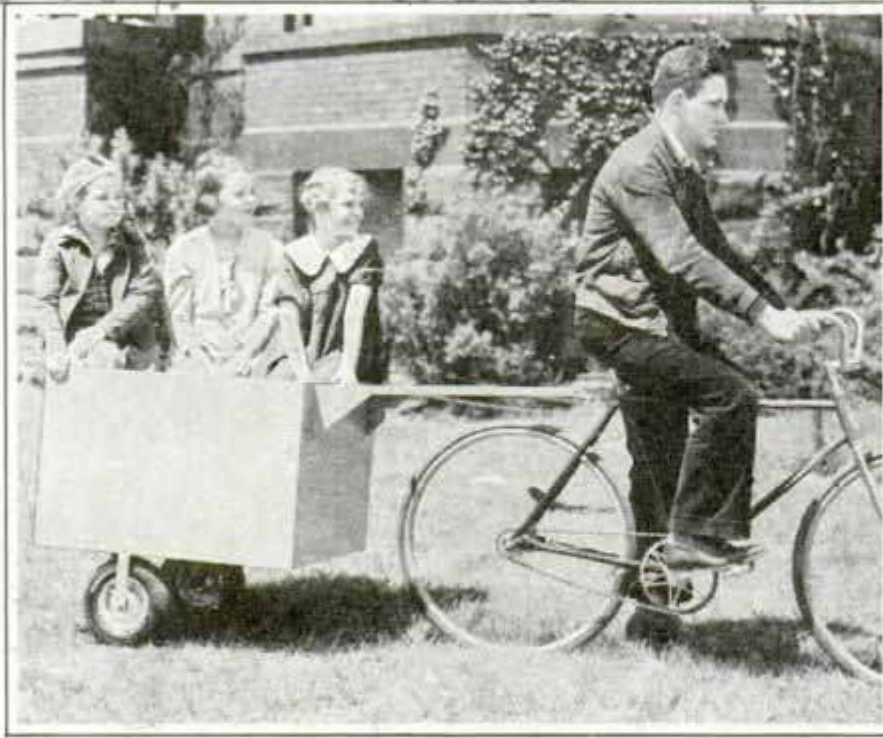
Passengers or Freight Ride Smoothly in This All-Steel Trailer, Two Feet Wide and Thirty Inches Long, Easily Towed by Bicyclist
