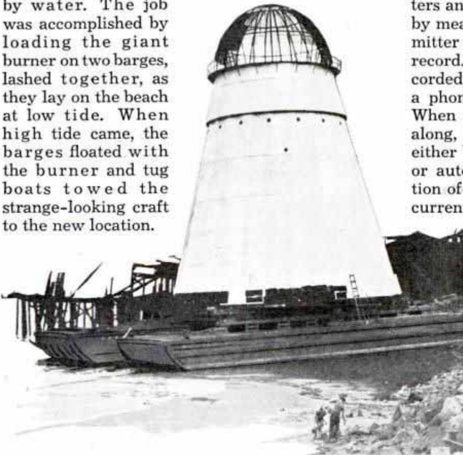
Showing Eighty-Foot Refuse Burner on Barges Which Transported It to New Location; Loading Was Accomplished at Low Tide
