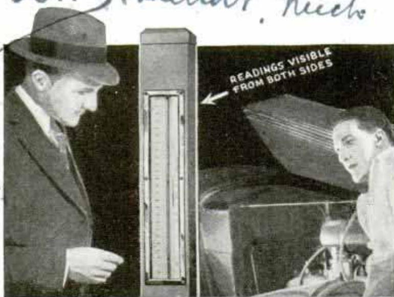
Customer and Mechanic Watch Mercury Column as Tester Is Applied to Various Parts of Auto Engine
