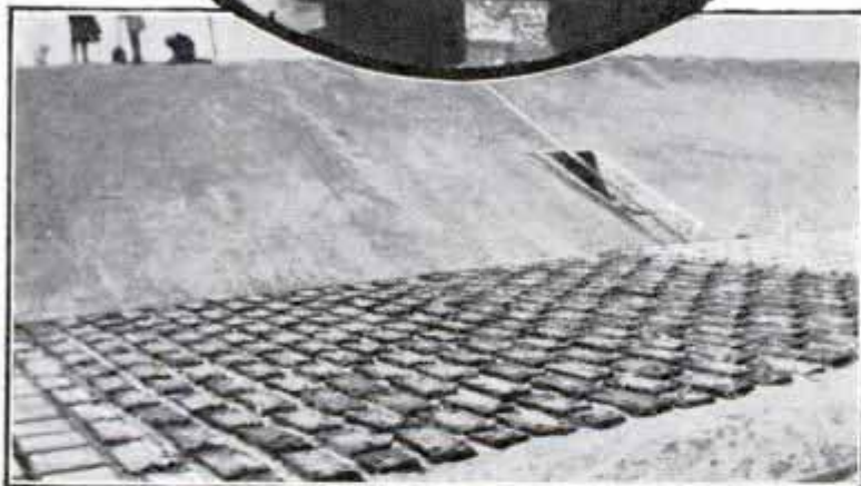
Top and Center, Right, Bullet-Proof Shelters Constructed of Tin-Can Blocks; Center, Left, Mechanical Conveyor Used for Stacking and Unstacking the Blocks; Bottom, Showing How the Metal Bales Were Placed on River Bed to Prevent Current from Undercutting the Banks
