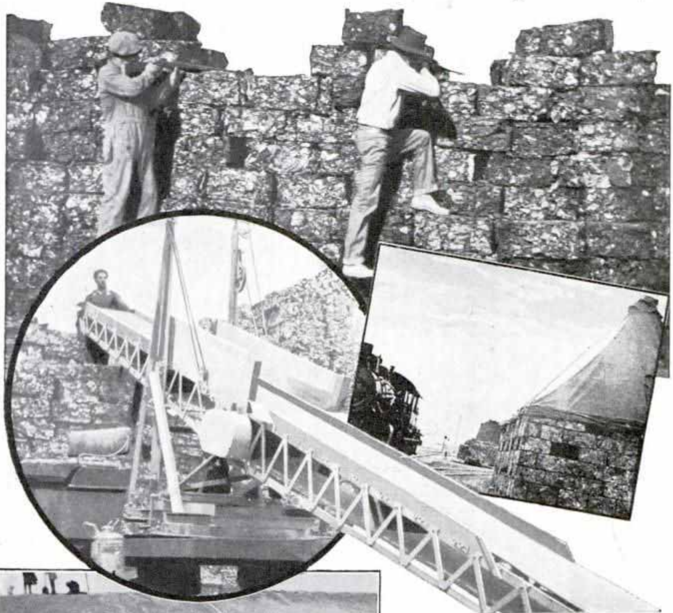
Top and Center, Right, Bullet-Proof Shelters Constructed of Tin-Can Blocks; Center, Left, Mechanical Conveyor Used for Stacking and Unstacking the Blocks; Bottom, Showing How the Metal Bales Were Placed on River Bed to Prevent Current from Undercutting the Banks
