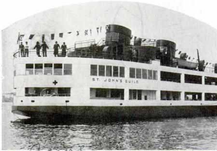
This Mercy Ship Will Transport Poor Children on Outings; Note How Second Deck Is Enclosed with Glass
