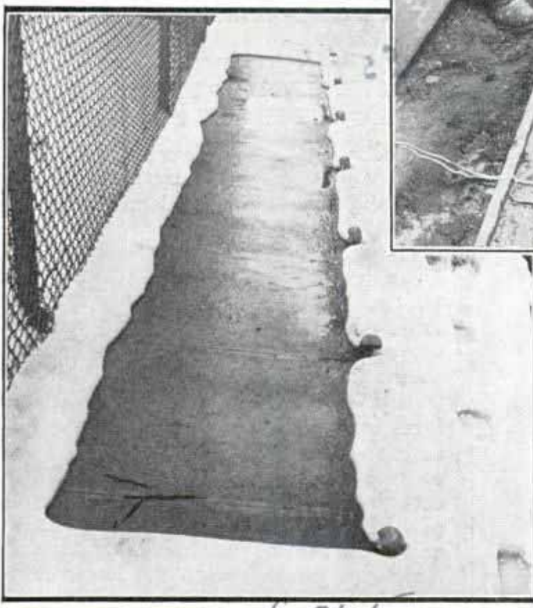
Cement Is Being Spread over Specially Coated Electric Cables in Sidewalk at Right; When Current Is Switched on, Heat Generated in Wires Melts Snow
