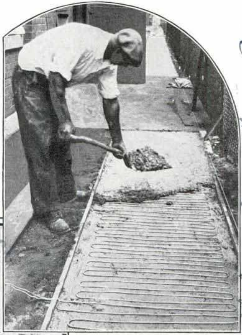
Cement Is Being Spread over Specially Coated Electric Cables in Sidewalk at Right; When Current Is Switched on, Heat Generated in Wires Melts Snow
