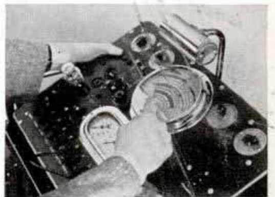
Master Meter indicates condition of radio tubes.
