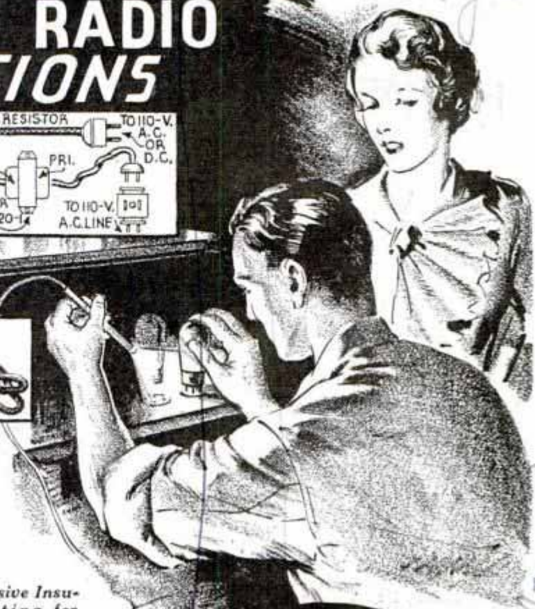
Homemade Probing Light for Working in Dark Corners; Construction Details for Two Varieties Are Given Above; the Multiple Plug Permits Operation of Set and Light from the Same Wall Socket
