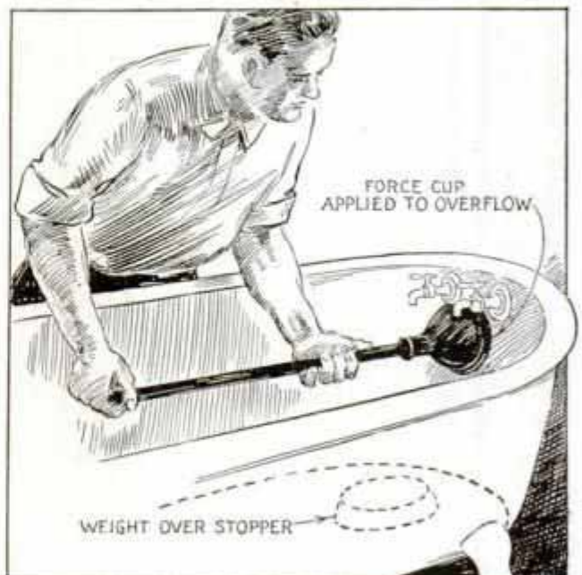
Bathtub Drain Cleaned by Using Plumbers' Force Cup at Overflow Opening
