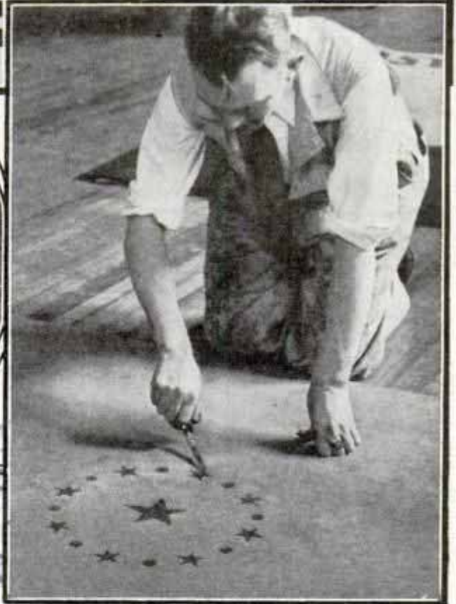
Three Steps in Preparing Latest Carpet for Inlays; Process Simplifies Decorative Work
