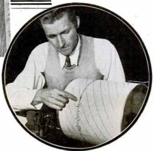
Jagged Lines Recording Earthquake, and Measuring a Distance Taken from Seismogram Records to Learn Location of Temblor
