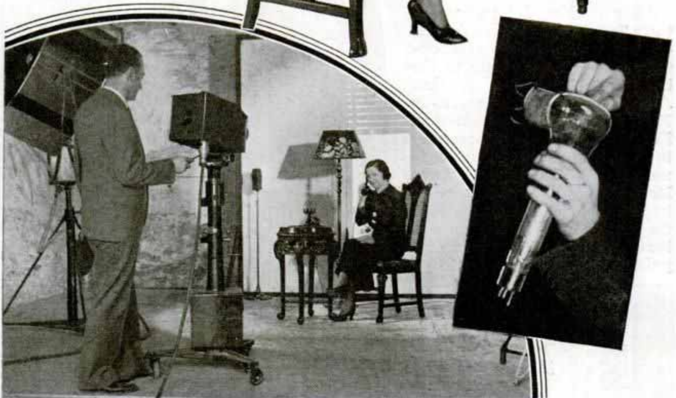
Above, Tuning in Television Receiving Set; Camera and Lighting Arrangements in Broadcasting Studio Are Shown Below; Right, Tube Which Projects Image upon Screen
