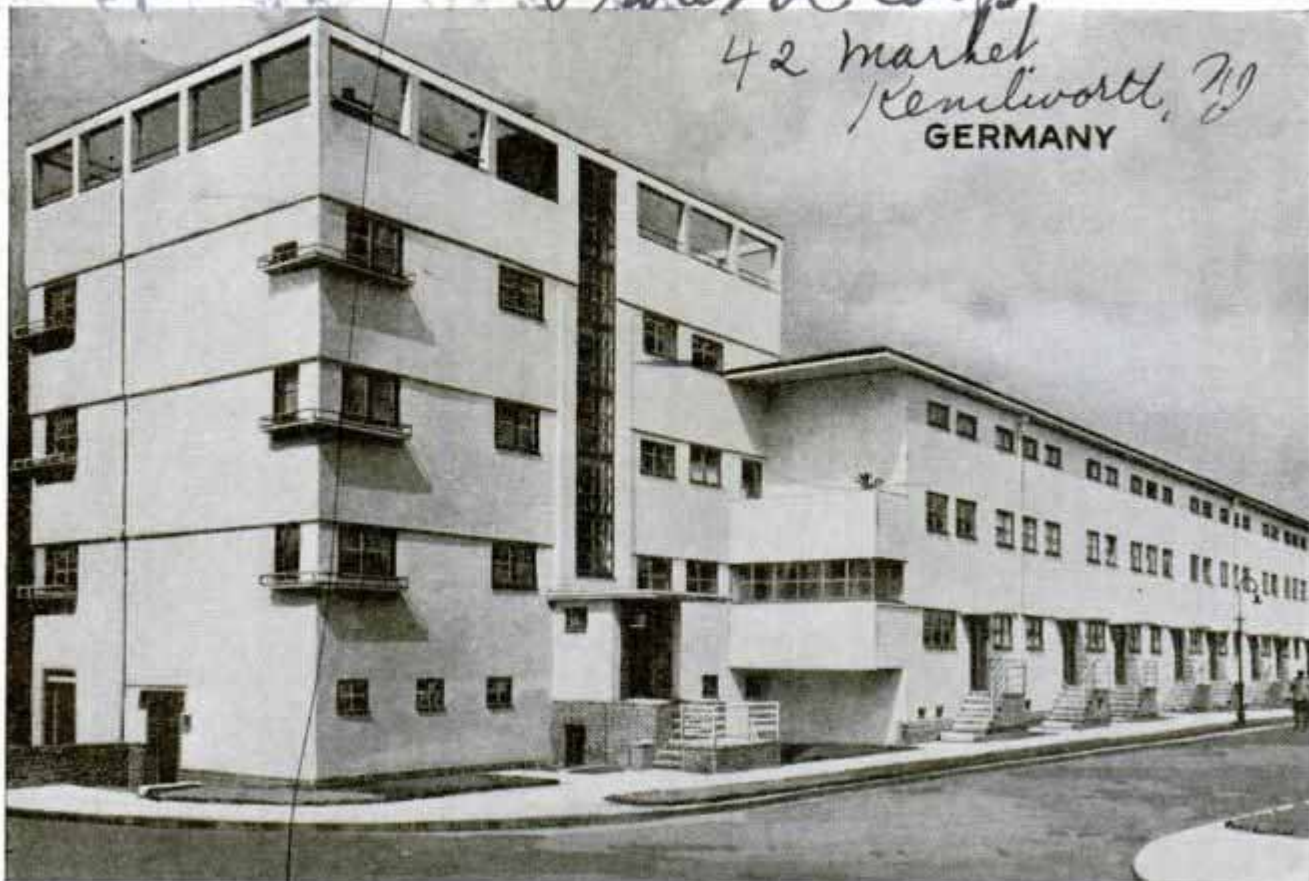
Flats for Workers as Provided in Germany Today; Note the Plain Surfaces, the Glass-Enclosed Top Story and the Little Balconies at the Corners
