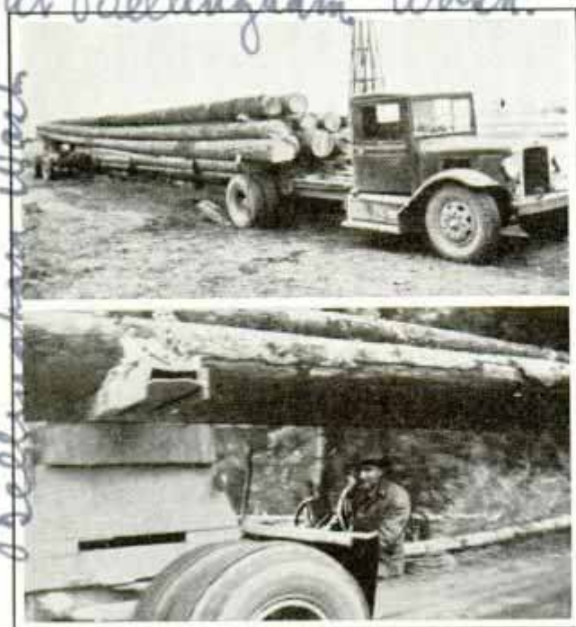
Top, Truck and Big Log Trailer; Bottom, Rear End Steering for Turning Curves
