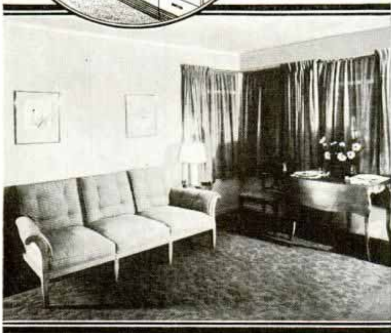
Top, Another Model of the Mechanical Home, with Two Stories, Sun Deck and Double-Car Garage; Center, Sketch of Conveniently Arranged Kitchen; Bottom, the Living Room of One of the Mechanical Homes
