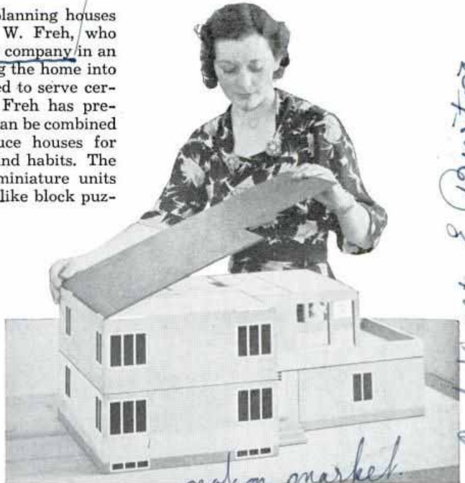
Model House Put Together in Units, with the Roof Being Lowered into Place; the Model Demonstrates a New Idea in Building Practice
