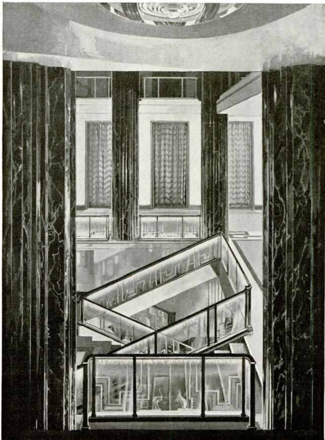
Main Staircase Hall of New Building of Royal Institute of British Architects, Showing Etched-Glass Stair Rails, Illuminated by Tubular Lights Concealed in the String
