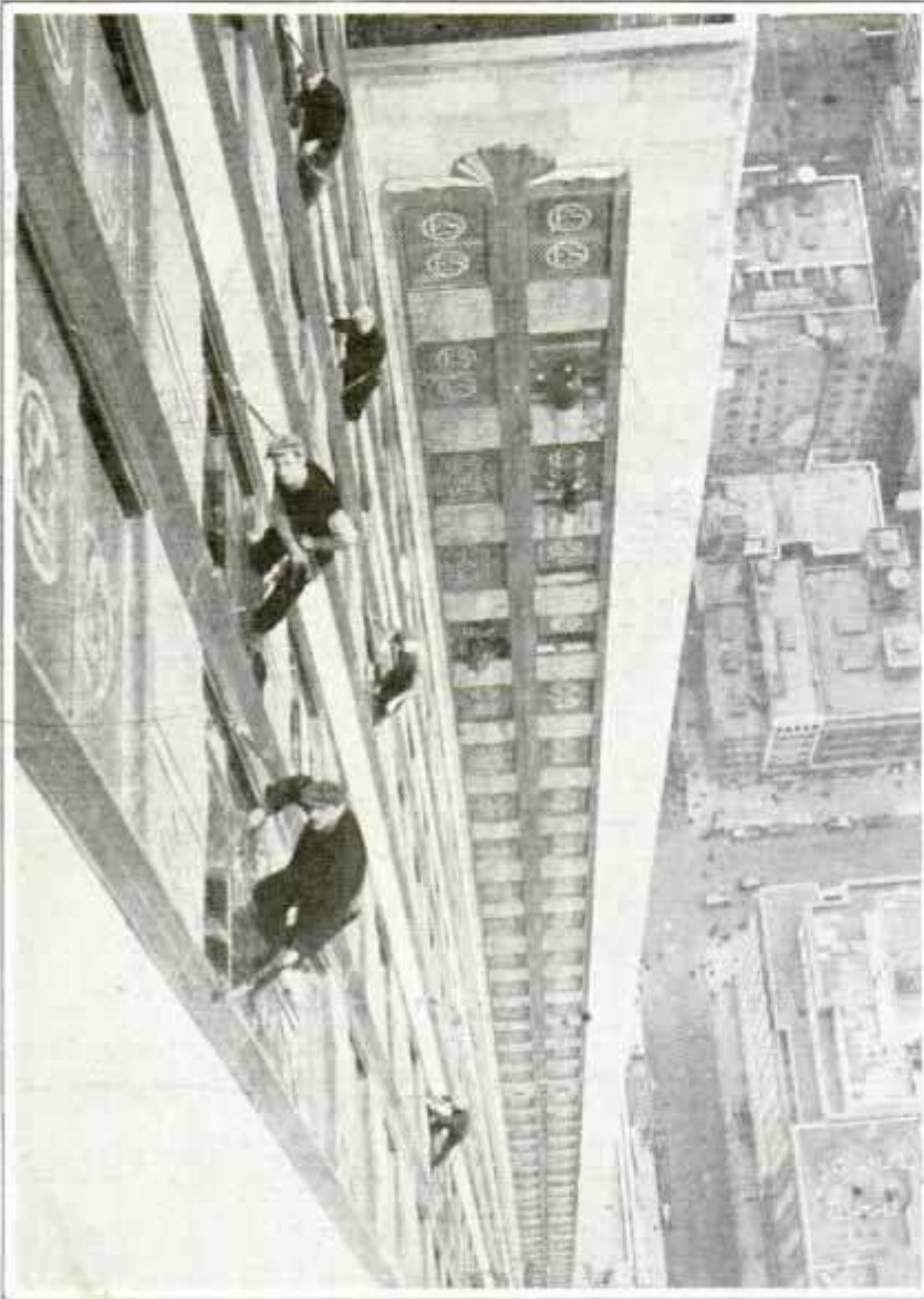
Window Washers at Work Near the Top of a Lofty Skyscraper; Note Safety Belts Attached to Lugs in Sides of Windows
