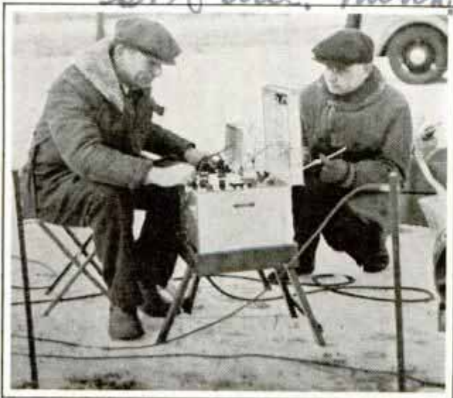
Sensitive Equipment Indicates Formation Below Surface; It Is Shown in Use
