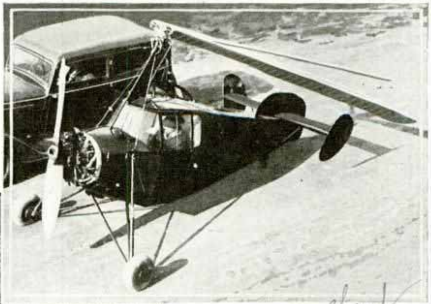
clm Showing How Rotor Blades Can Be Folded for Taxiing Like Auto
