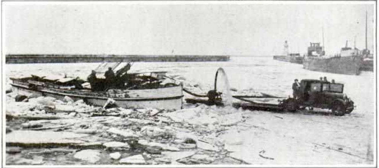
Auto Is Shown Pumping Water from Sinking Boat; Note the Pump Located between the Car and the Boat; This Unusual Means of Salvage Saved the Boat after Ice Had Punctured a Hole in Its Hull
