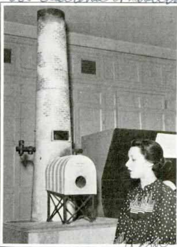
Model of Photo Cell in Chimney
