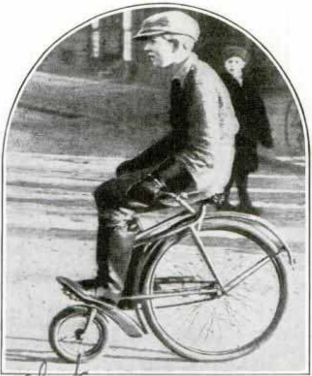
Int. Bicycle with Small Front Wheel Which Is Steered with Single Handle and Pedaled in Usual Manner
