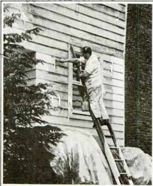
Removing Old Paint with a Paste Which Is Applied with a Brush and Then Peeled Off
