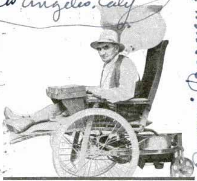
Motorized Wheel Chair for Invalid Operated by Two Levers, One for Steering and One for Accelerating
