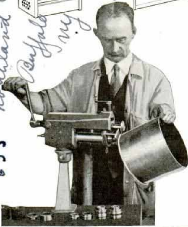
Seams and Joints in Sheet-Metal Work Are Readily Formed with Small, Commercial Outfits, Which Can Be Purchased, and Come Equipped with a Number of Attachments
