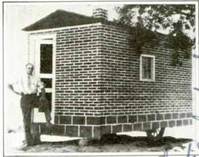
Traveling Home in Which College Student Lives; the Wood Is Painted to Resemble Brick
