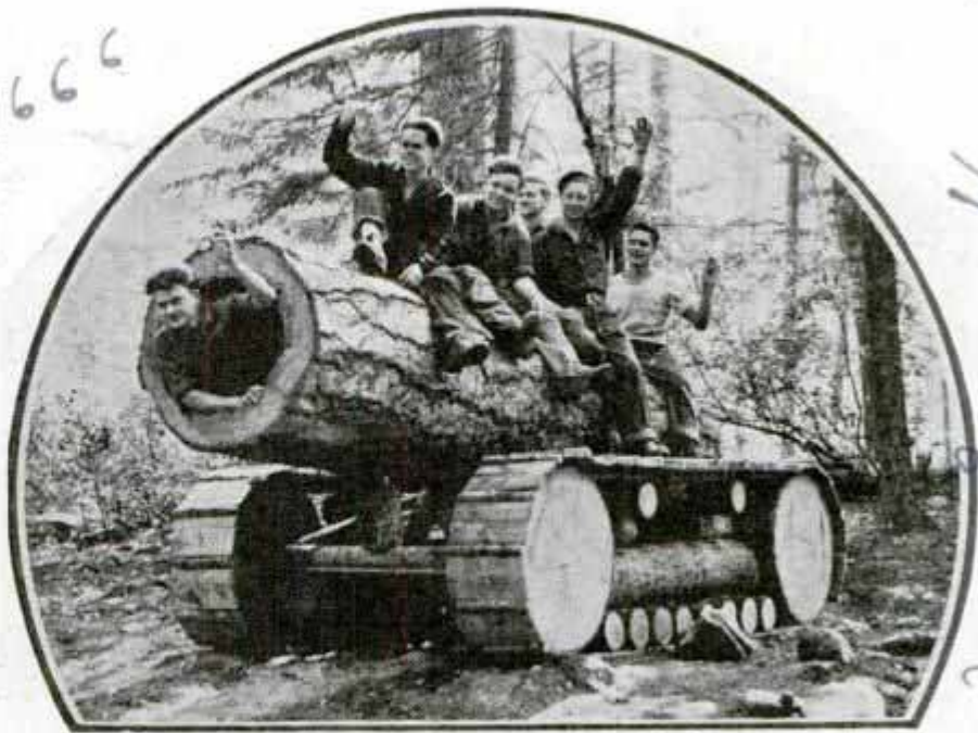
This Is a Wooden Gun, But It Is Too Large to Be Called a Toy; the "Big Bertha" Is Made of Logs and Is Mounted on a Log Tractor
