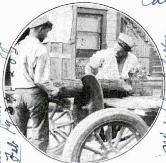
Circular Saw Being Operated from Truck Differential
