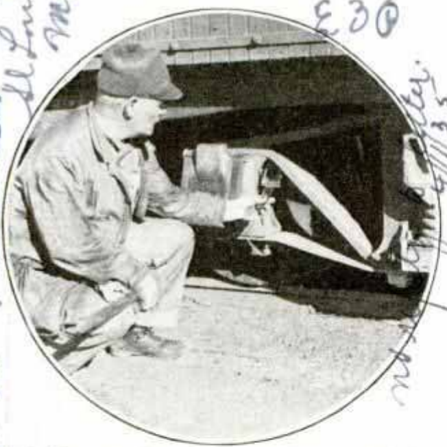
Car Inspector Using Mirror to Examine Arch Bar
