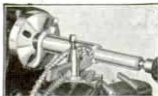
Turning Down a Steel Bar.
