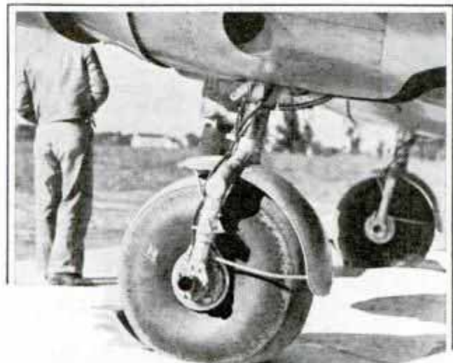
These Mudguards Protect Plane's Retractable Landing Gear from Flying Mud and Gravel
