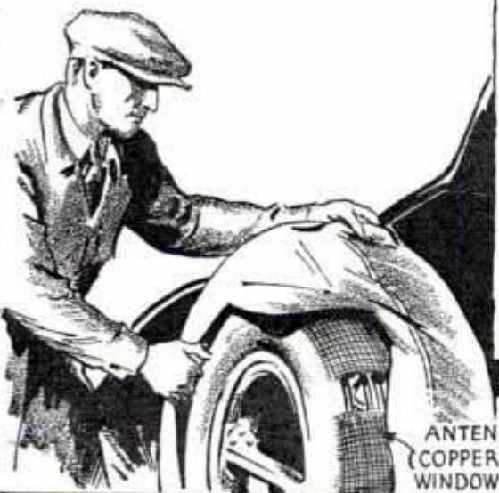
Below, Strip of Copper Screen under Fabric Tire Cover on Spare Tire, Makes Good Auto Antenna; Shield Lead to Set
