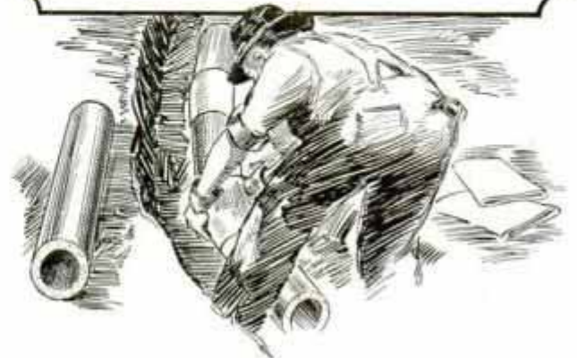
Time and Labor Saved in Laying Temporary Sewer by Joining the Tile with Sections of Inner Tubes
