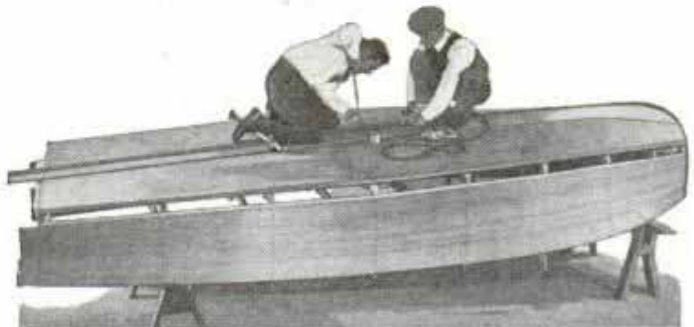
Planking "Roamer"—Popular Mechanics' Outboard Cruiser (765 to 770)
