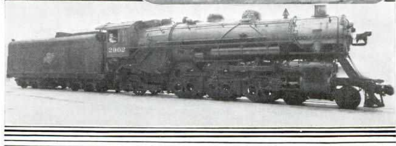
Oil-Burning Locomotive Which Covers Schedule of 400 Miles in 400 Minutes; Note Virtually Solid Drive Wheels; Above, the Racing Iron Horse Traveling at More Than Mile a Minute
