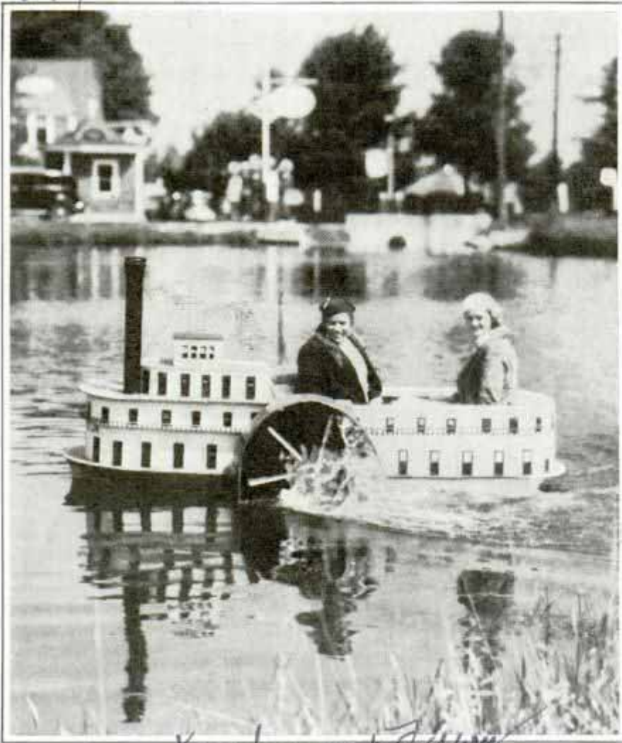
Two-Passenger Model of the River Boat, "Robert E. Lee," Which Is Propelled by a One-Horsepower Motor
