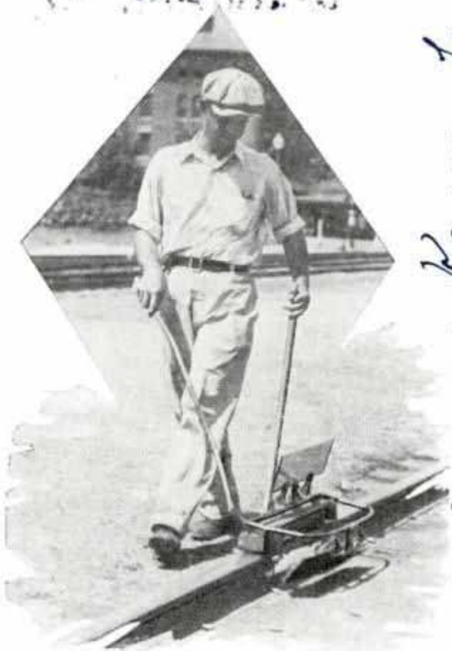
Track Walker Inspecting Rails with the Aid of Small Instrument Containing Two Mirrors
