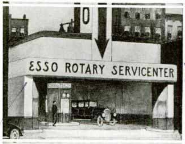
Turntable for the Car Speeds Up Servicing
