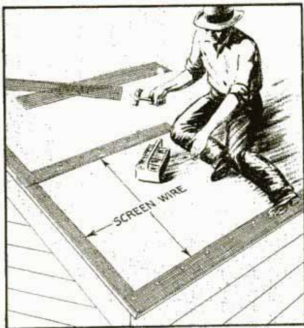
Strips of Screen Wire Folded over Edges of Roll Roofing Prevent Wind from Tearing It Loose
