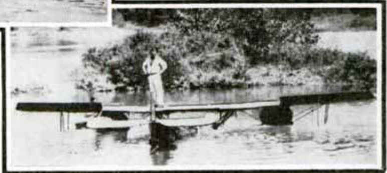
Left, Bags under Wing Beginning to Fill with Gas; Right, How System Works; Bottom, Bags Supporting Plane and Pilot
