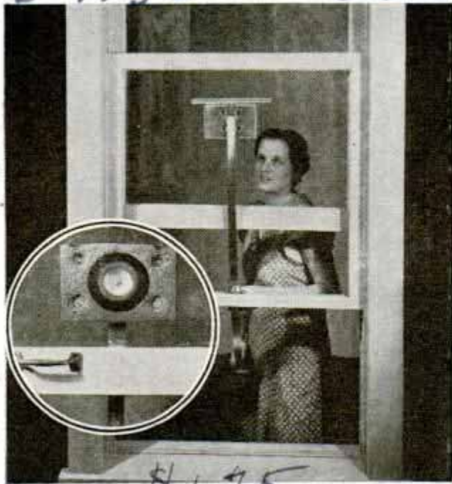
Cleaning Outside of Window From Inside of Room, and Washer Which Makes It Possible
