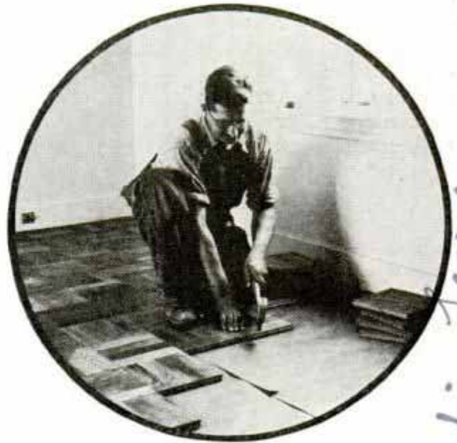
Laying Tongued-and-Grooved Patterned Hardwood-Floor Blocks Finished at the Factory
