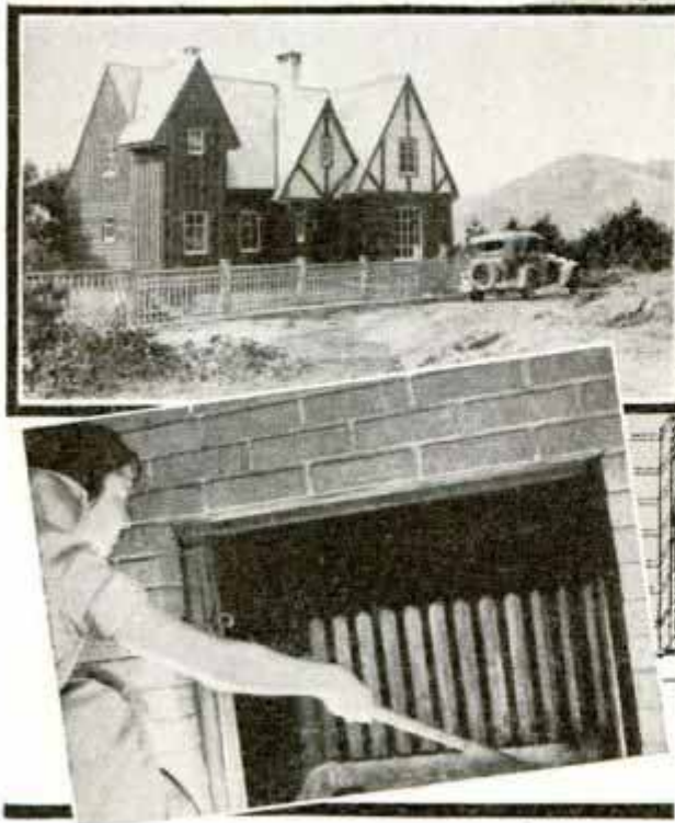
Top, Home Heated by Fireplace Plant; Bottom, Close-Up of Coils; Right, Drawing of the Plant as Installed in One Home; Note Simplicity of Connections to Existing Hot-Water System
