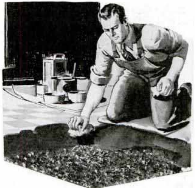
Appearance of Worn Linoleum Can Be Improved Greatly by Stippling It with Enamel
