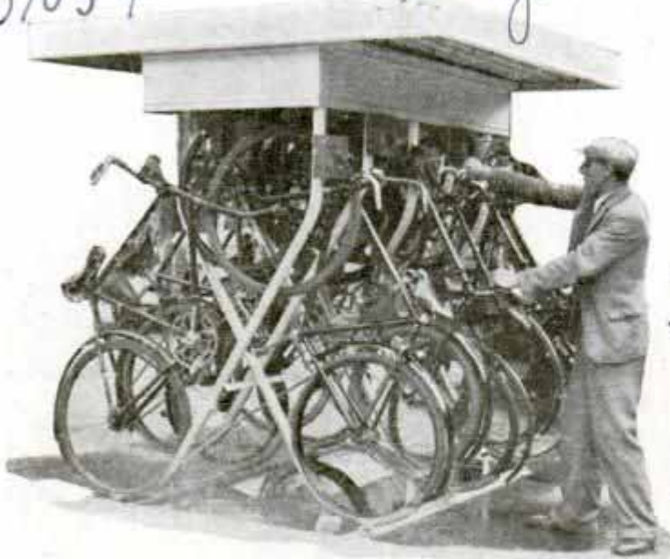
Covered Rack for the Angle Parking of Bicycles; Such Racks Are Widely Used in Berlin
