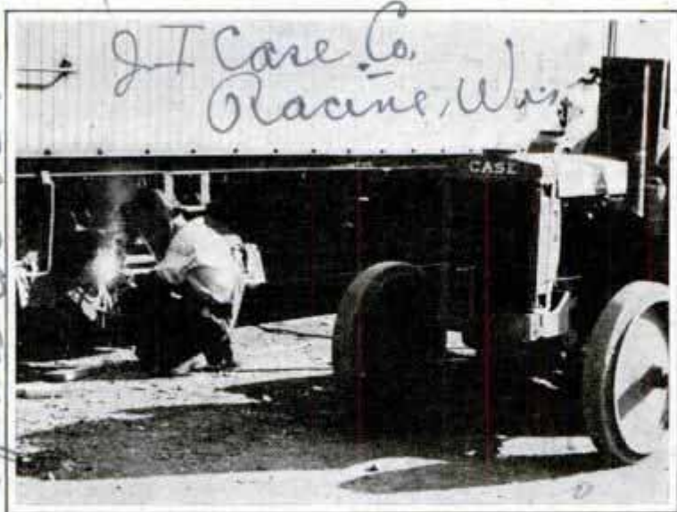
Portable Welding Outfit Mounted on Tractor and Used in Making Electrical Welds in Railroad Yards
