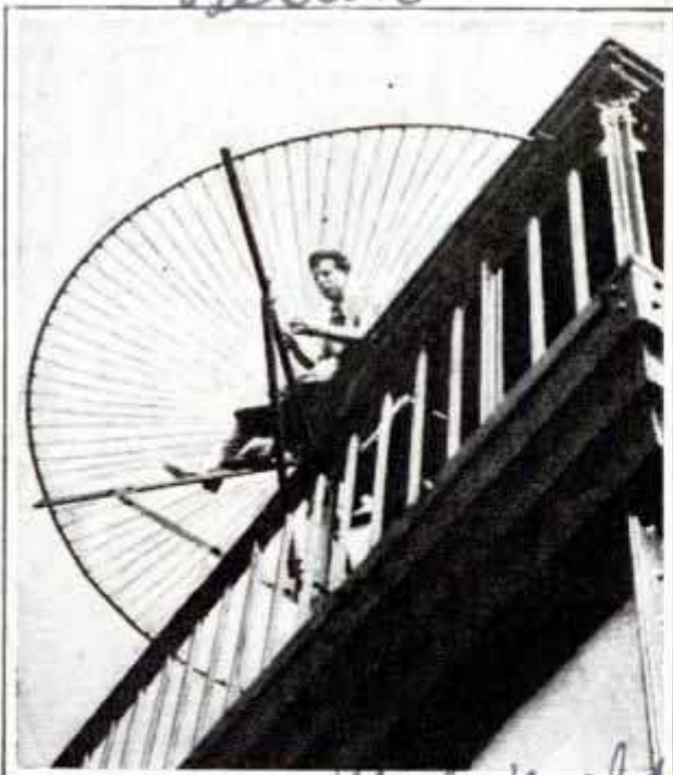
This Wire "Wheel" Is a Television Aerial Used in Germany in Transmitting Pictures
