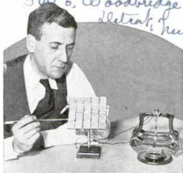
Model Sunlight Motor Actually Produces Electricity; Note Sensitive Plates at Left
