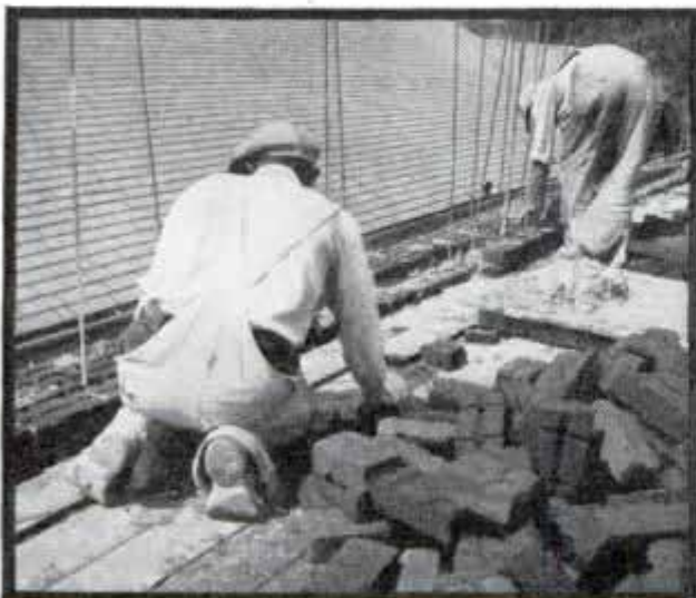
Rods Tie Bricks Together in Wall
