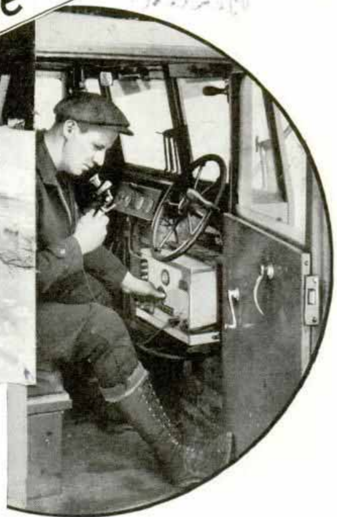
Radio Helps Keep Mountain Roads in the Cascades Clear of Snow by Forming a Means of Communication between Snow Camps and Trucks; over the Short-Wave Set Extra Aid Can Be Summoned in Case of a Sudden Blizzard, and Slides, Weather Conditions and Breakdowns Are Reported; Above, Snowplow, Showing Radio Antenna; Right, Radio Set in Truck
