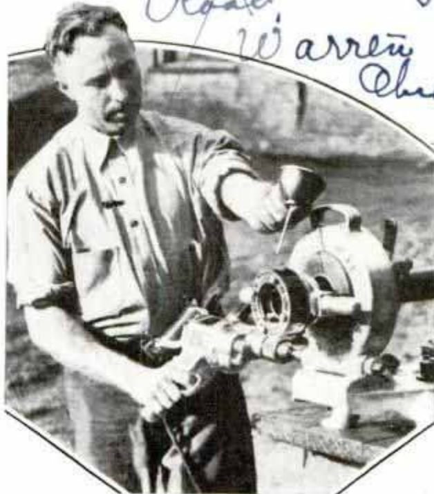
Lightweight Portable Pipe Threader Which Can Be Operated by Pneumatic or Electric Drill
