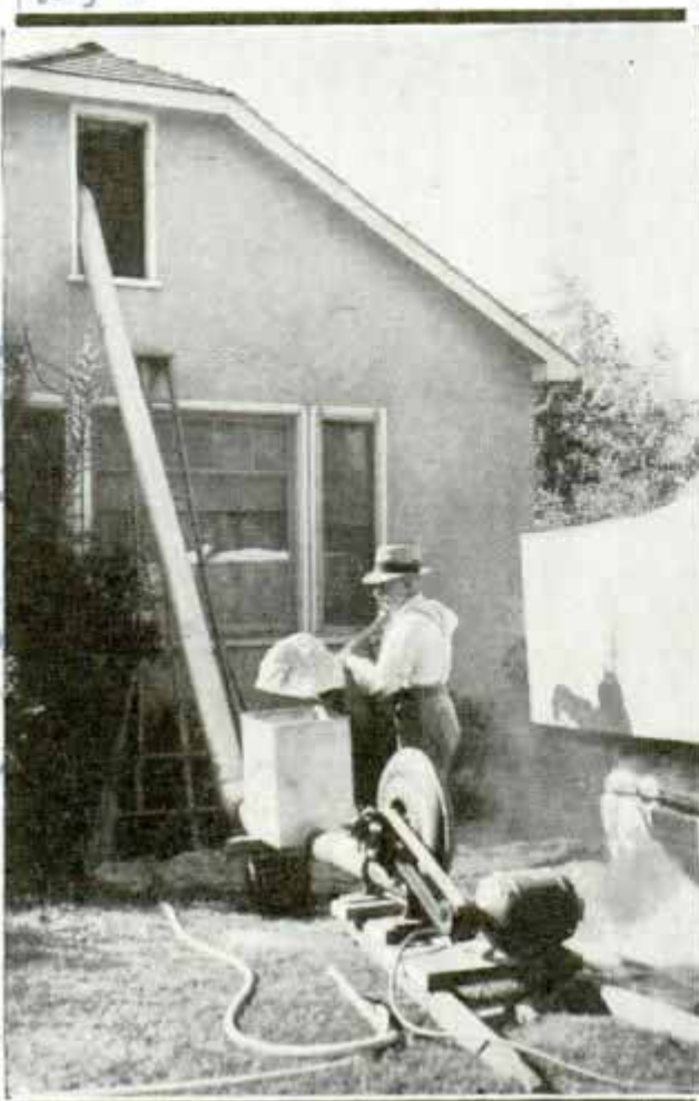
Blowing Rice-Hull Ashes into the Attic of a Building to Form Layer of Fireproof Insulation
