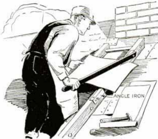
Sheet Metal Cut as Needed on Roof with Shears Screwed to Side of Ladder
