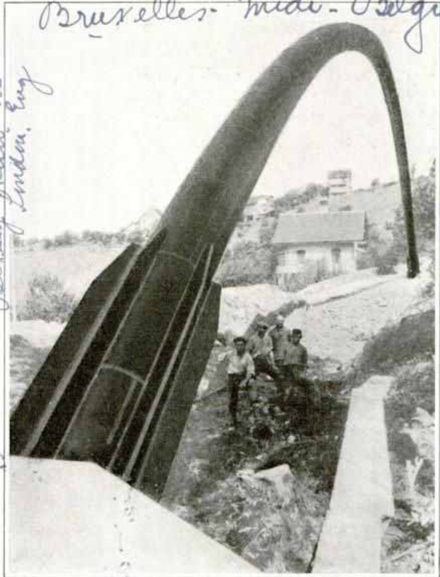
Showing Great Arched Pipe That Carries Water over Shaky Soil in Switzerland; Compare Its Height to That of Men in Photo
