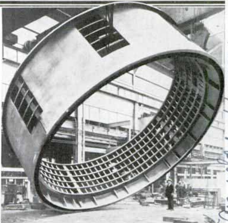
Top, Niagara Falls Lighted by Power It Generates; Bottom, Frame for Waterwheel Generator at Boulder Dam
