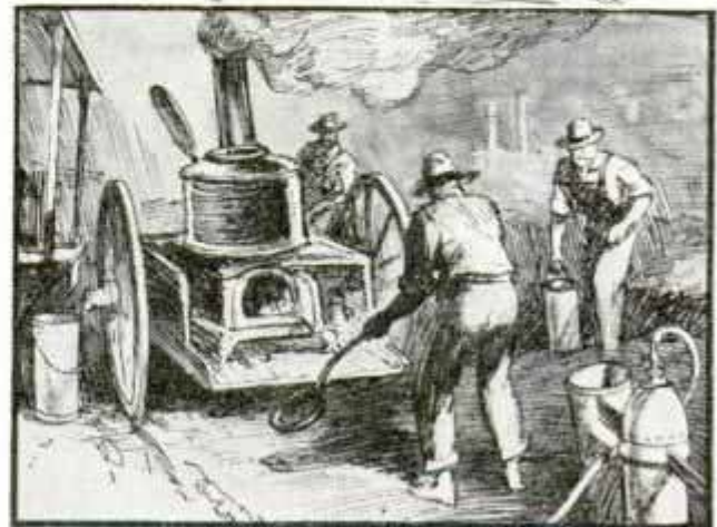
Drawings from Harper's Weekly, 1882, of Electric Wire Tubes Being Laid in New York
