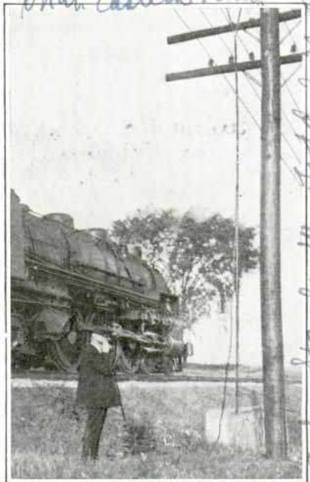
Using Collapsible Pole and Telephone to Establish Connection with Railroad Division Offices
