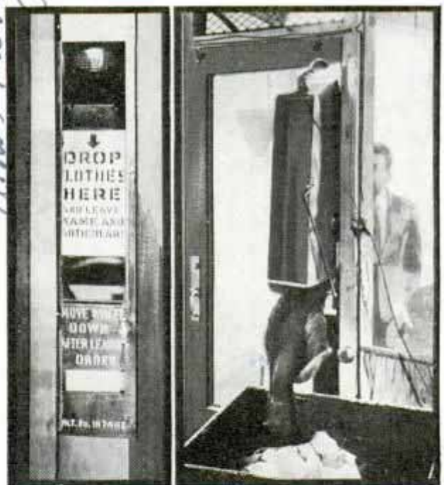
Left, Outside of Parcel Chute; Right, Inside View, Showing Receiver for Parcels
