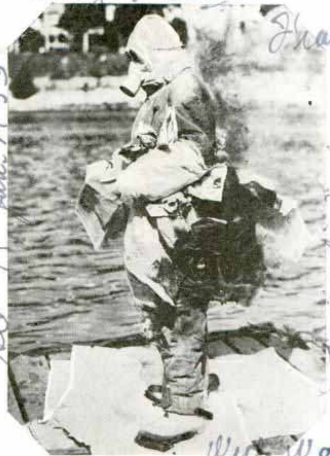
Testing Fireproof Qualities of Suit of Flyers Which Will also Keep Wearer Afloat in Water
