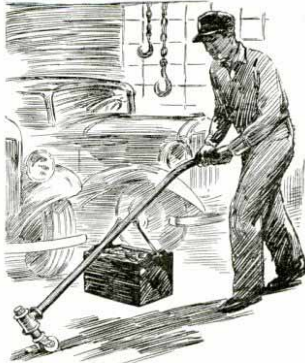
Simple Truck Improvised from Pipe and Fittings for Carrying Storage Batteries in Garage
