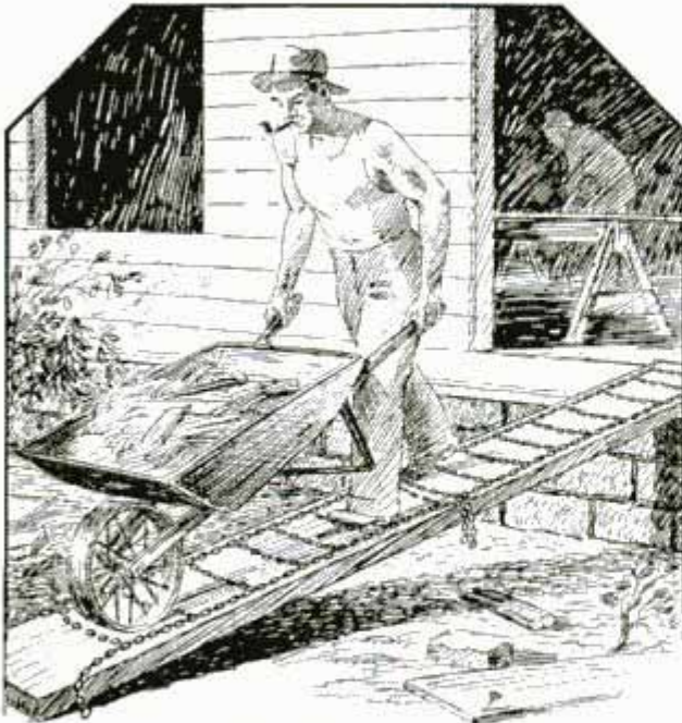
Skid Chains Nailed to Gangplank Provide Footing for Workmen Pushing Wheelbarrows
