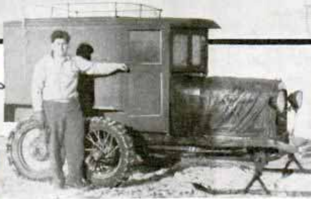
Dog Teams in the Far North Replaced with Cars Having Runners and Tractor-Type Wheels
