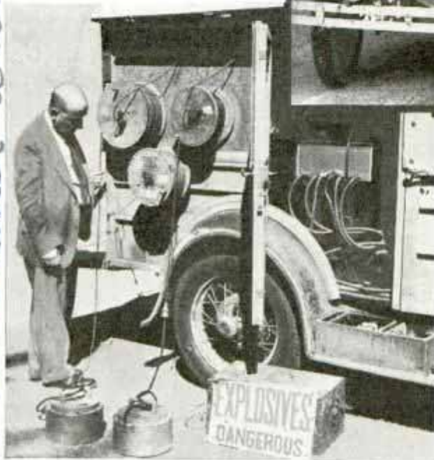
Wide World Truck and Recording Instruments Used to Reveal Underground Secrets with Aid of Explosives
