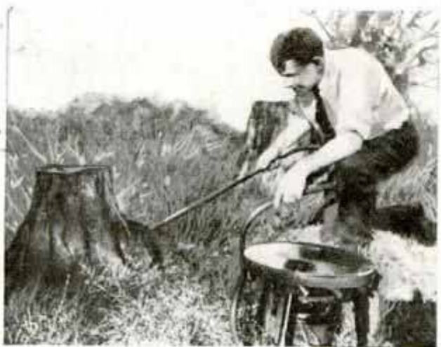
Using a Forced-Draft Burner to Destroy Stumps
