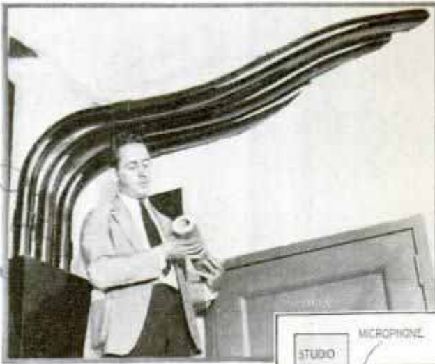
Pipes Carrying Sound to Echo Vault, a Diagram of Plan and Microphone in One of Vaults
