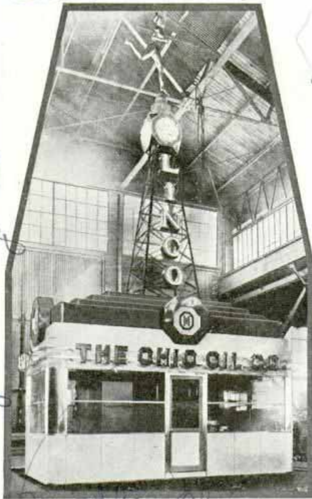
Portable Gasoline Filling Station Which Can Be Moved by Truck or Rail to a New Location
