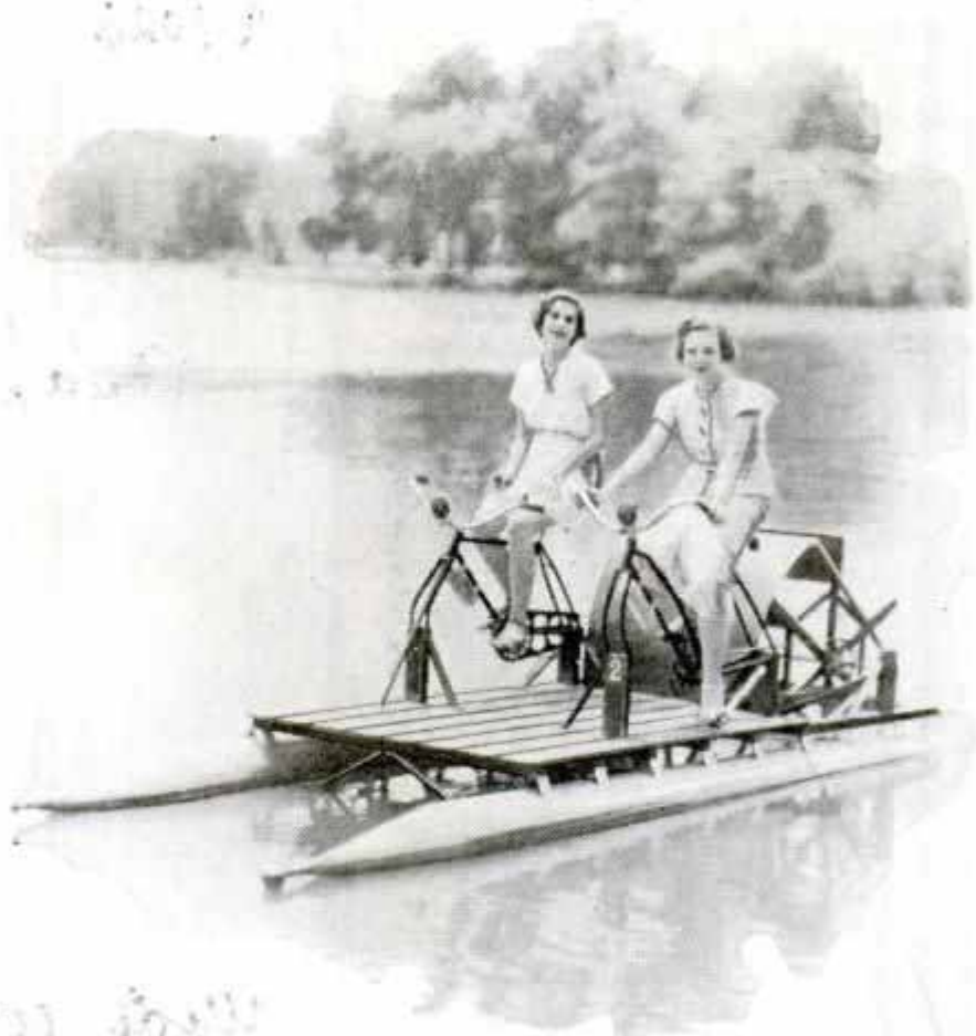
Pontoon Boat Operated by Pedals Which Turn Paddle Wheel at the Rear
