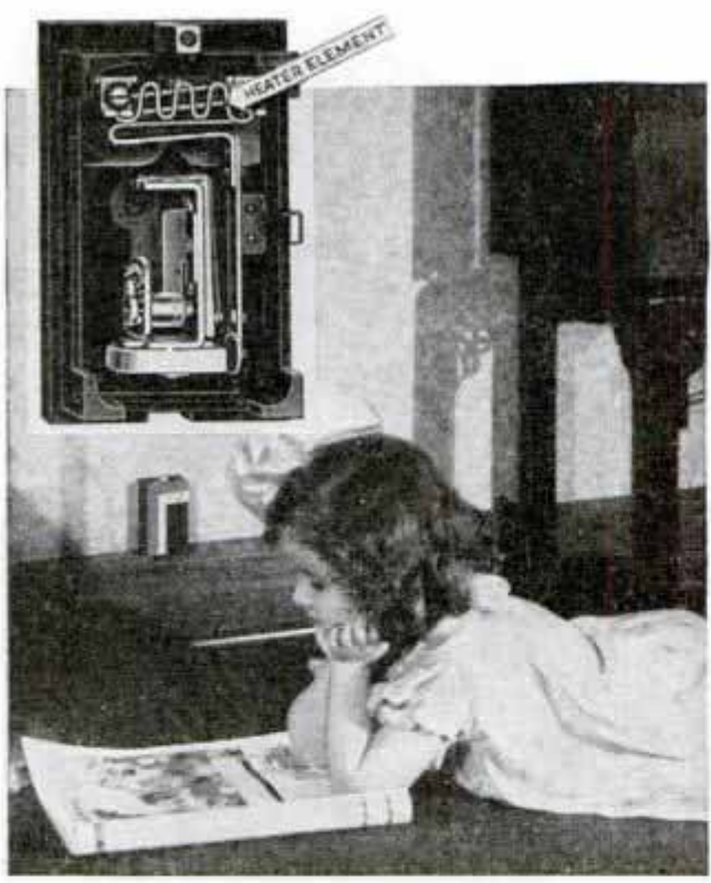
Switch Installed Just above Baseboard; Inset at Top, Closeup of Thermostatic Switch
