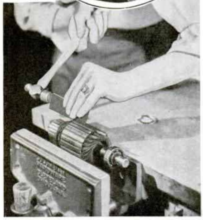
Loosening and driving out the coil wedges
