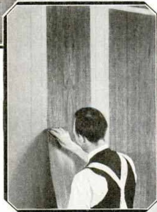
Top, Wooden Wallpaper with Cloth Backing; Center, Applying Wooden Wallpaper; Bottom, Foreign and Domestic Woods Used in Wooden Wallpaper and Plywood
