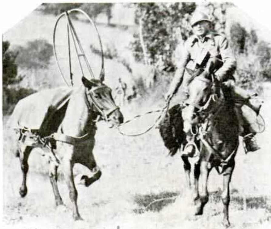
How Field Radio Equipment Is Transported by the Italian Cavalry During War Games; Note Position of Aerial on the Horse's Back
