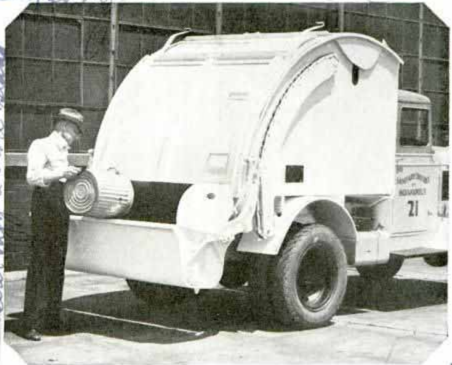
Emptying Garbage Can into Loading Receptacle; the Larger Garbage Container Is Water and Air Tight, Preventing Escape of Odors
