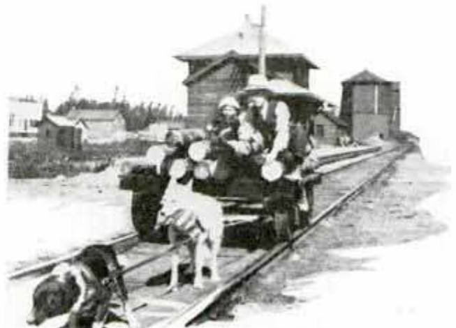
Dog-Power Railroad Car Is Used to Haul Building Materials to Places Isolated from Highways
