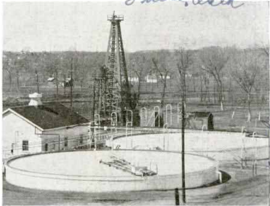
Well Which Pumps Natural Brine to Surface Where It Is Converted into High-Grade Salt and Other Useful Products
