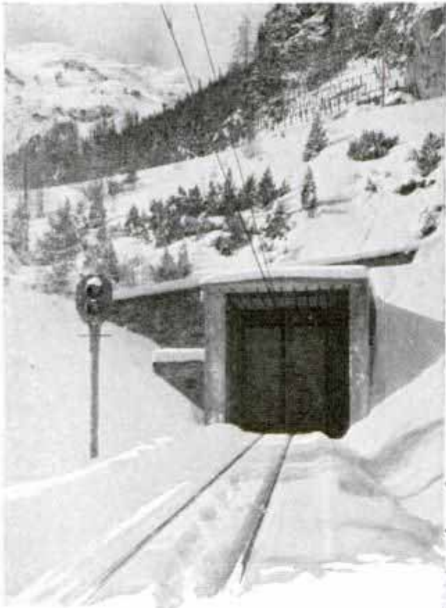
Doors at Entrance to a Railway Tunnel in Swiss Alps Which Open Automatically as Train Approaches
