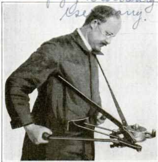
Portable Stitcher for Closing Bags or Cartons; It Converts Wire into Clips as a Reel Unwinds
