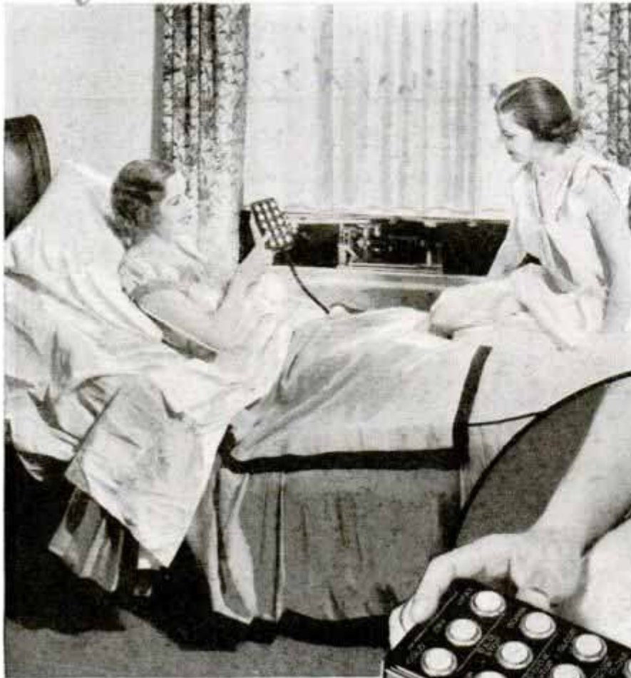
Keyboard Controls for Windows, Doors, Bed and Air-Conditioning Plant
