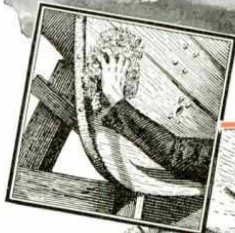
After a thorough rub-down with steel wool the bottom of the hull is painted
