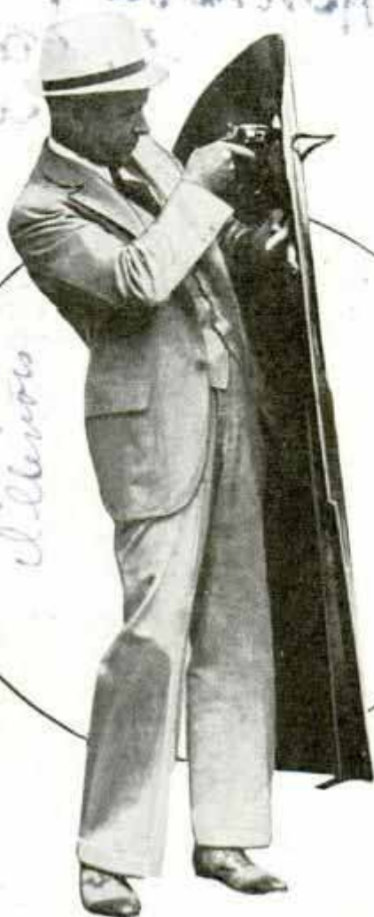
Bulletproof Shield for Use of Police Officers; It Can Be Handled Easily by One Man
